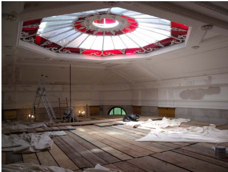
Montefiore Synagogue, Ramsgate, during repairs.
