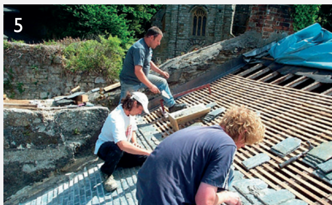
Trainees using traditional Cornish slate to repair a roof in Tuckingmill, Cornwall. © Cornwall Council Historic Environment Service.
