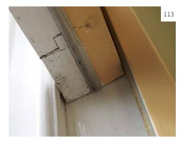
Compression strips are available in a range of materials. The simplest to install are self-adhesive strips of rubber (EDPM). These are available in a variety of profiles and thicknesses to cater for different gap widths. Foam strips are cheaper still but have a short life. Silicone and rubber 'O' tubes are available in a variety of diameters. Some attach to the frame using an adhesive others come on a carrier strip that is either attached to or cut into the frame.
