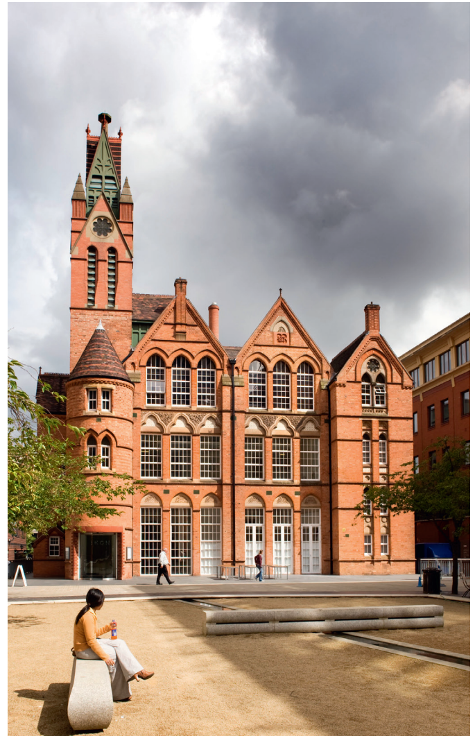
Schools project. Ikon Gallery, Oozells Square, Birmingham, West Midlands. General view of front elevation. © Historic England
