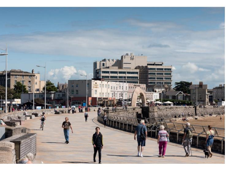
Figure 93 The new flood and tidal defence scheme included the creation of an additional splash wall on the road side of the widened promenade and stepped sea defences to protect the base of the sea wall. [DP218045]
