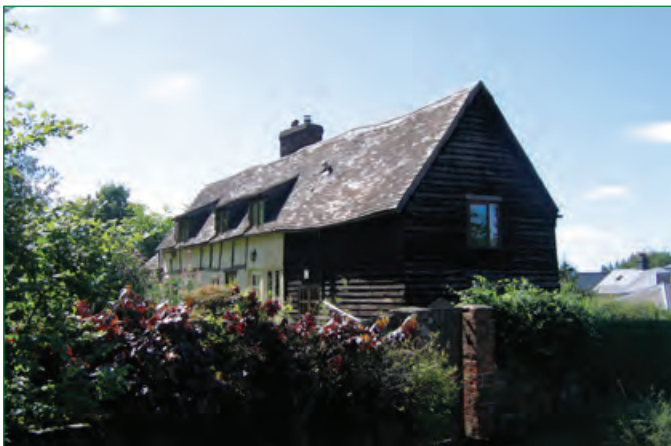
A rare surviving example, to the west of the area, of a timber-framed linear farmstead of the 17th century or earlier where the house and working buildings are attached and in-line.
