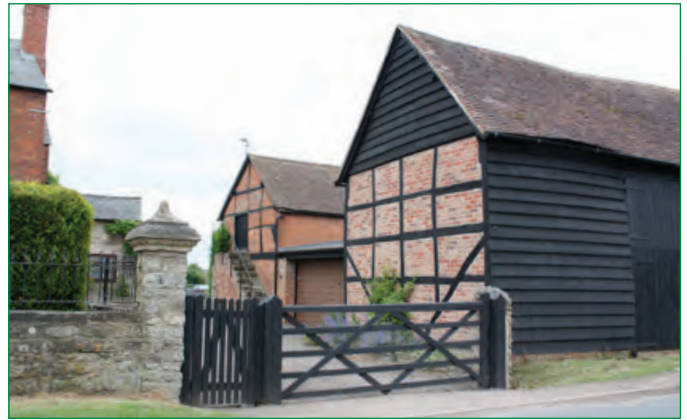
Some substantial timber-framed barns of the late 16th and 17th centuries have survived, with the distinctive square panel timber framing typical of the western English carpentry tradition.
