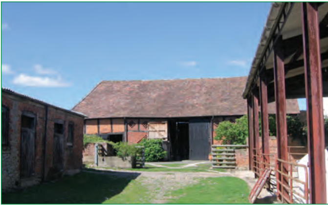
Some substantial timber-framed barns of the late 16th and 17th centuries have survived, with the distinctive square panel timber framing typical of the western English carpentry tradition.
