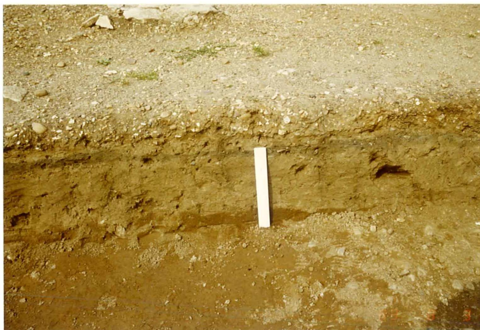
B. SITE 2: SECOND ROAD SECTION TRENCH PROFILE BELOW CENTRE OF ROAD.
