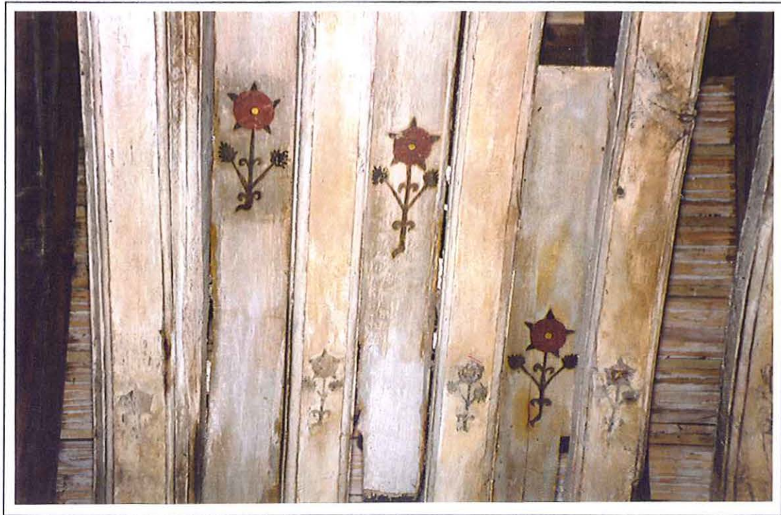
Detail, painted decoration on ceiling timbers
