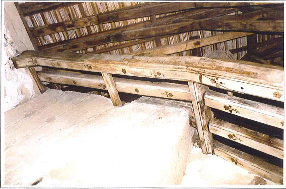
Prior's Lodgings, ceiling
