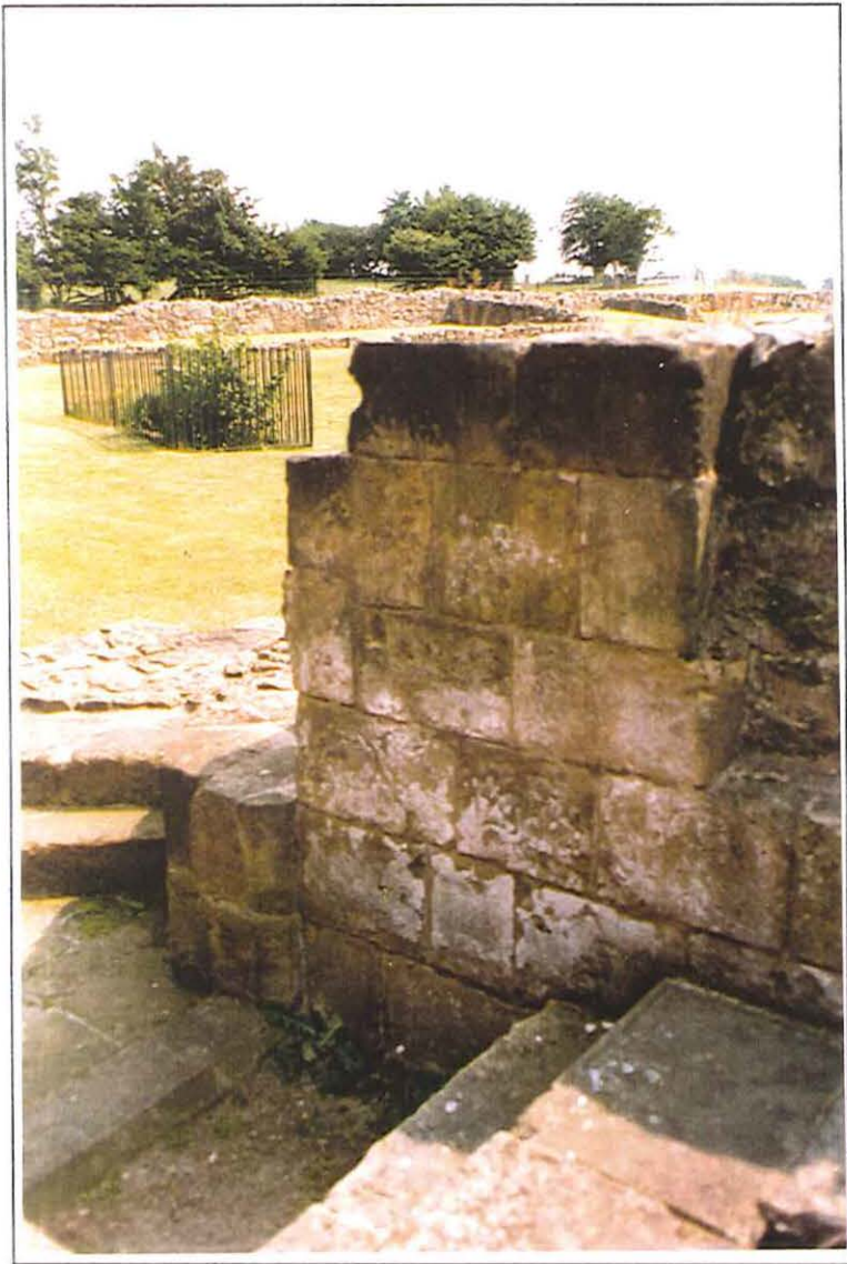
East end, south chapel, southeast corner
