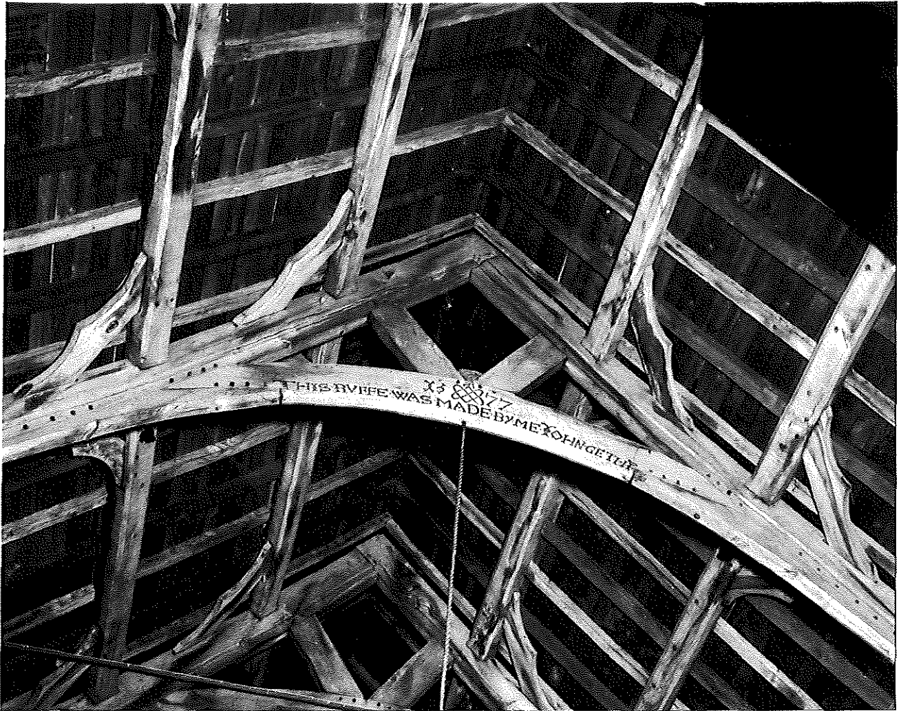
Figure 5 The Church of St. Mary the Virgin, Bromfield Shropshire. Detail of the collar in the nave roof dated by inscription to AD 1577 (© Crown Copyright)
