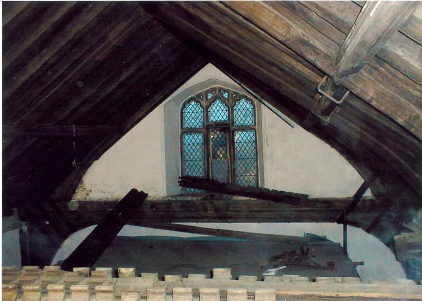
Figure 2: View of the nave roof showing moulded purlins and principal rafter and embattled tie beam (photo A F Knight Builders of Debenham)
