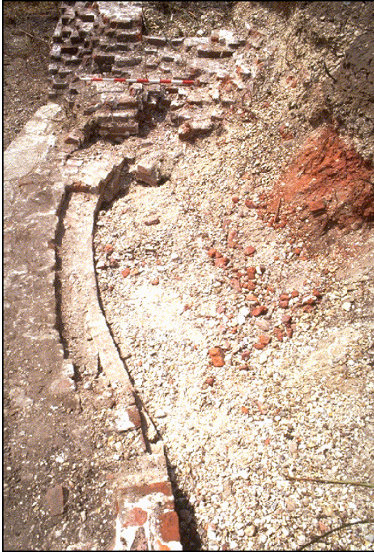
Figure 3 Photograph showing the breach in the counterscarp wall and the Portland limestone foundations (formerly a straight wall line) 2m scale
