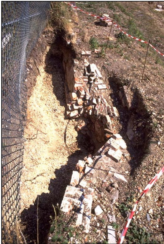
Figure 4 Photograph showing the bomb damage to the parapet wall of the covered way
