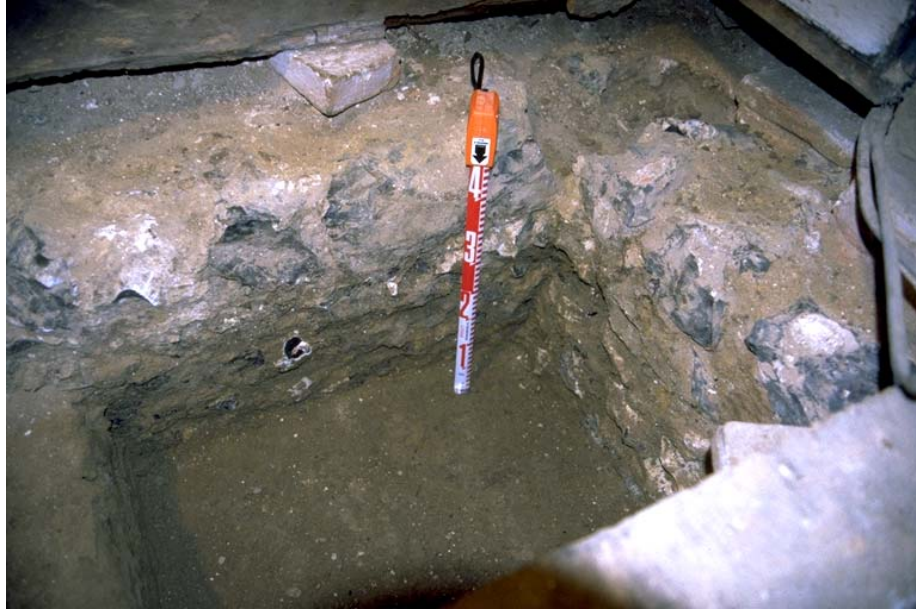
Figure 14: Trench P2 Junction between the north wall of the crosswing and the footings of the jettied western front of the house - 0.4m scale
