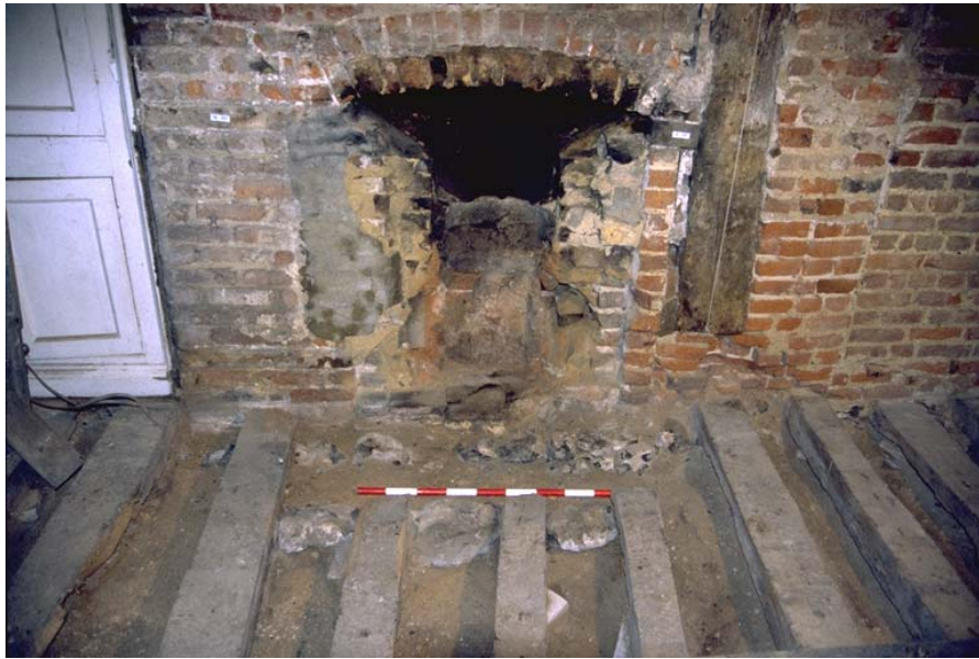
Figure 11: Southern face of western chimney stack showing shortened joists and flints from hearth -1m scale
