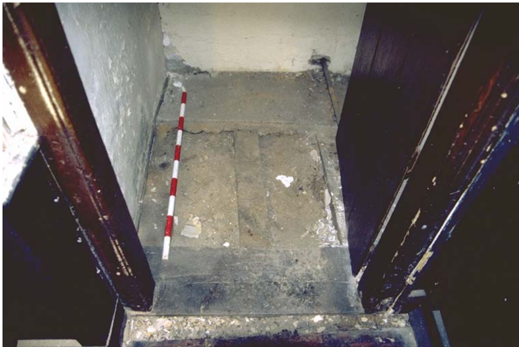
Figure 6: The base of the cupboard following removal of floorboards - 1m scale
