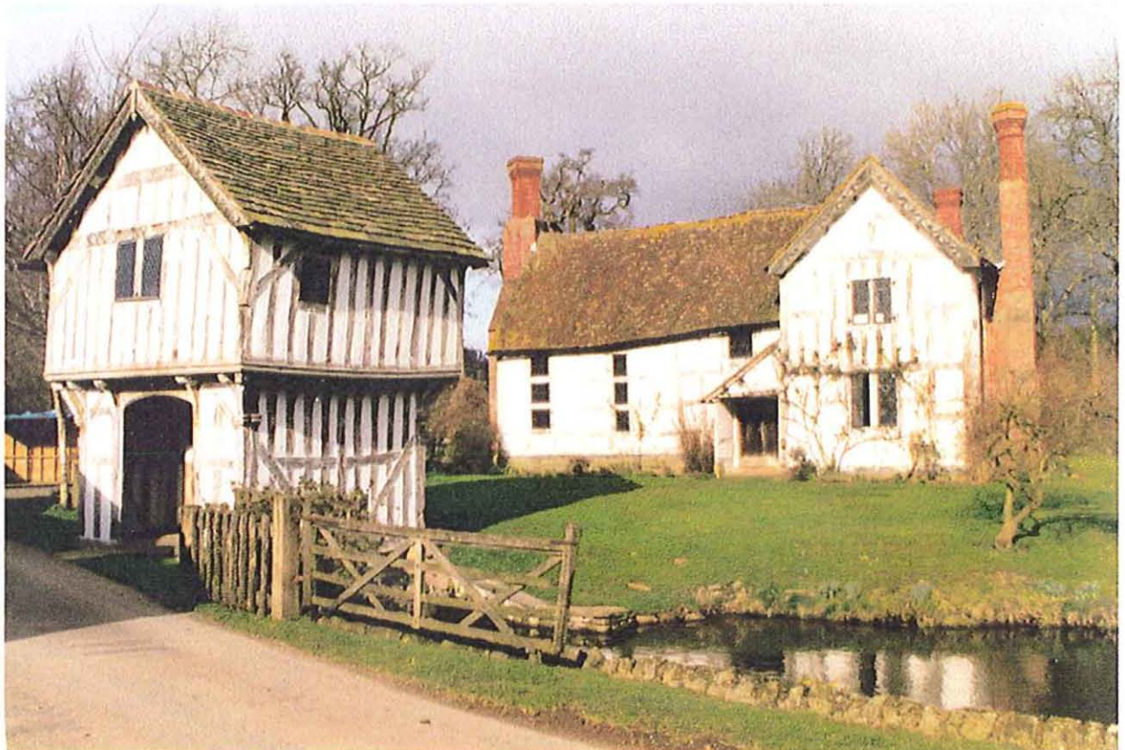
Figure 2 Lower Brockhampton Gatehouse (left foreground) and moat with Lower Brockhampton House in the background. View towards the north-west (the author)
