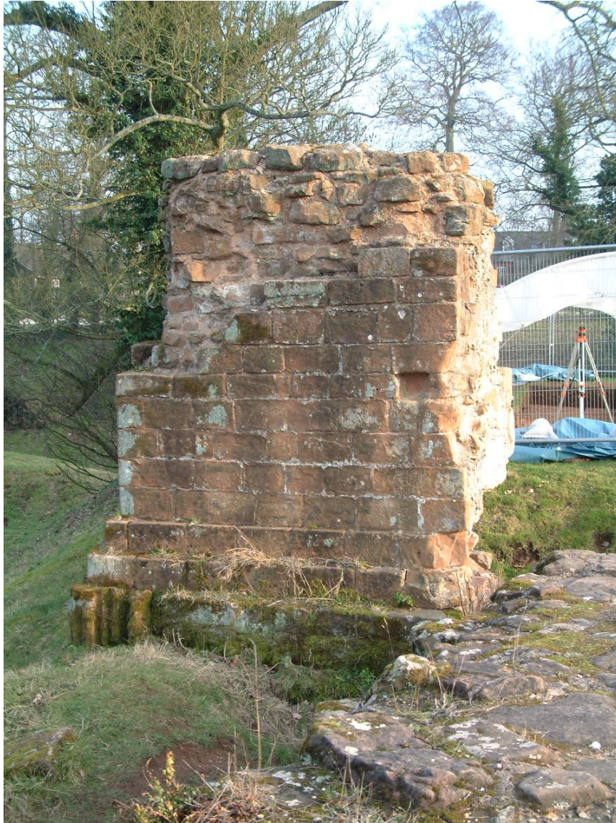
Fig 8. Exterior of Gallery Tower wall showing steps in foundation, as well as fluted block.
