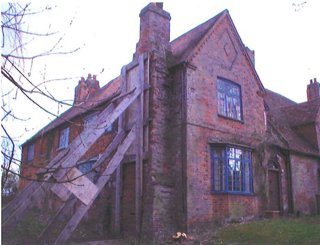
Figure 4 The north-east corner of Wymondleybury (photograph C Locatelli)
