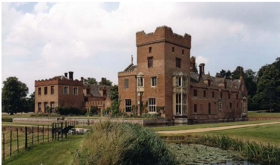
Fig 12. The leat supplying Oxburgh's moat. (NMR BB032385)
