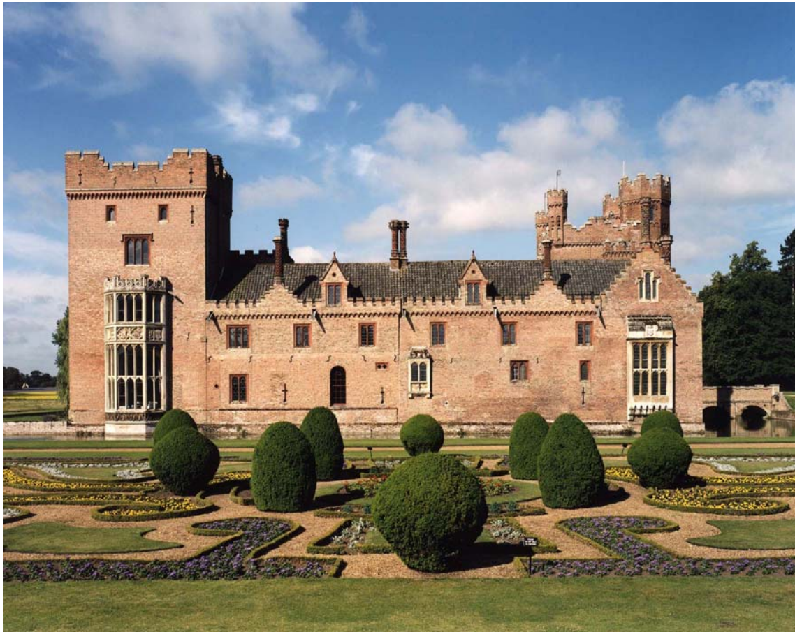
Fig 124. The moatside elevation of the east range, with the French garden in the foreground. (NMR BB32387)
