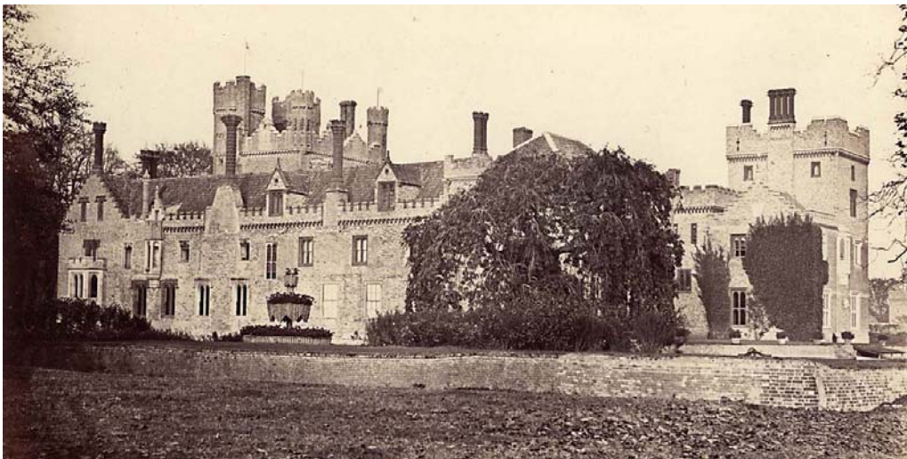
Fig 9. 'Oxburgh Castle' from the south-west, taken before the construction of the south range and published in Norfolk Photographically Illustrated in 1865. Two surviving sash windows show on the ground floor of the west elevation. (NMR)
