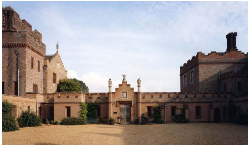
Fig 117. The courtyard elevation of the south range. (NMR BB032410)
