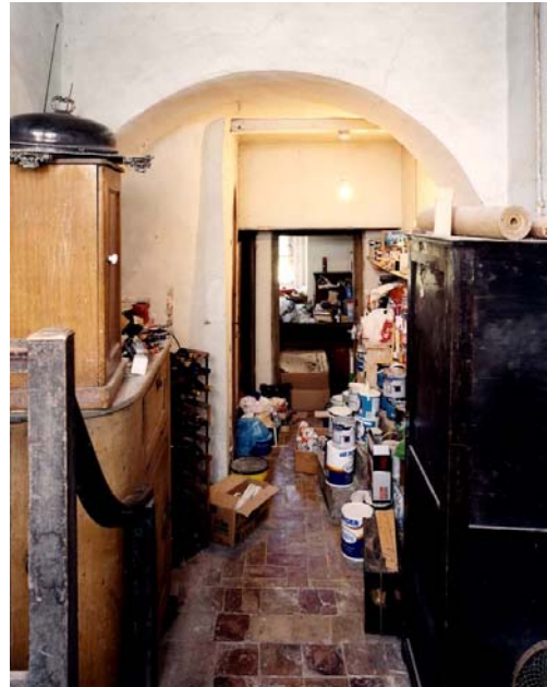
Fig 126. The former Boot Room where some Second World War graffiti survives. The arch carries a flying flue. (NMR BB032447)
