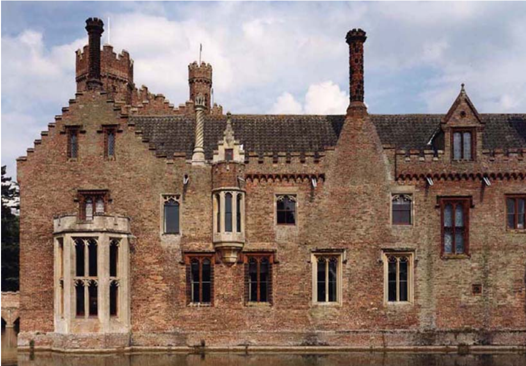
Fig 51. The northern half of the west range: the moatside (west) elevation. All the windows date from the 19th century in their present form. Replaced brickwork just to the right of the bay window is the result of patching consequent upon the discovery of garderobes at the junction of the two ranges. (NMR BB032405)
