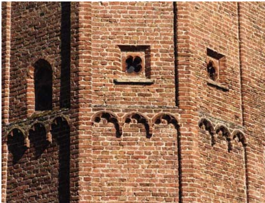
Fig 22. Arcaded panels and quatrefoil windows lighting the gatehouse stair turret. (NMR AA026775)
