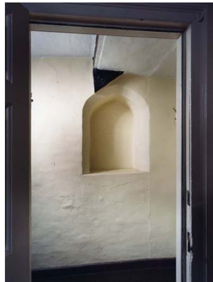
Fig 41 (left). The garderobe opening off the first floor of the north range. (NMR BB032443)
