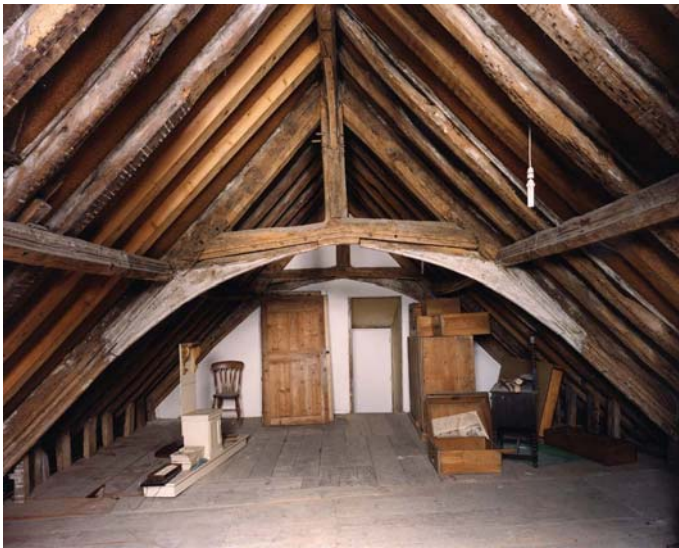
Fig 49. The roof over the northern half of the east range, from the south. The attic floor is a later insertion. (NMR BB032463)
