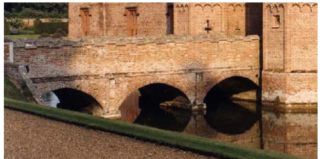
Fig 62. The bridge traditionally attributed to Lord Burlington, from the north-west. (NMR BB032390)
