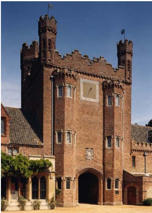
Fig 27. General view of courtyard elevation. (NMR BB032406)
