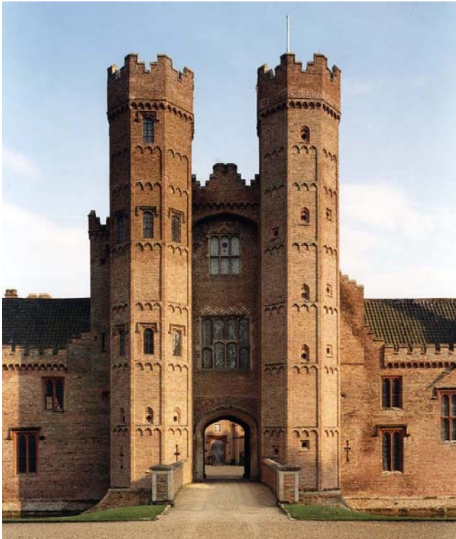
Fig 20. The north elevation of the gatehouse. The turret rising against the east (left) face of the gatehouse houses the garderobes. Compare Fig 21. (NMR BB032391)
