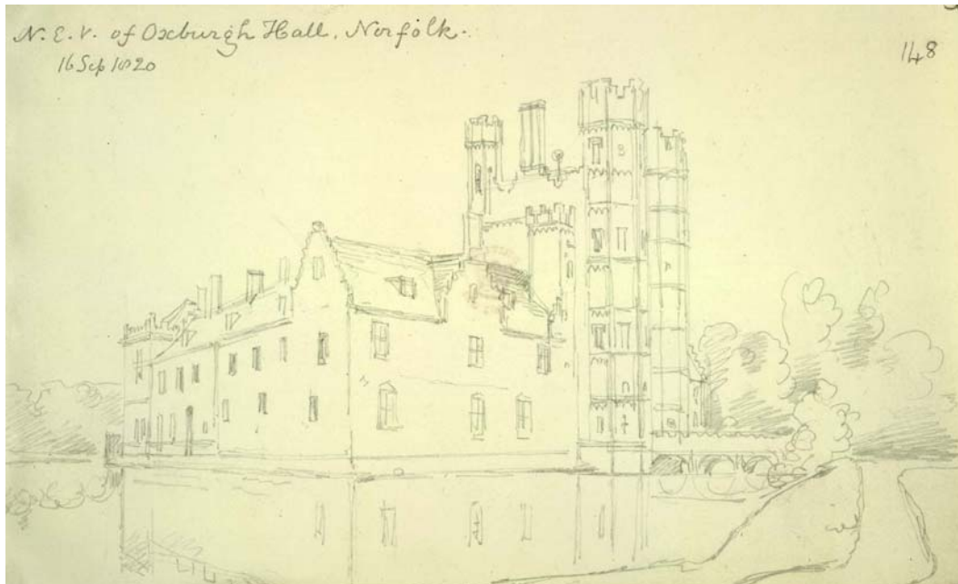
Fig 48. Buckler's 1820 view, showing the fenestration of the north and east ranges before the 19th-century alterations. Buckler also shows the single brick diaper at the left end of the north range. (British Library)
