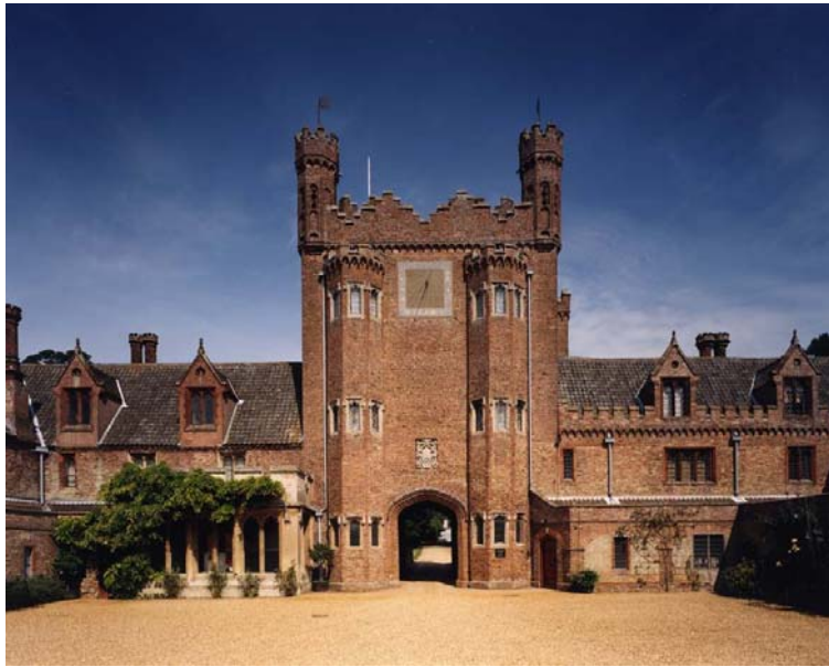
Fig 94. The courtyard elevation of the north range and gatehouse, showing the impact of Buckler's dormer windows. (NMR BB032407)
