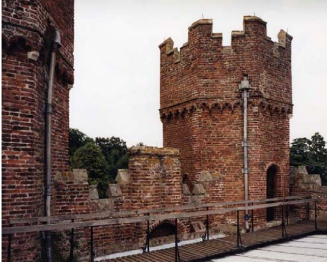
Fig 18. Dummy chimney stacks supported on an arch above the machicoulis on the north front of the gatehouse. The nearer turret contains the stair; the turret beyond housed the dovecote. (NMR AA026768)
