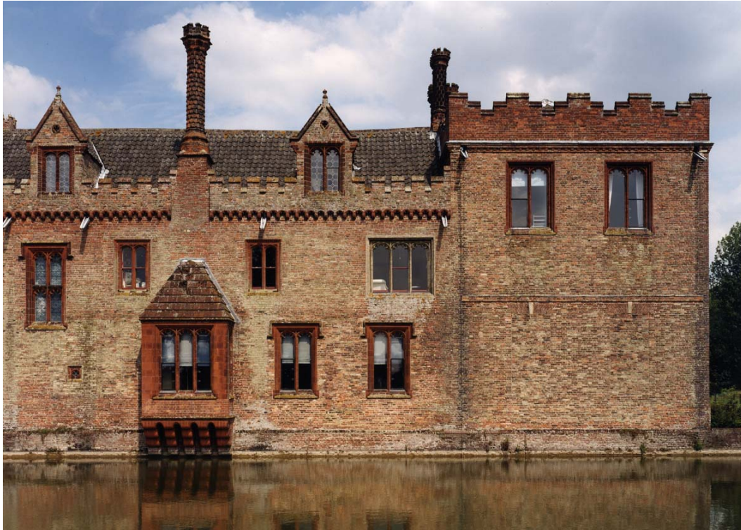
Fig 52. The southern half of the west range: the moatside (west) elevation. In the 1770s the range was slightly truncated when Tasker's pavilion (right) replaced the former Kitchen and service rooms. Part of an original window head is visible above the window lighting the west stair (left). (NMR BB032404)
