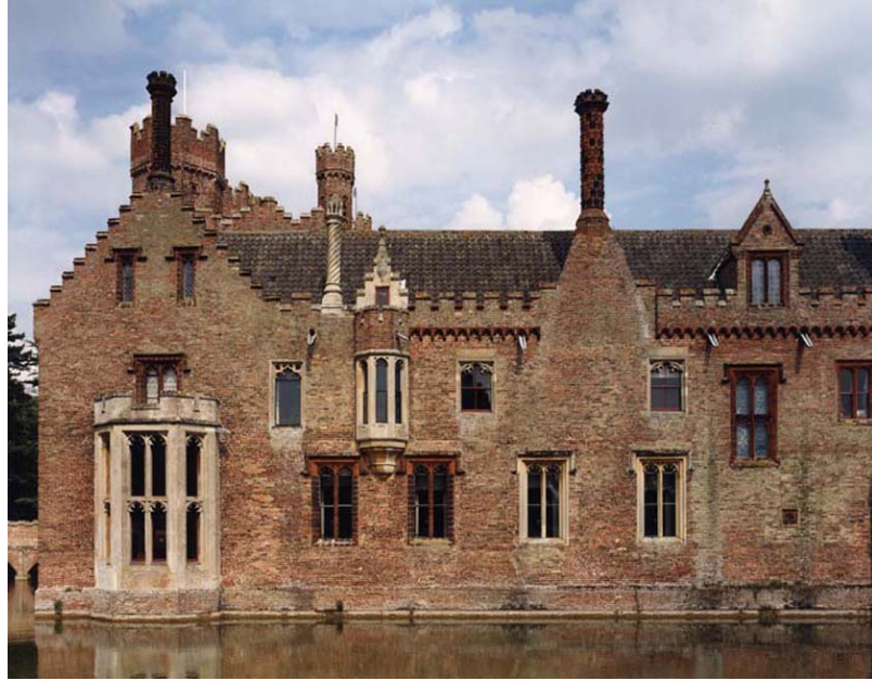
Fig 93. The moatside elevation of the northern half of the west range, showing the diversity of window types employed by Buckler. (NMR BB032405)
