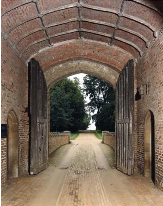
Fig 26. The carriageway passing through the gatehouse, with the 18th-century bridge beyond. The doorways to either side are 19th-century replacements. (NMR BB032414)
