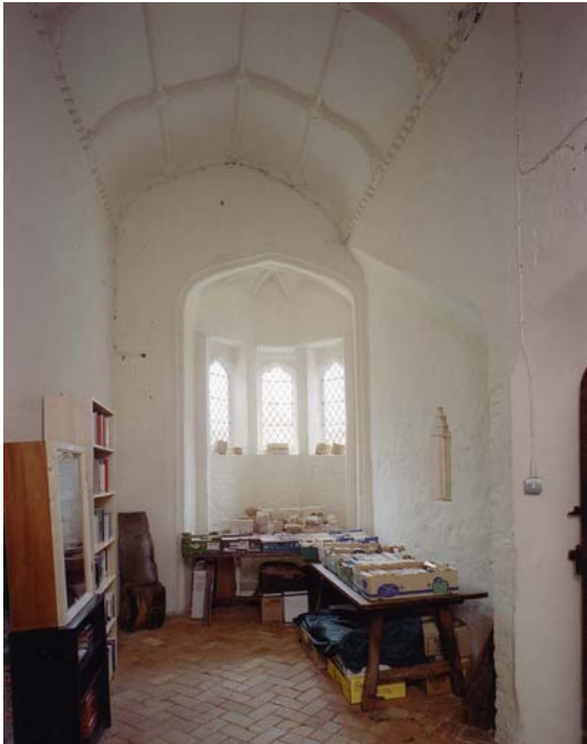
Fig 29. Interior view of Porter's Lodge from the north, showing the asymmetrical positioning of the window. (NMR BB032420)
