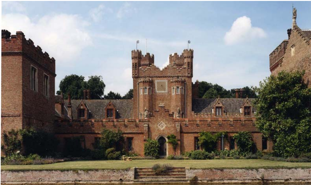
Fig 119. The south elevation of the south range, viewed across the moat. By setting the range back an area of private garden was left inside the moat. (NMR BB032402)
