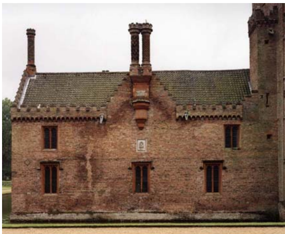
Fig 95. The moatside elevation of the north range east of the gatehouse. (NMR BB032396)
