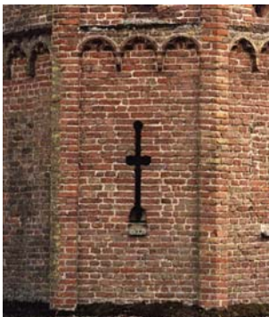
Fig 19. Gun-port in the lowest stage of the NE gatehouse turret. (NMR AA026773)
