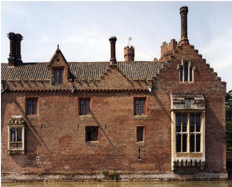
Fig 47. The northern half of the east range. (NMR BB032397)
