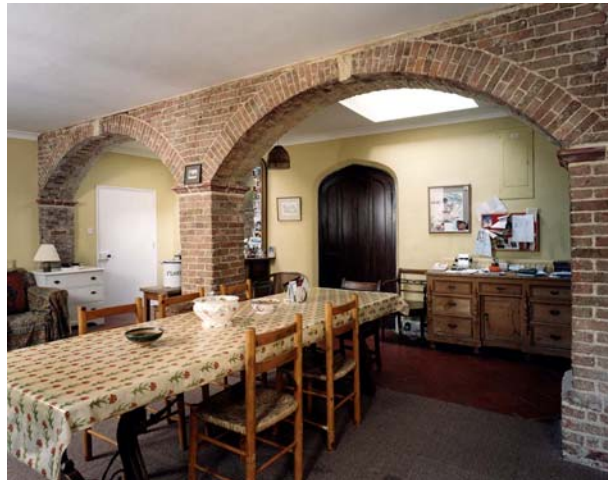
Fig 87. Two bays of the arcade alongside the east range were restored in recent years. View from the south-west. (NMR BB032448)
