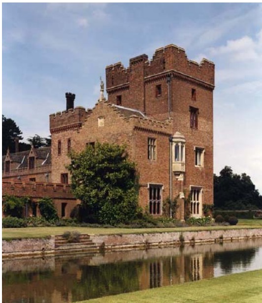
Fig 110. The remodelled south-east pavilion with its tower added in two stages. (NMR BB032401)
