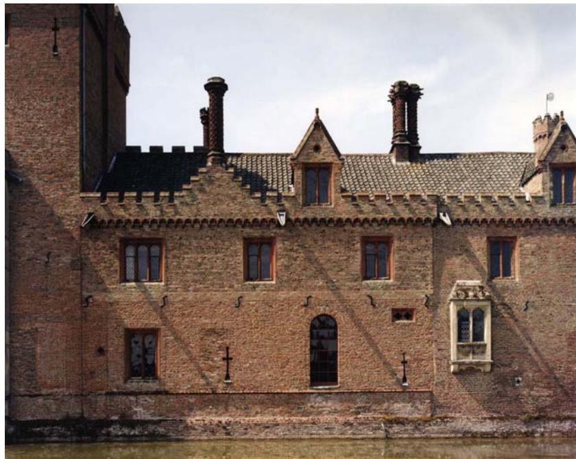
Fig 73. The moatside elevation of the rebuilt portion of the east range. The mullioned windows date from a the 19th-century remodelling. (NMR BB032398)
