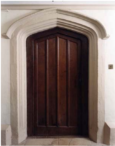
Fig 14. The doorway to the west stair. (NMR BB032484)
