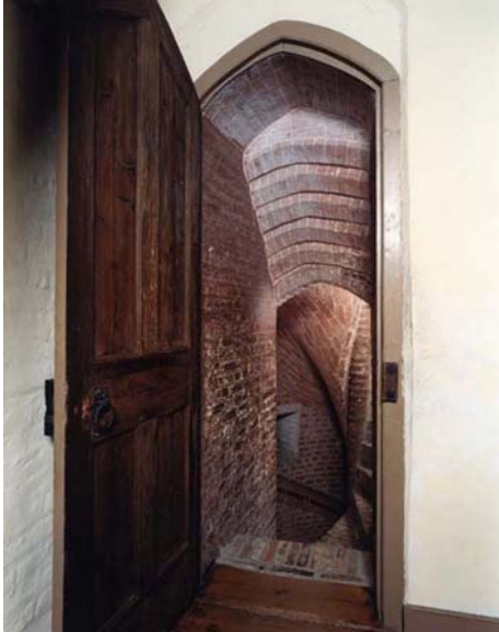
Fig 33. The doorway from the King's Room to the stair. (NMR BB032432)
