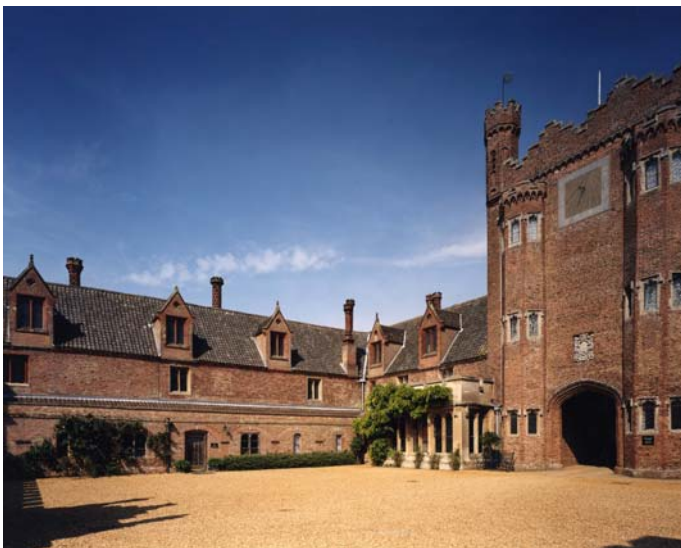
Fig 79. The now-infilled western arm of the arcade (left), together with the north return, largely remodelled to form a bay window. (NMR BB032412)
