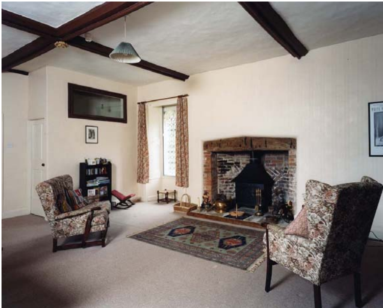
Fig 57. The first-floor room adjoining the gatehouse. The modern boxing and door (far left) conceal the original garderobe entrance. The ceiling dates from the 16th century and later. (NMR BB032444)
