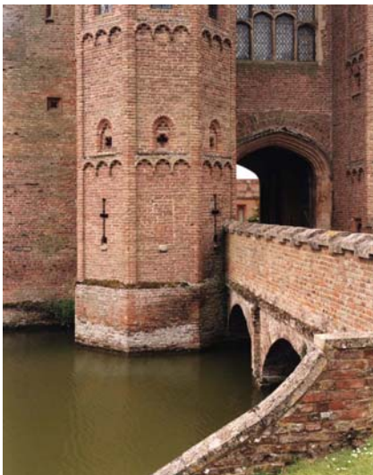
Fig 13. The bridge across the north arm of the moat. (NMR BB032392)
