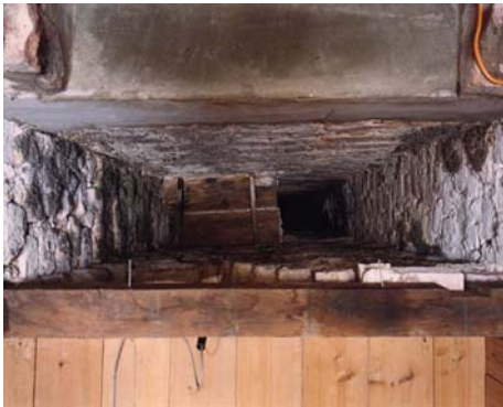
Fig 40. View looking up the garderobe chute. (NMR BB032438)
