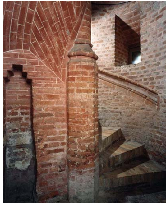
Fig 32. The foot of the turret stair. (NMR BB032423)
