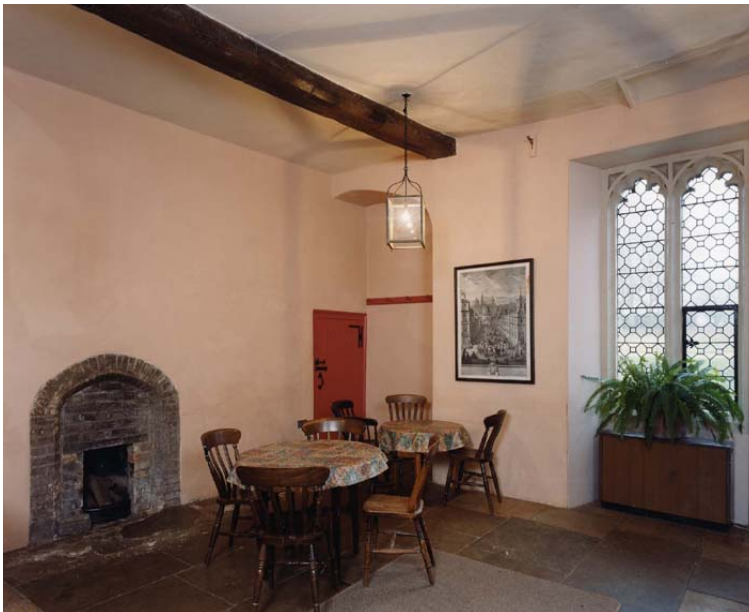
Fig 56. Successively the Laundry (1774) and the Servants' Hall, and now part of the Tea Room, this room must always have performed a service function. The fireplace, though it has an outwardly late 15th-century form, is a reduction of an earlier large fireplace. The recess in the far corner provides access to the base of the gatehouse garderobe chutes. The supports for a first-floor fireplace (served by one of the flues of Buckler's corbelled stack) can be seen top right. (NMR BB032437)
