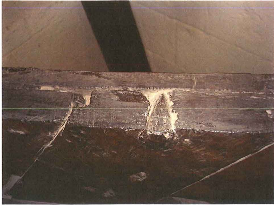
Figure 16: Detail of peg inserted into reused brace ( wa91 ) used in the construction of the Chapter House undercroft door (D Miles)
