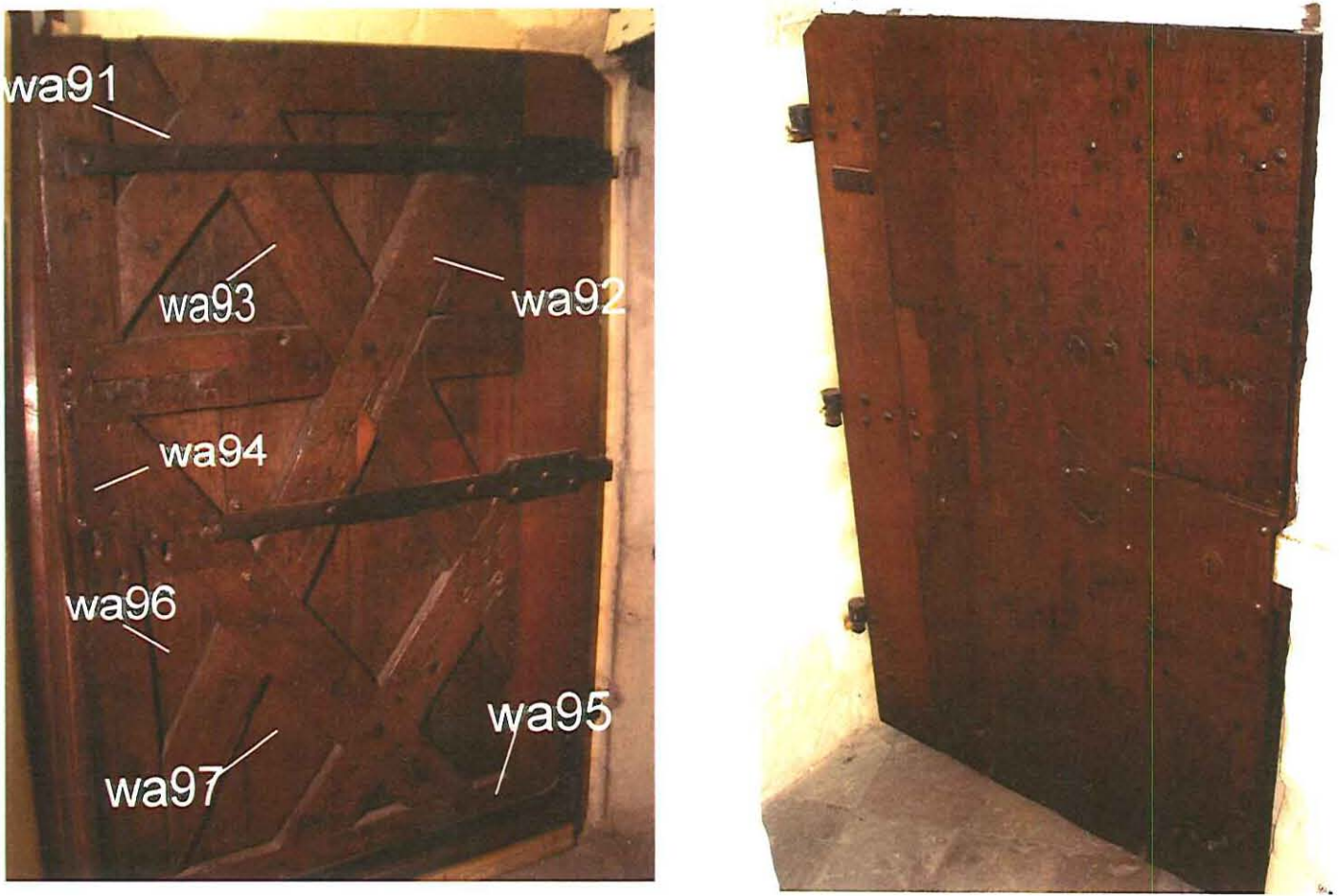
Figure 15: Outer (after W Rodwell) and inner faces of door to Chapter House undercroft showing sample locations
