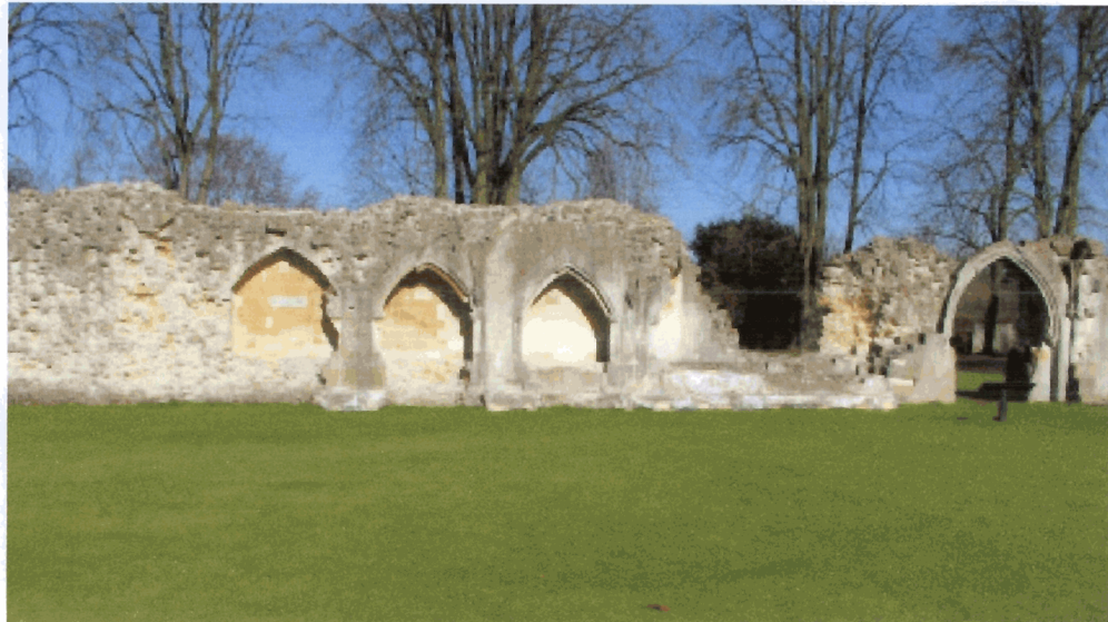
Figure 3. The northern cloister wall.
