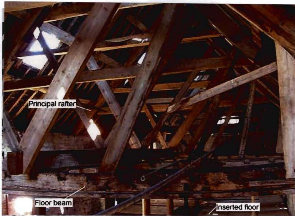
Figure 3: Internal view of the Riding House, looking towards the east end
