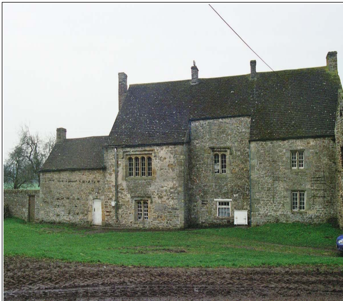
Figure 2: Low Harperley farmhouse, viewed from the north
