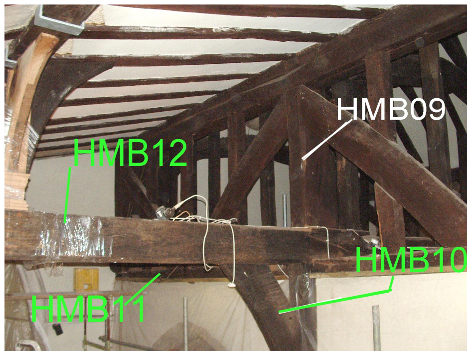
Figure 5: Inner north aisle roof, looking south-east towards the inner nave, showing timbers sampled
