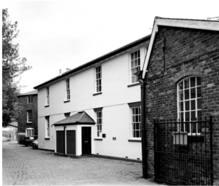
Fig 57. The Offices, originally single-storeyed, now raised to two storeys. (BB001893)
