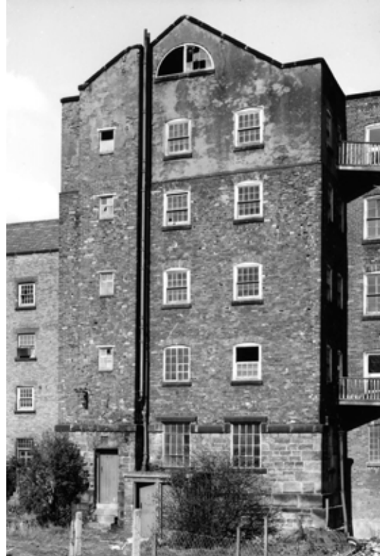
Fig 15. The south gable wall of Long Mill in 1975. (BB82/6264)
