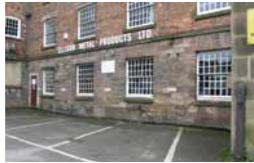
Fig 39 (left). The north elevation of West Mill in 1975. The rainwater fall pipe roughly marks the junction between the two phases of construction. (BB82/6265)
