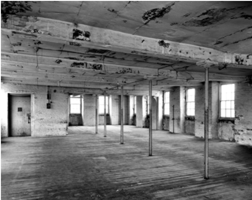
Fig 16. The interior of the third floor from the south-west. (BB001906)
