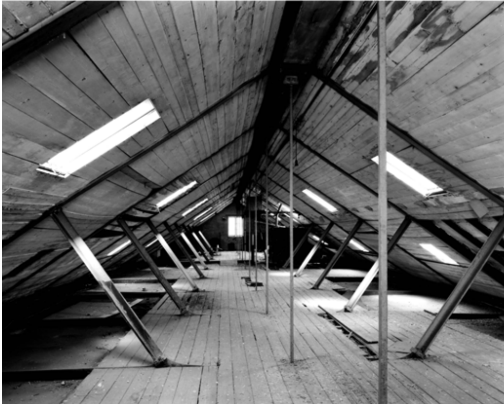
Fig 49. The main roof of North Mill, viewed from the west. (BB001931).
