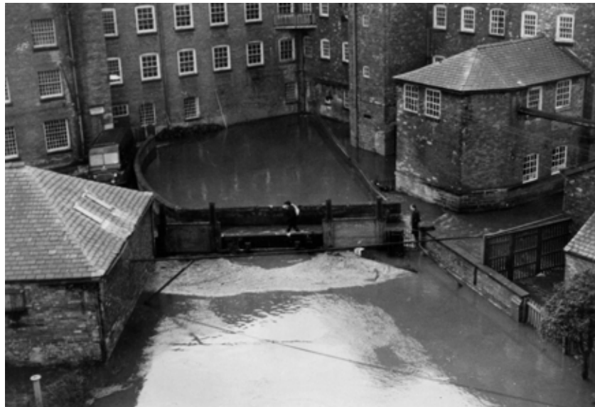
Fig 5. Flooding was a recurrent hazard of water-powered sites, with the potential to interrupt production and sometimes worse. Here the leat upstream of Middle Mill is seen spilling over onto Old Lane. (BB001871; courtesy of John Nelson)
