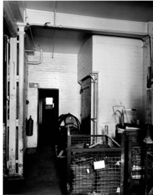
Fig 50. The westernmost bay of the ground floor, from the north. (BB001928)
