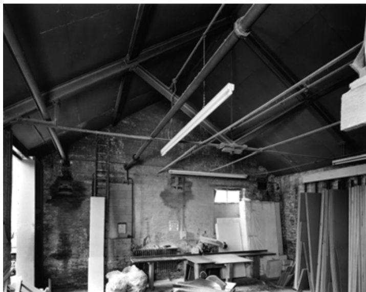
Fig 70. The interior of the four-bay range from the north. (BB001932)
