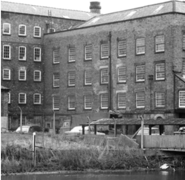
Fig 39 (left). The north elevation of West Mill in 1975. The rainwater fall pipe roughly marks the junction between the two phases of construction. (BB82/6265)
