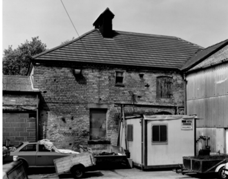
Fig 63. The stable from the south. (BB001898)
