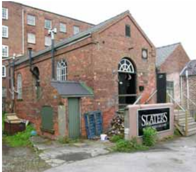
Fig 76 (above). The engine house from the south-west with the Bobbin Shop to the right. The paving immediately to the left of the engine house marks the former edge of the leat passing beneath Middle Mill.
