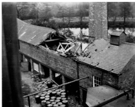
Fig 64. The now-demolished range south of the stables, as seen following damage caused by an explosion in 1938. (BB001867; courtesy of John Nelson)
