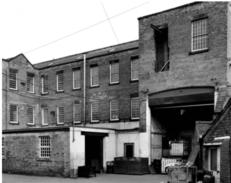
Fig 46. The rear elevation of North Mill, from the north-west. (BB001896)
