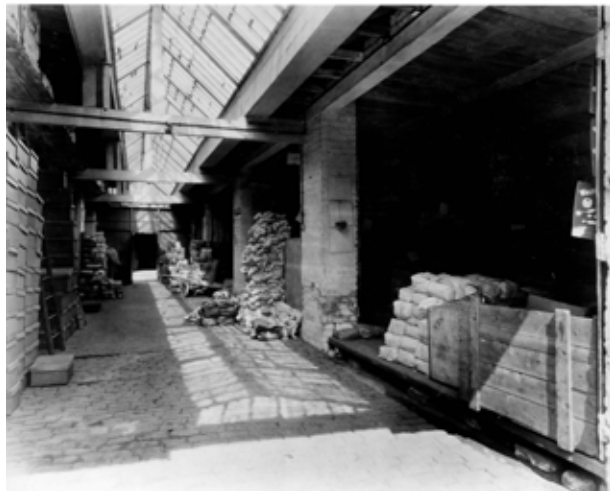
Fig 31. The open-fronted shed, as depicted in a photograph dating from c1930, by which time a north-lit roof linked it with the adjoining building to the west. (BB001860; courtesy of John Elliott)
