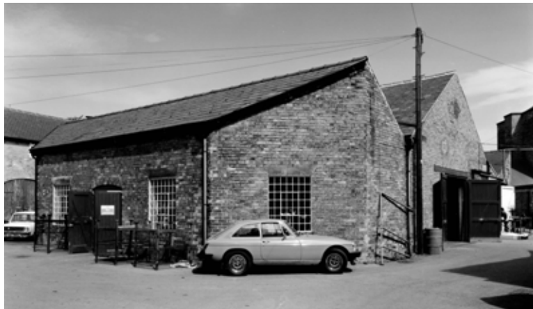
Fig 61. The earliest part of this range of buildings is the taller block to the rear. Canted corners on the nearer block assisted vehicular movement around this cramped part of the mill site. (BB001899)
