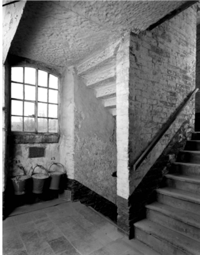
Fig 54. The stair in the north-west corner of Long Mill. An exposed timber beam is visible top left, and timbers used to form the windows were left similarly un-plated, but the stair is considerably less vulnerable to fire than the timber stairs commonly found in early cotton mills. (BB001904)
