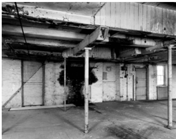
Fig 79. Evidence for the removed rope race transmission in Long Mill. (BB001907)
