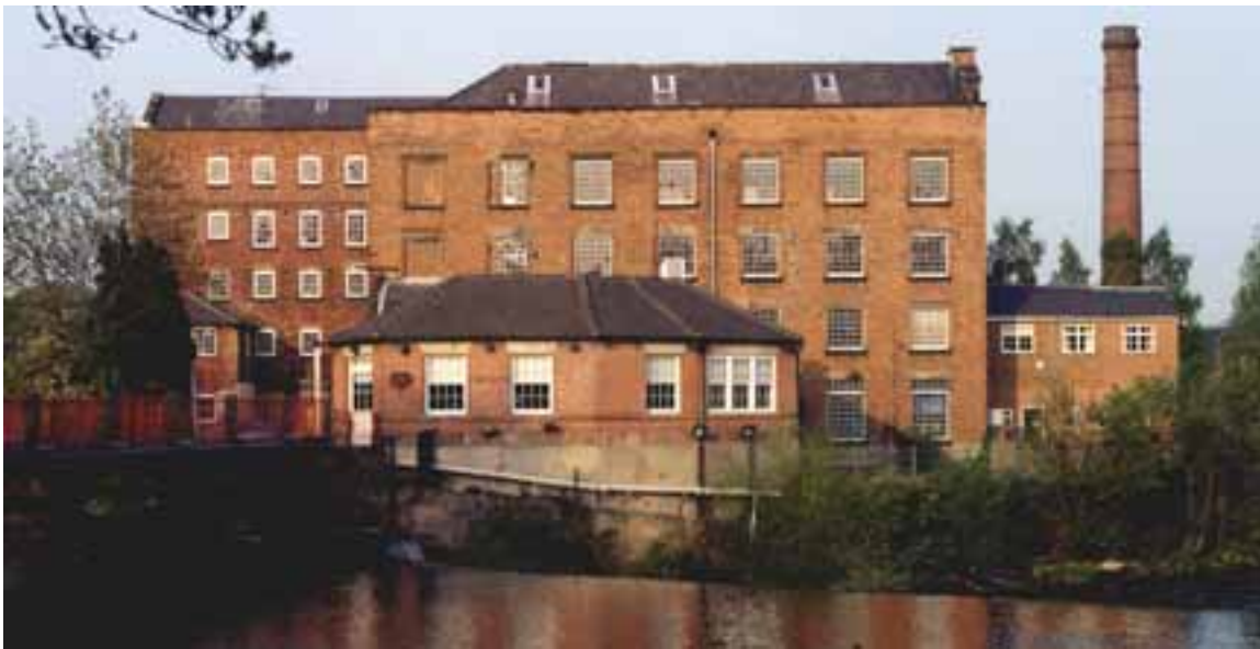
Fig 41. The west elevation of West Mill, showing the blind windows (and parts of windows) corresponding to the stair compartment at the north end. The single-storey building in the foreground is the former mill dining room, now a restaurant. (BB001880)
