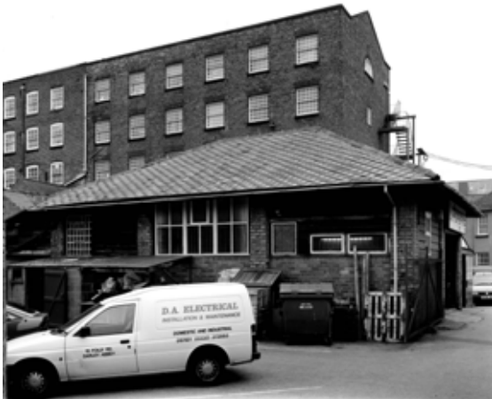
Fig 72. The coppice barn (22) from the south-east. The roof slates are laid so as to permit ventilation. (BB001885)
