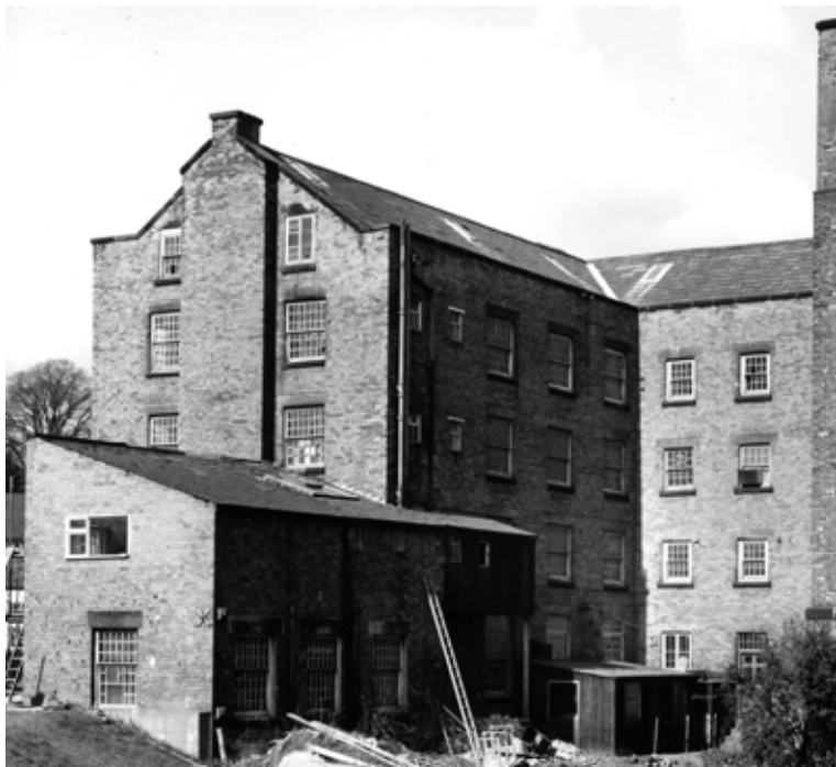
Fig 38. West Mill from the south-east in 1975, showing the L-shaped plan. The leat passed beneath the right-hand range. (BB82/6264)
