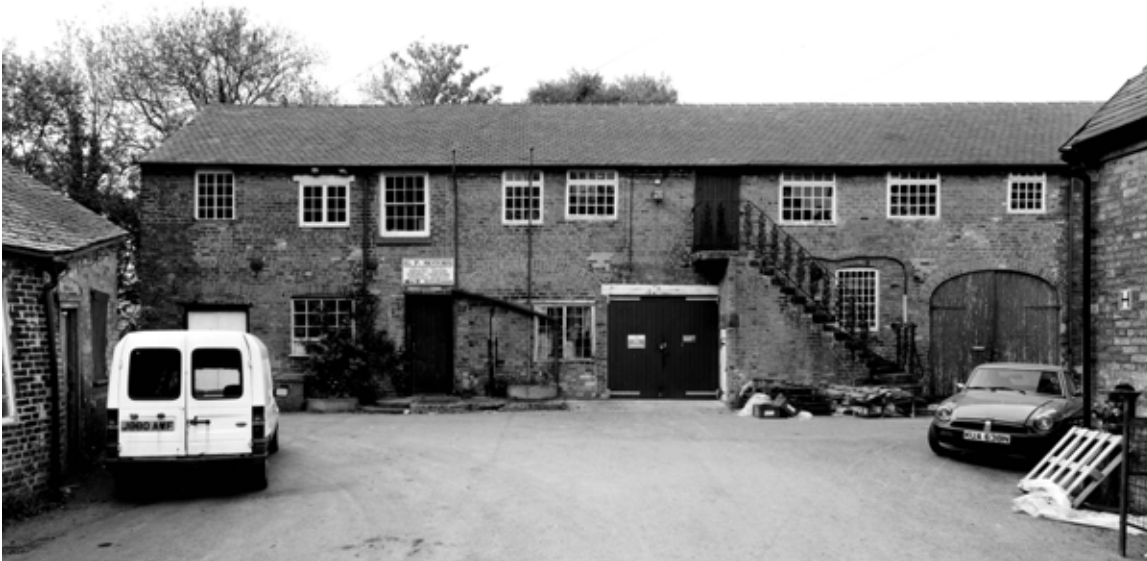
Fig 26. The western portion of the proto-fireproof range from the south. (BB001900)
