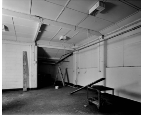
Fig 73. The interior of the coppice barn (22). The roof has been underdrawn, but would originally have been exposed. (BB001886)
