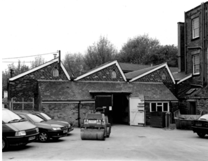
Fig 86. The east elevation of the Polishing Shed, showing the north-lit roof and Gothic-style gable windows. (BB001890)
