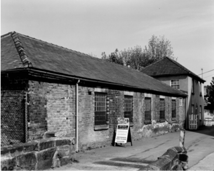
Fig 74. The gassing shed from the west, with the house, 5 Old Lane, beyond. (BB001888)
