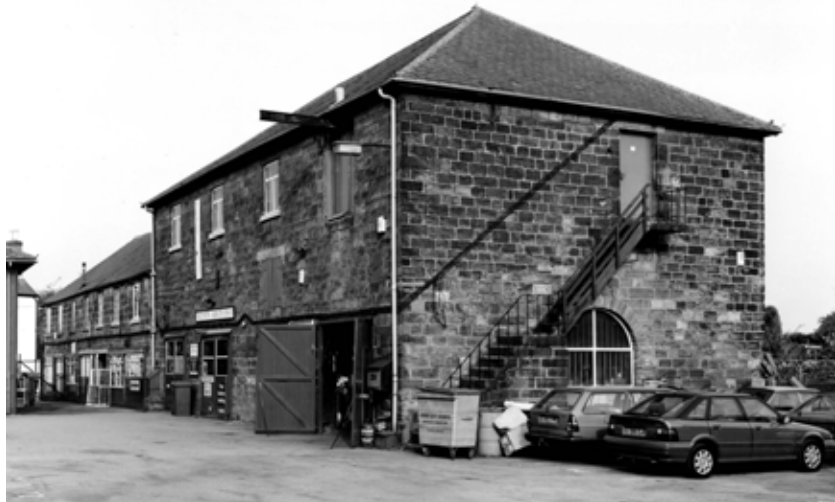
Fig 58. The western block, with the lower eastern block beyond. (BB001882)
