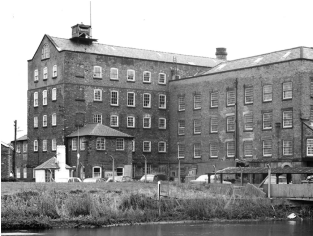
Fig 13. Long Mill from the north-west in 1975, with West Mill to the right. The brickwork of the fourth floor and attic retains traces of render. The structure on the ridge is the Second World War ARP post. (BB82/6265)
