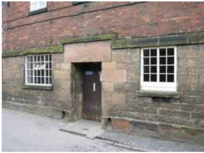
Fig 55. The inserted north entrance to Long Mill. The window to the left, widened leftwards probably at the same time, lights the counting house.
