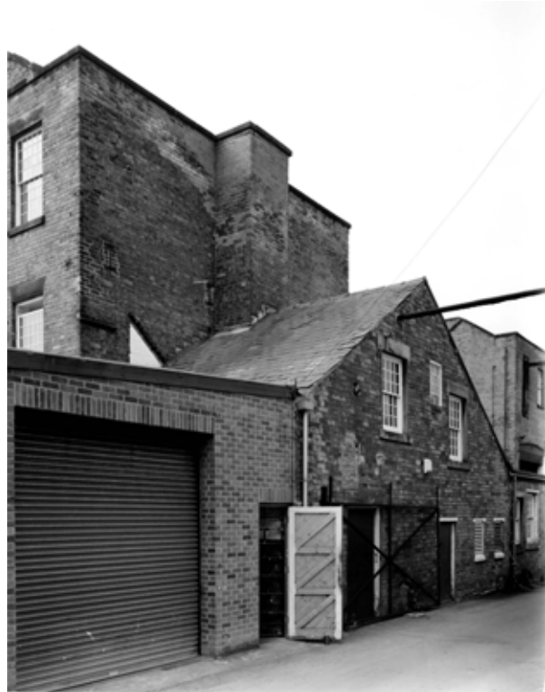
Fig 47. The more easterly of the two ranges projecting on the north elevation of North Mill, from the north-east (BB001897).
