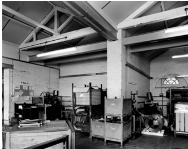
Fig 52. The interior of the engine house (left) and boiler house (right). (BB001925)
