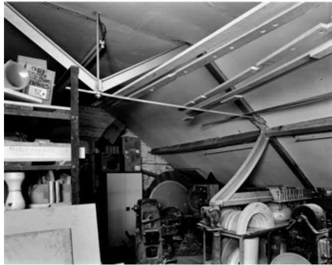
Fig 69. Interior of the two-bay range, showing the unusual form of the cast and wrought-iron roof truss. (BB001933)
