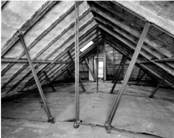
Fig 43. The roof of the east-west arm. (BB001914)
