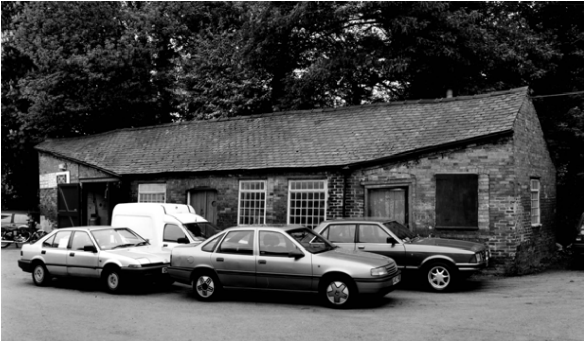
Fig 65. The Fire Station from the east. (BB001901)
