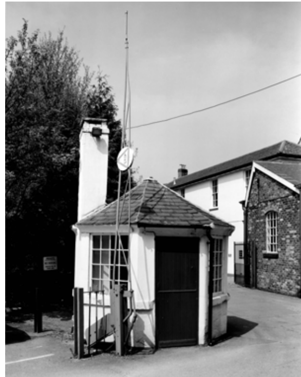
Fig 56. The watch house from the south. The present entrance is a later insertion. (BB001892)
