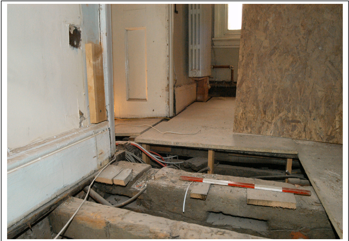
Figure 3a/b: Photos of one of the moulded timbers used as a joist (top) and the timbers of the stairwell (bottom)
