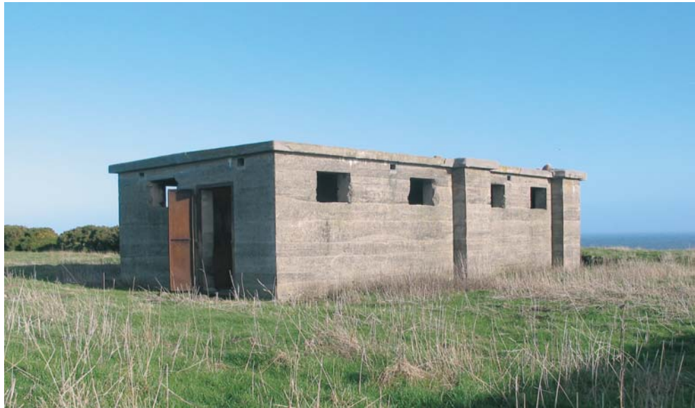
Figure 10 The TxRx Block viewed from the south-west. Note the surviving metal door at the western end of the building.
