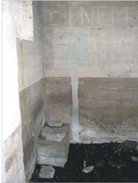
Figure 12b The interior of the eastern room of the TxRx Block, showing further evidence of the positioning of equipment within the building
