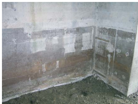
Figure 12a The gaps in the paintwork show the position of equipment and wiring within the TxRx Block
