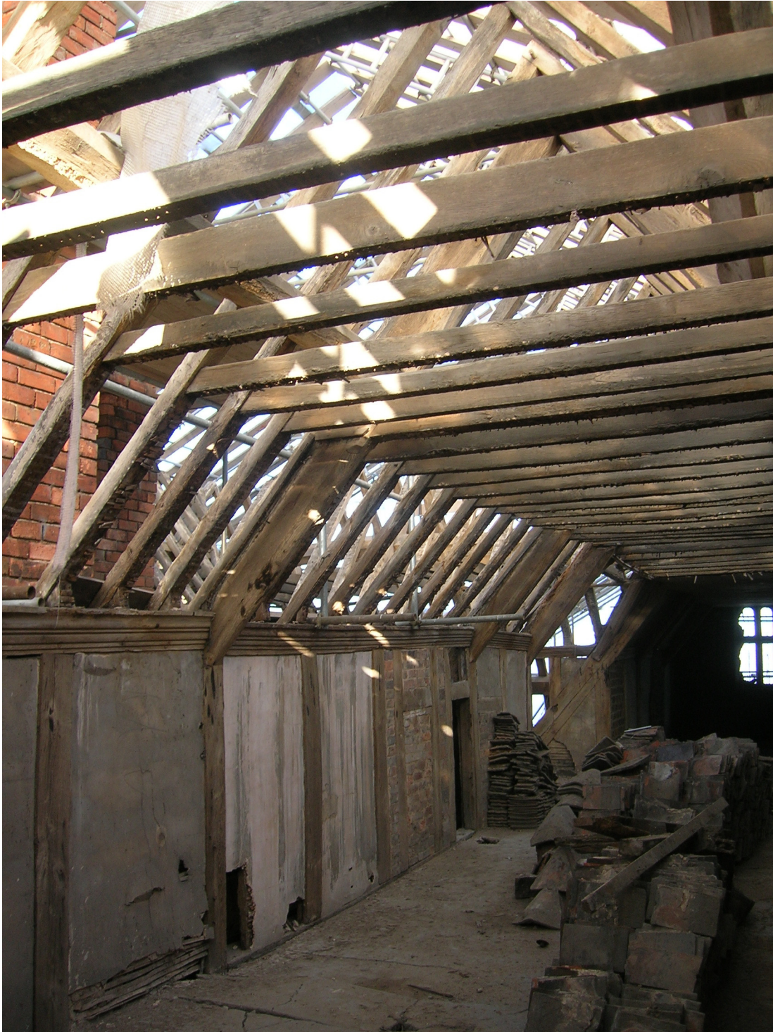
Figure 3: Kingsbury Hall, Warwickshire; South Range roof (looking north-east)
