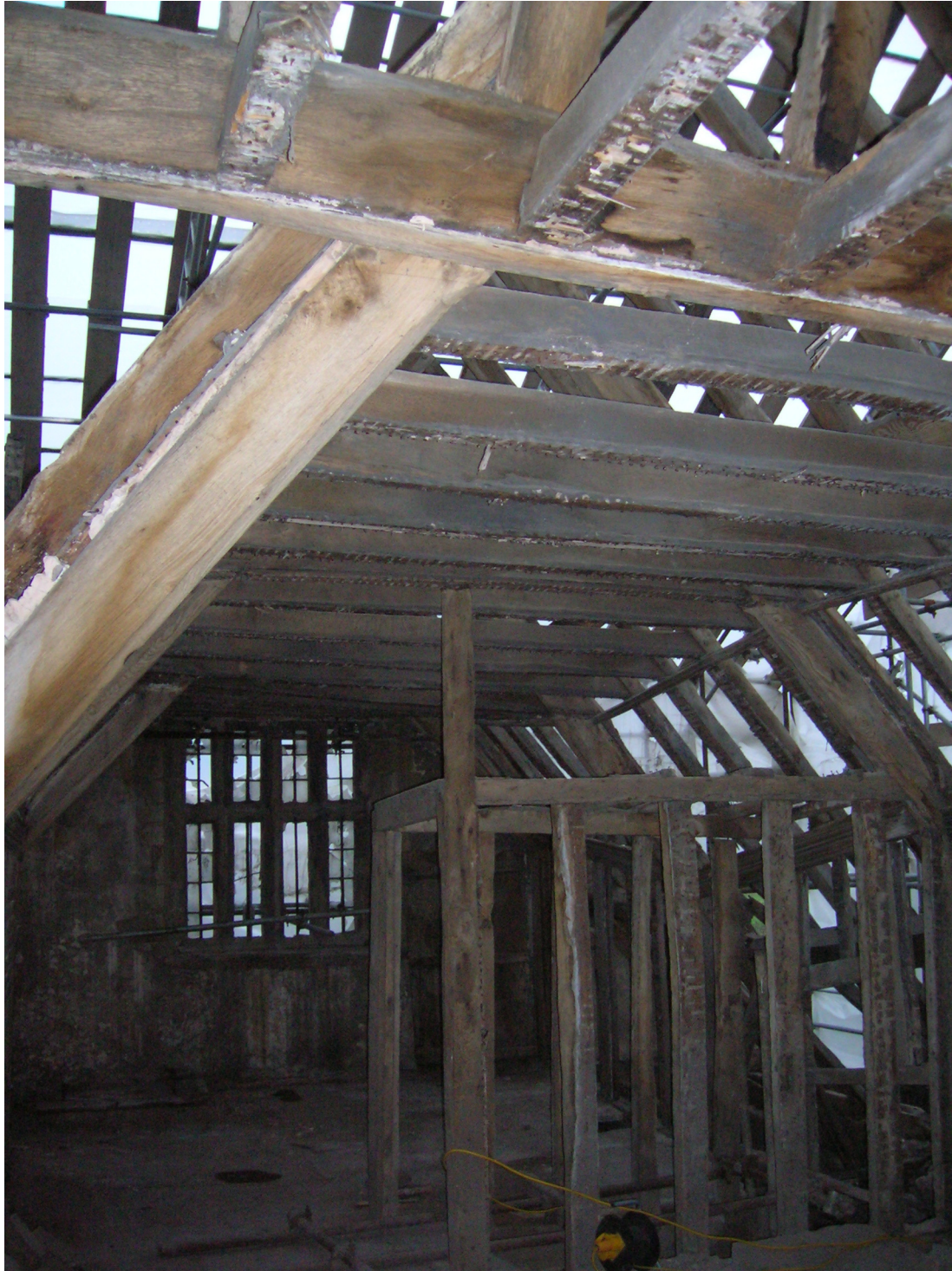
Figure 4: Kingsbury Hall, Warwickshire; East Range roof (looking north)
