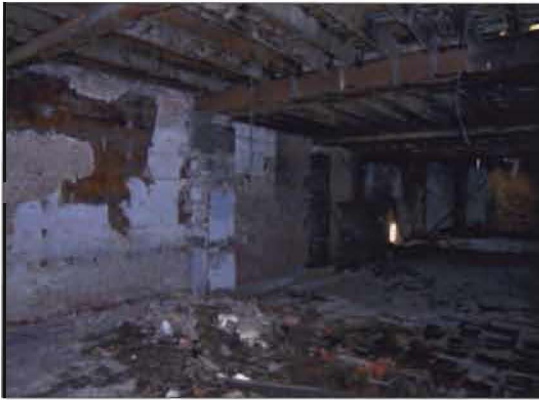
Figure 3. The ground-floor shop interior. Pete Smith 5/10/2006
