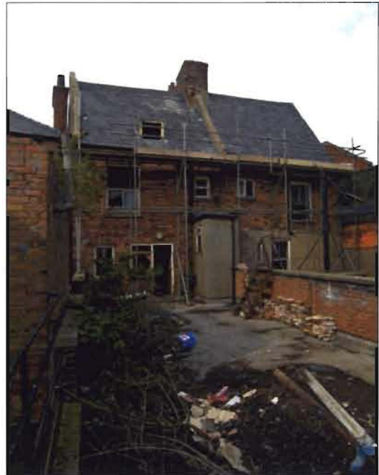
Figure 2. The rear south-east front, from the roof of the ground floor rear extensions. Pete Smith 5/10/2006
