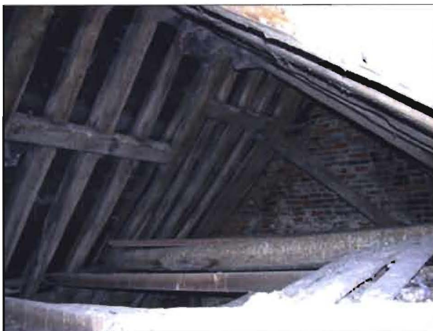
Figure 7. Interior of rear roof. Pete Smith 5/10/2006
