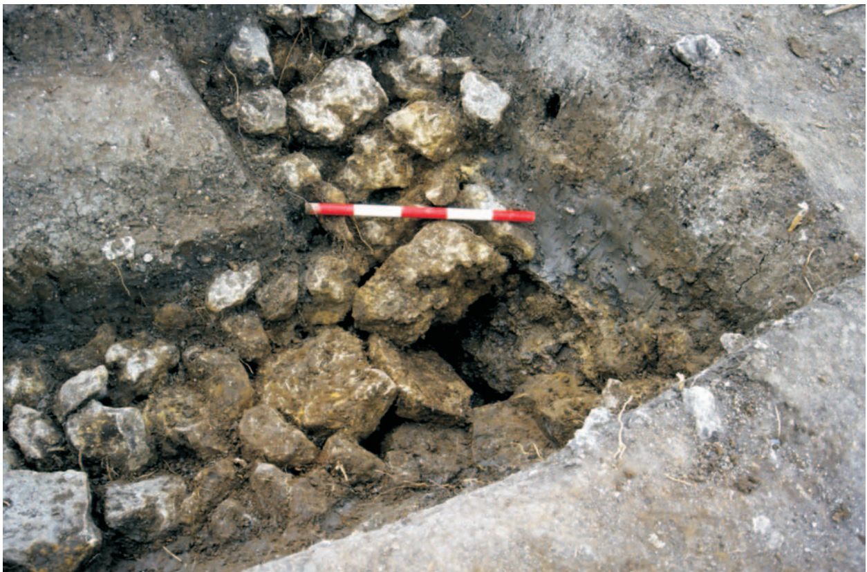
Figure 4. (below) Trench 5 post-medieval culvert showing junction of main north-south culvert (upper element) with branch joining from west and cap-stone removed. View near vertical/north-east. Photo © English Heritage
