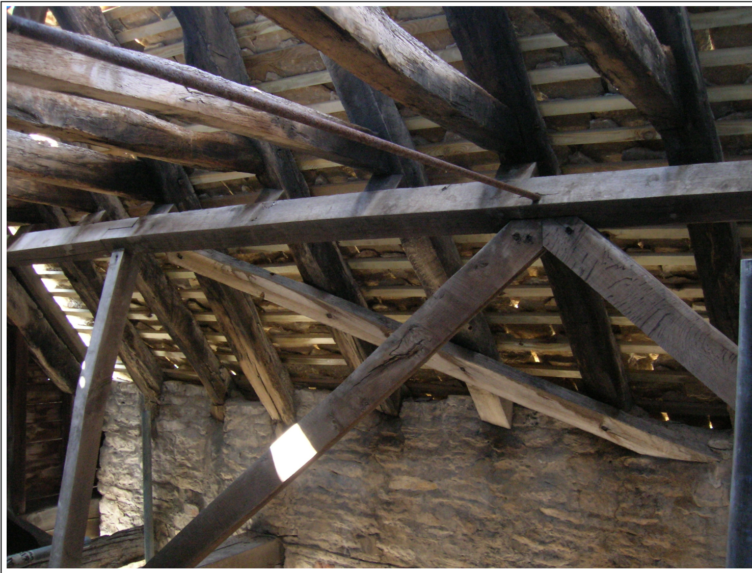
Figure 4: North side, showing one of the 'inserted' nailed-on braces
