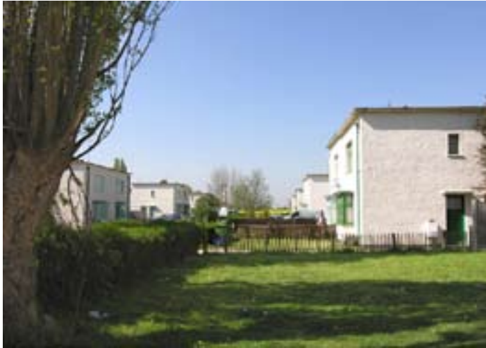
Figure 52 Bata Avenue, viewed from the east, in 2007 (DP040059)
