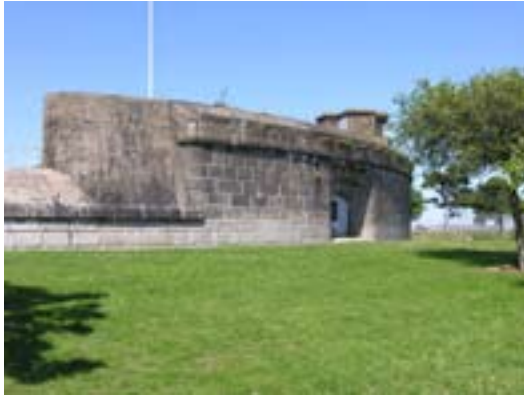
Figure 30 Casemates of Coalhouse Fort (DP040046)
