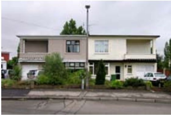
Figure 58 Managers' houses, 1-2 Queen Mary Avenue (DP040036)
