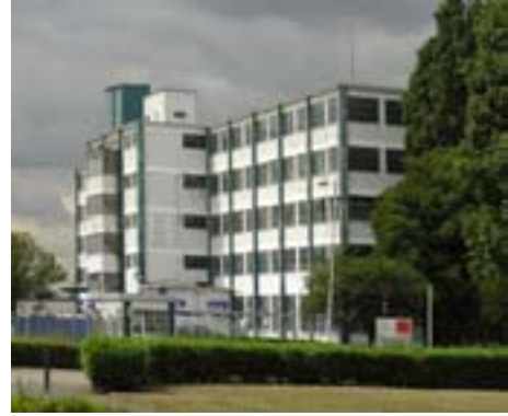
Figure 38 Trafalgar House (originally building 13), the first of the multi-storey blocks (DP040061)
