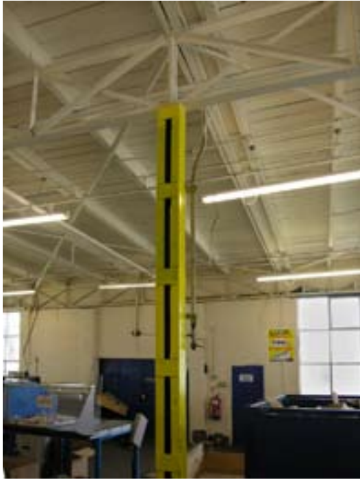
Figure 41 Detail of the construction of building 12, taken in 2006 (DP040052)
