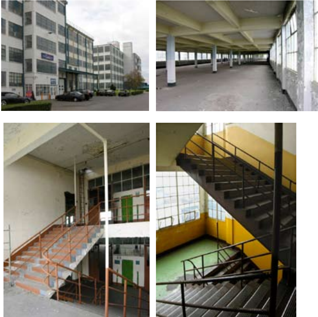
Figure 43 (top left) Exterior of Nelson House and Victory House (DP040067); figure 44 (top right) Third floor, Trafalgar House (DP040042); figure 45 (bottom right) Stairs, Nelson House (DP040043); figure 46 (bottom left) Stairs, Trafalgar House (DP040041)
