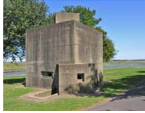
Figure 31 Concrete observation tower with the moat of Coalhouse Fort behind. (DP040070)
