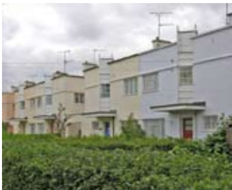
Figure 68 Modern Movement houses, Silver Street, Silver End, Essex (DP040058)
