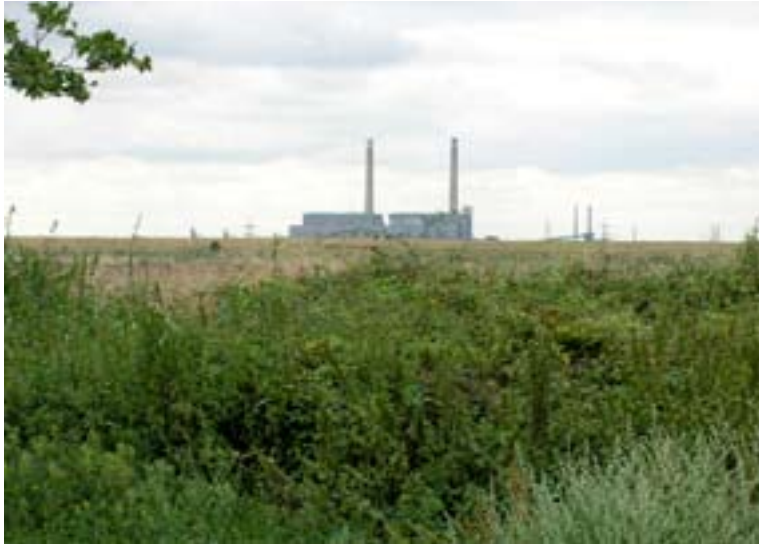
Figure 66 Tilbury Power Station, as seen from Coalhouse Fort car park (DP040066)
