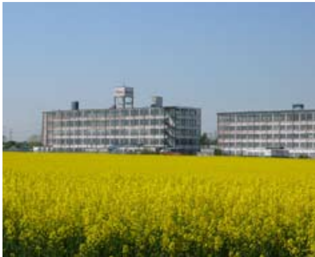
Figure 71 The former Bata Factory, viewed across a field of rape, in 2007 (DP040060)
