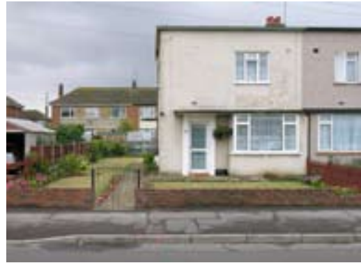
Figure 59 Princess Margaret Road housing viewed from Thomas Bata Avenue (DP040037)
