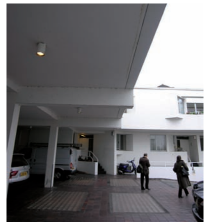
Fig. 6: The car port, with piloti for the upper floor. (DP040011)
