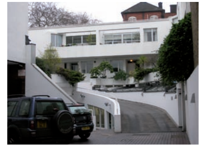
Fig. 7: The car ramp from the west (DP040019)
