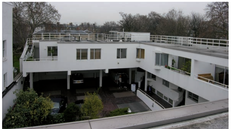
Fig. 3: View looking north from the roof (DP040009)
