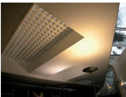
Fig. 19: The offices are lit by a mixture of pavement lights, glazing and artificial lighting (DP040017)
