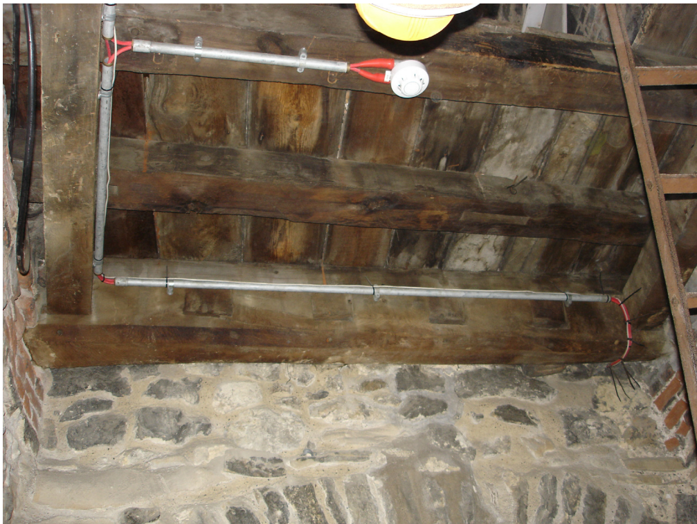
Figure 40: Beam and joist comprising lower floor of south-east turret
