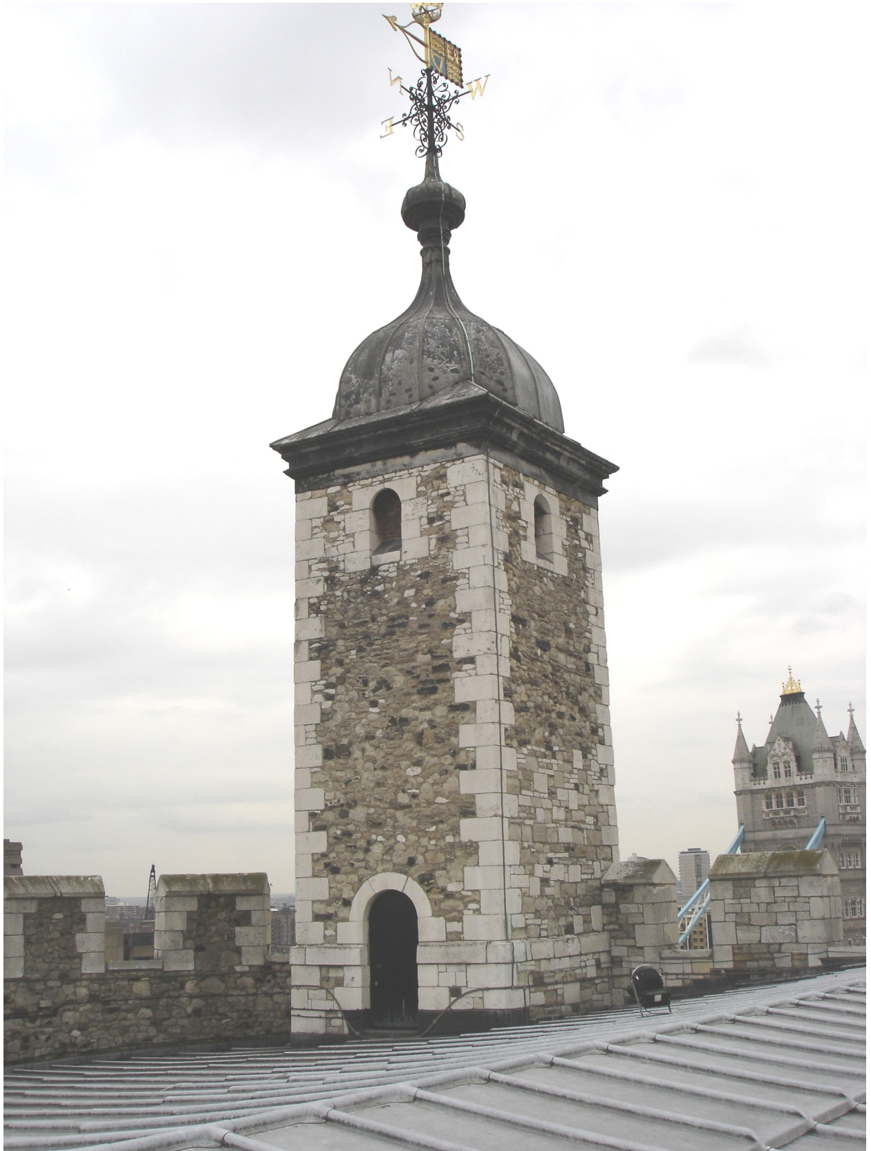
Figure 39: View of south-east turret
