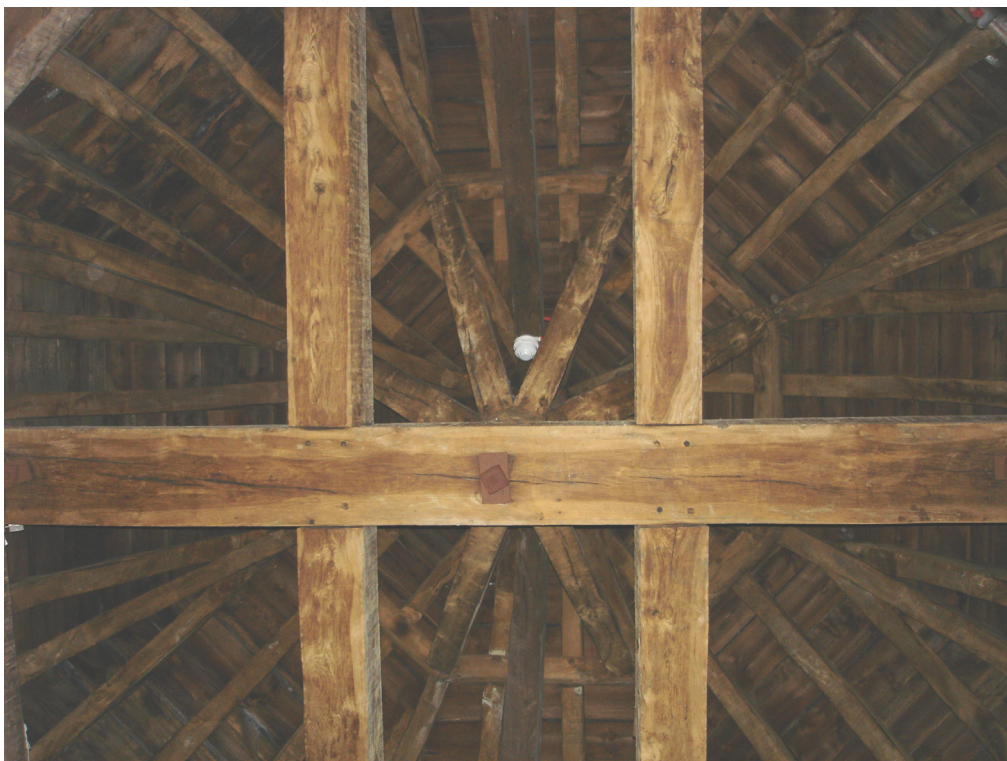
Figure 38: Roof, north-west turret
