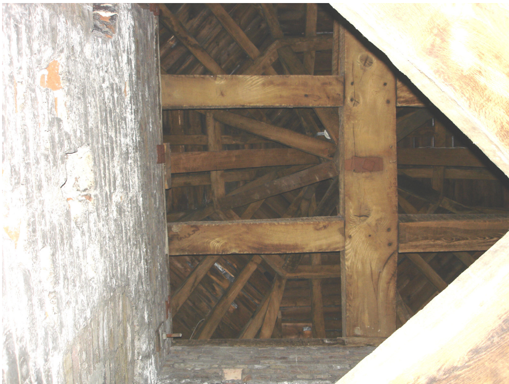
Figure 45: View of roof inside south-west turret
