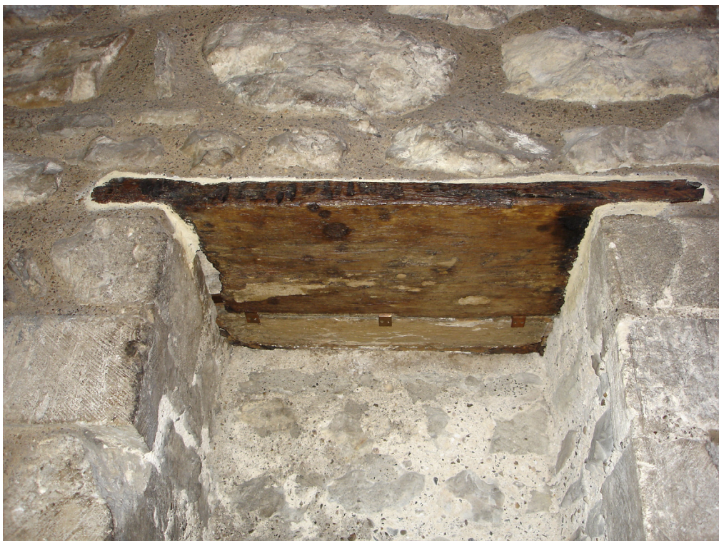
Figure 11: First-floor lintel over cupboard recess in north-west embrasure (wt19)
