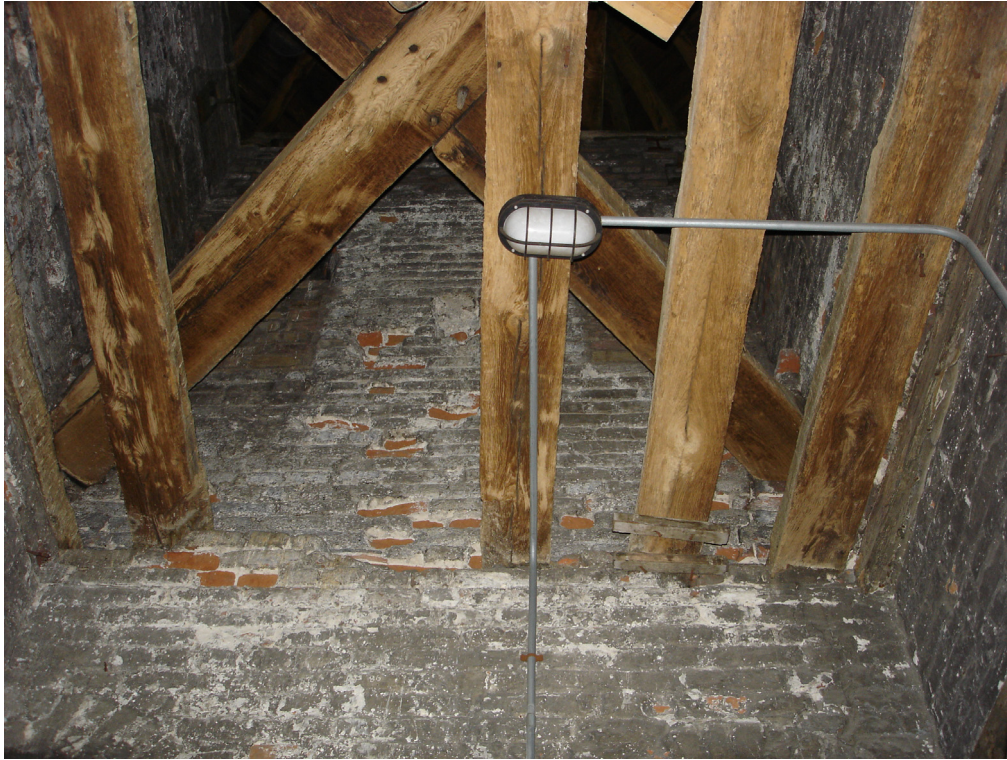
Figure 44: Second-floor details and cross-braces in south-west turret
