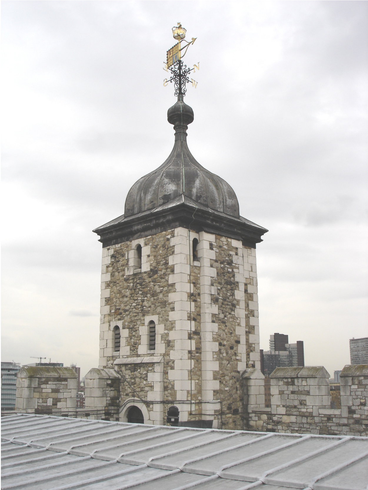
Figure 43: View of south-west turret
