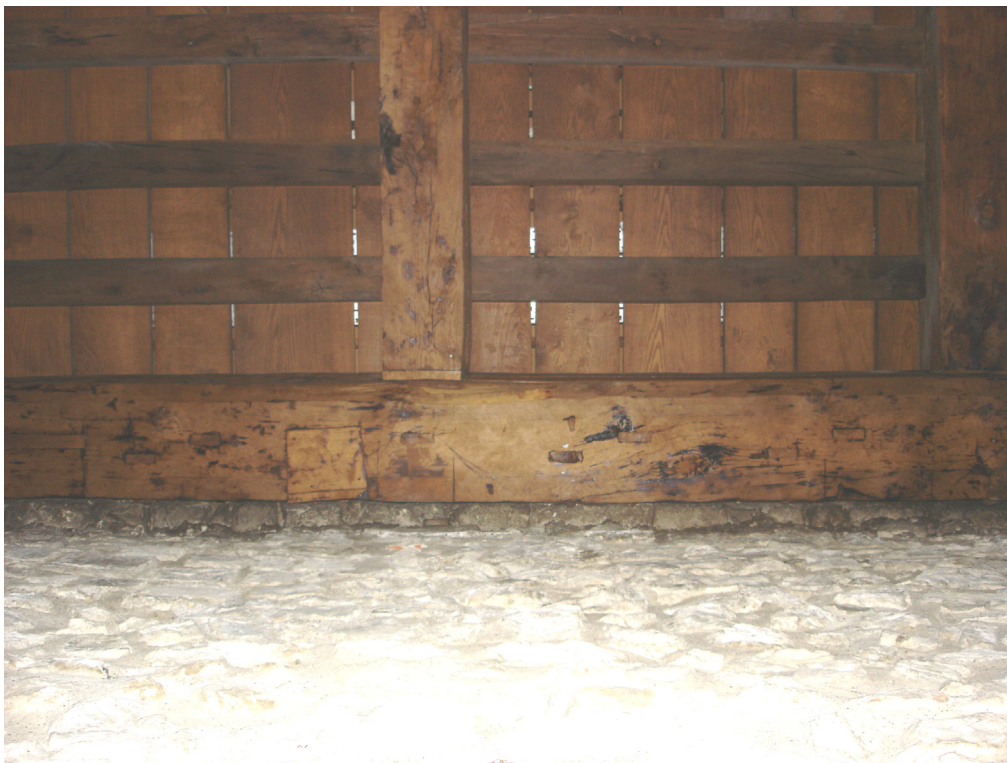
Figure 27: Southern tiebeam of western room roof showing blocked mortices
