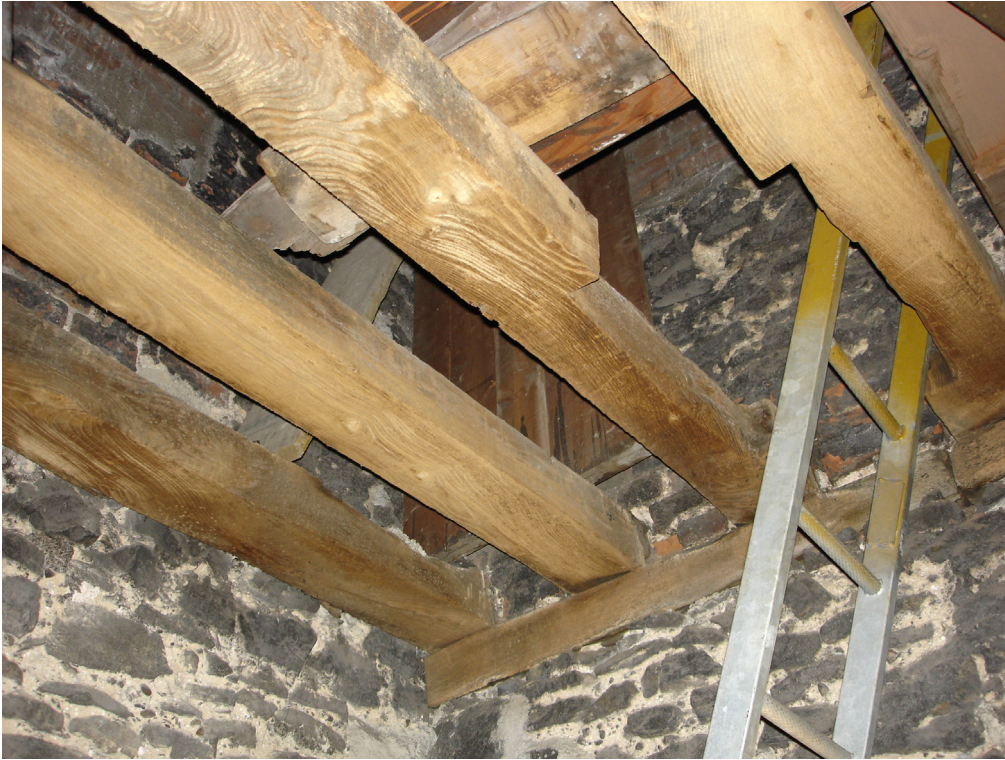
Figure 41: Second-floor details of south-east turret
