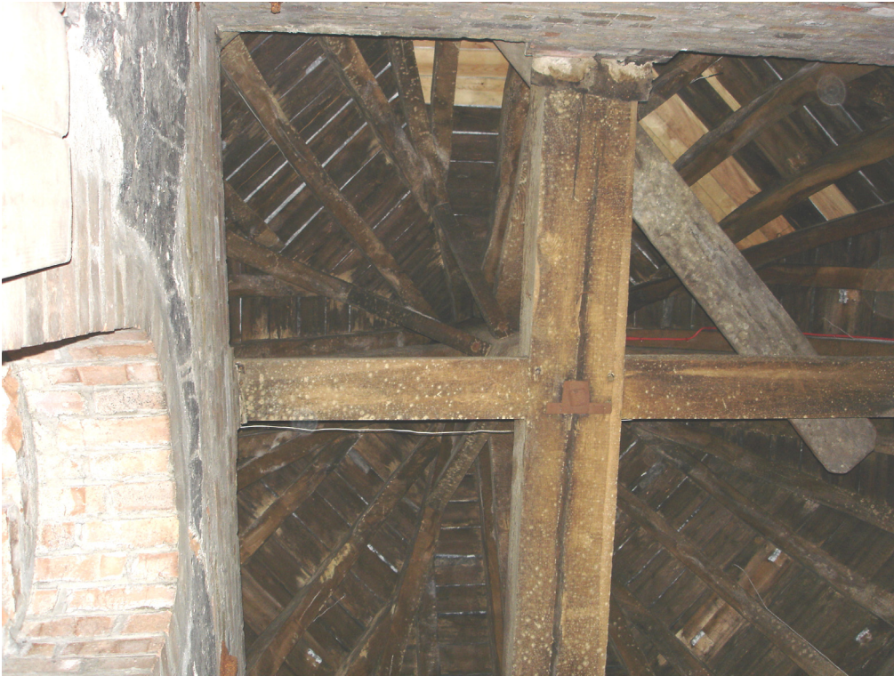
Figure 42: Underside of roof of south-east turret
