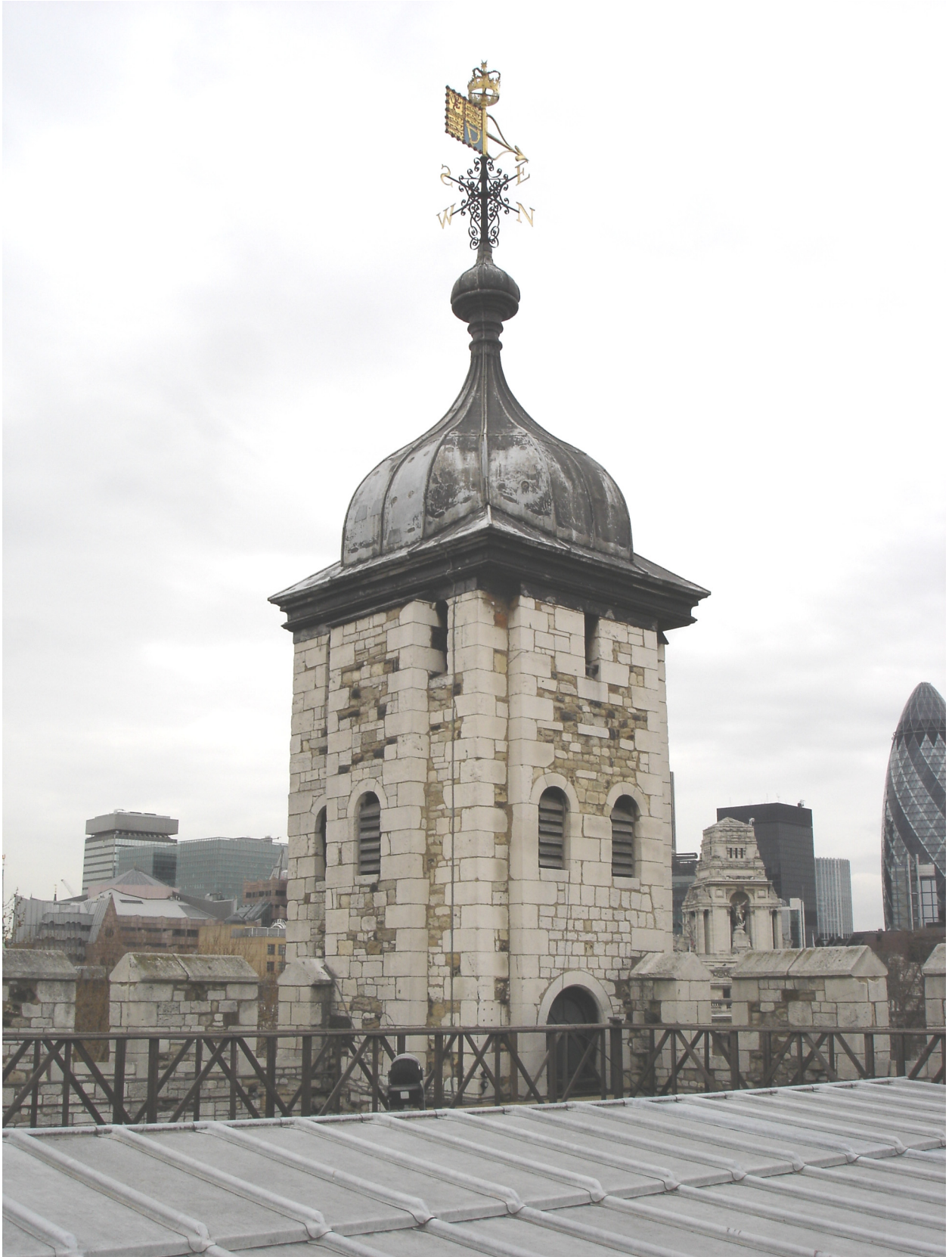
Figure 36: View of north-west turret
