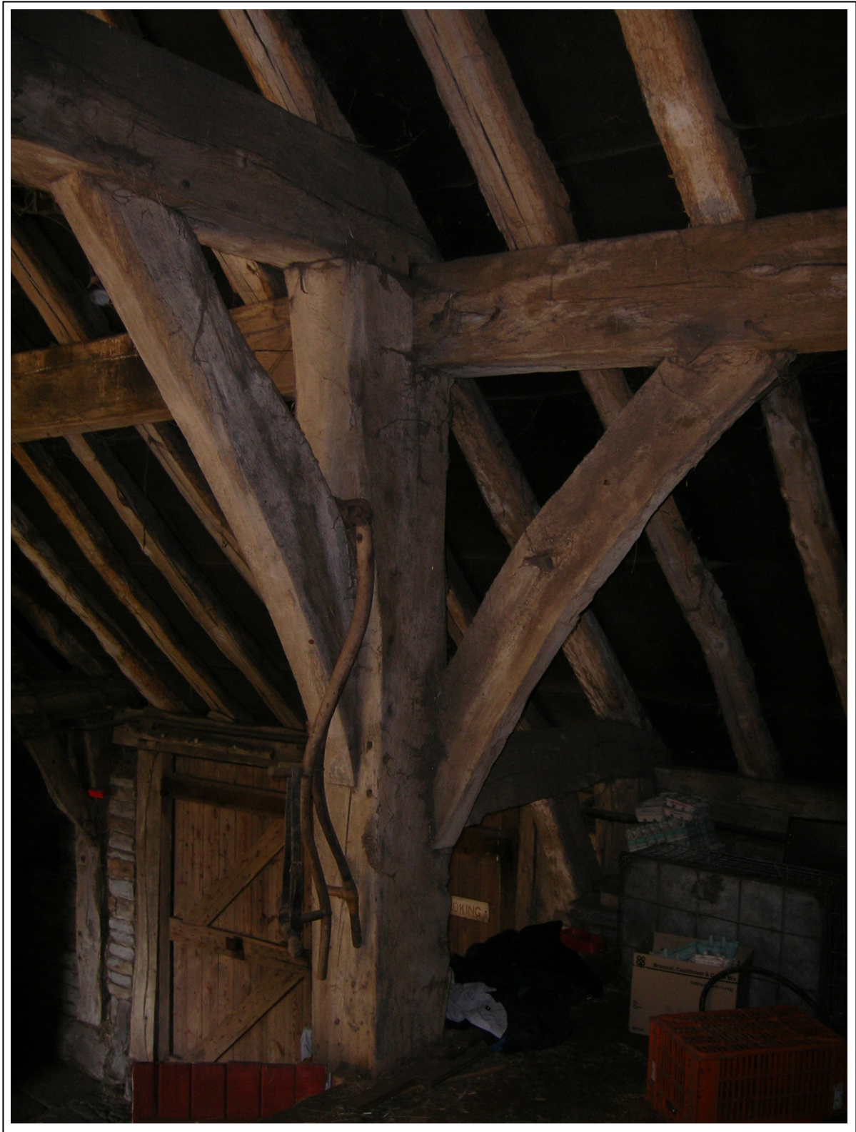
Figure 4: East arcade post braces, truss 2
