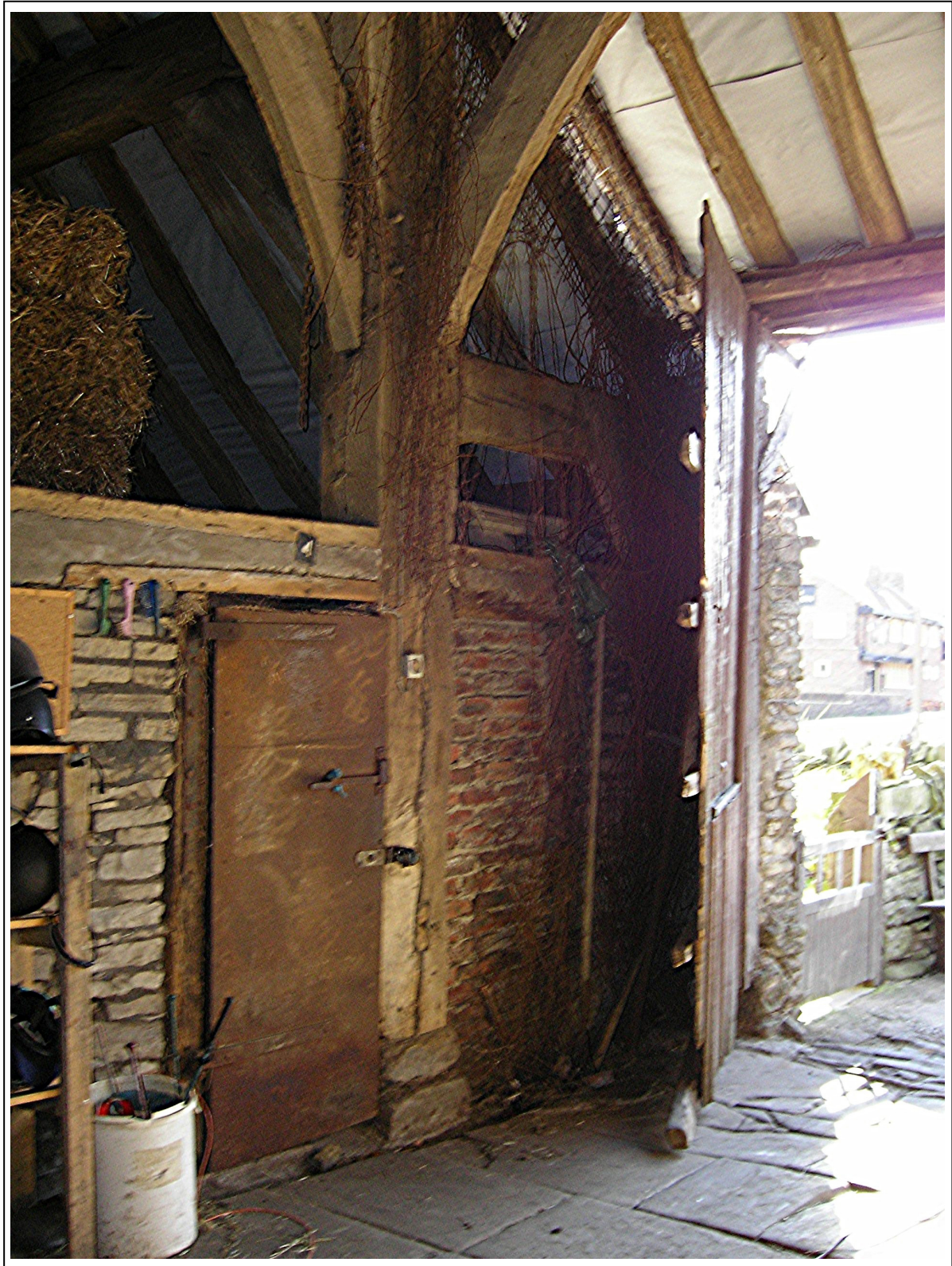
Figure 5: Truss 2 showing one of the arcade posts on a stone slab
