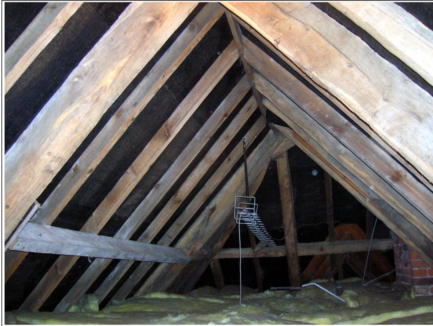
Figure 3: The Old Rectory; roof, looking west
