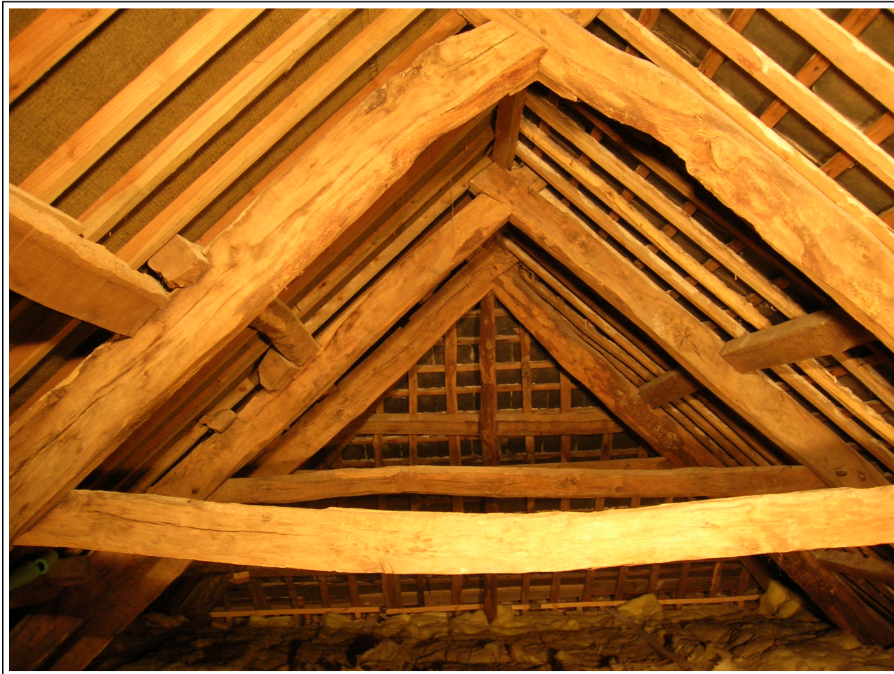
Figure 5: Western range roof truss; truss 3 in foreground
