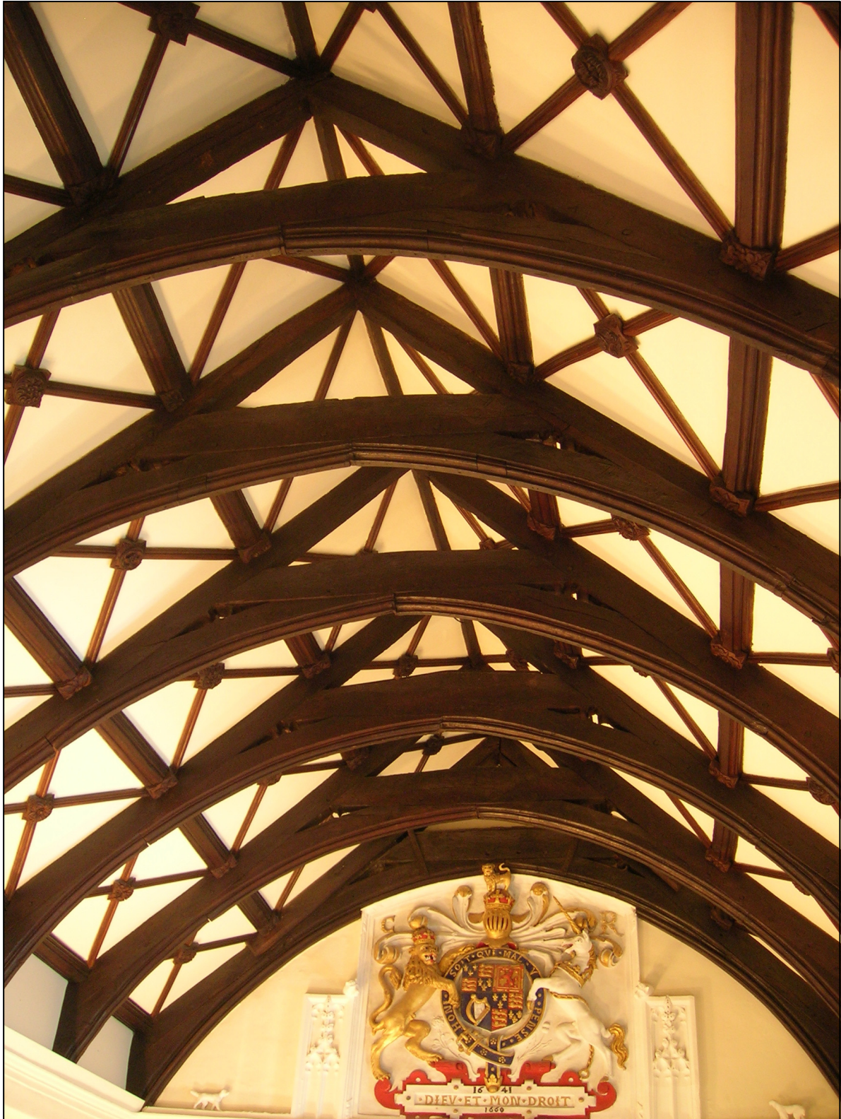
Figure 4: Chevy Chase room, roof structure (viewed from the west)
