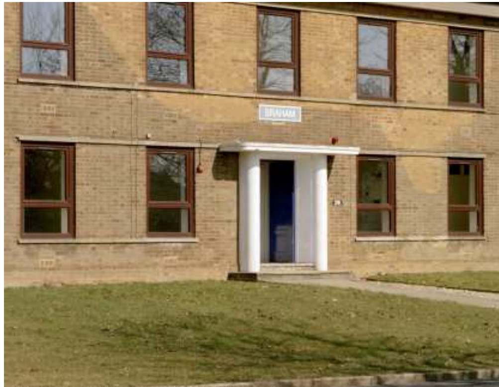
Figure 74 Braham, Building 27B, 1930s barracks to the northeast of the parade ground. Traces of wartime camouflage paint is still visible on many of the barrack buildings. (c) English Heritage AA054448
