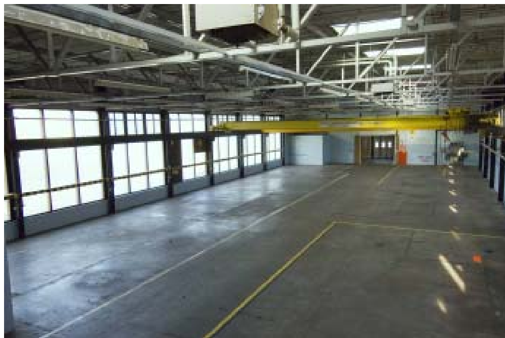
Figure 158 October 2006, Propulsion and Aircraft Components Flight (PACF) Adour Engine Assembly Facility. (c) English Heritage DP035662
