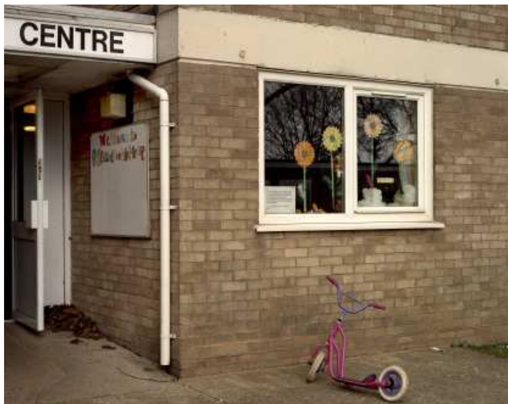
Figure 108 RAF Coltishall Amenities Centre, off Ormesby Road. (c) English Heritage AA054369
