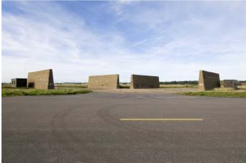
Figure 252 Eastern group of blast walls, 48 and 49 looking west. In 1956, in anticipation of the introduction of Javelin aircraft the airfield's runways and taxiways were strengthened, and two groups of eight pairs of Y-shaped blast walls built. Each group of blast walls was large enough to protect a squadron's aircraft. To either side of the blast walls were prefabricated huts for the aircrew and servicing personnel, their positions occupied by the more recent huts. (c) English Heritage DP035646
