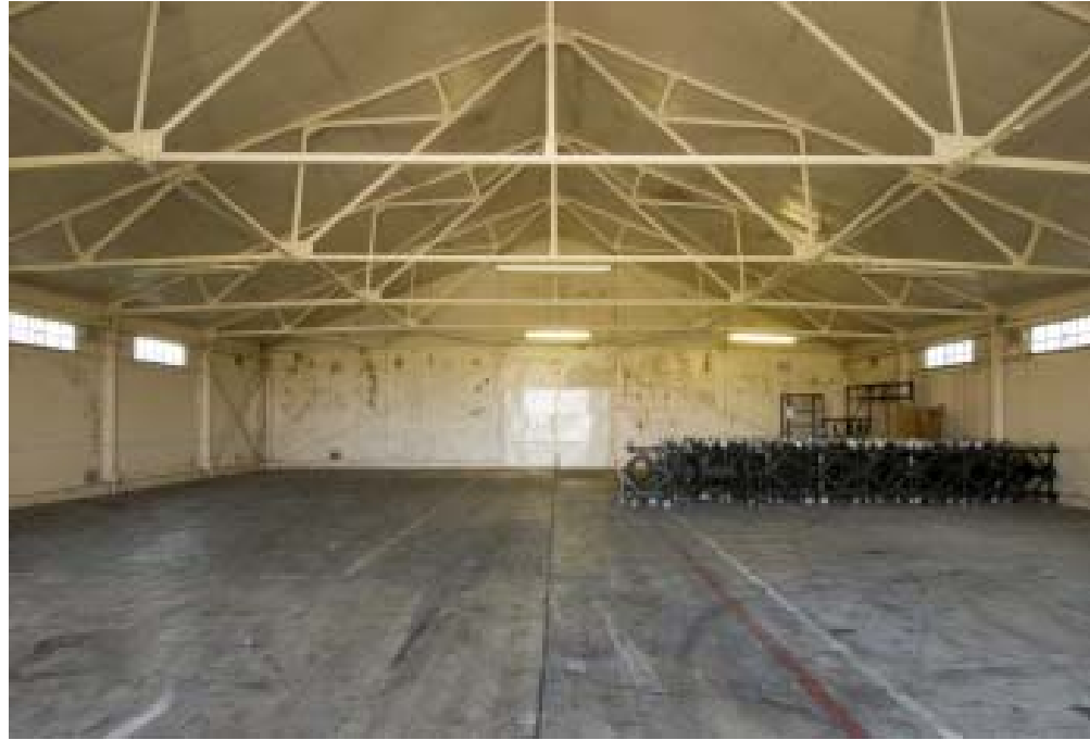
Figure 283 Missile and munitions storage area, 1950s missile storage building 223B interior from west. (c) English Heritage DP027165
