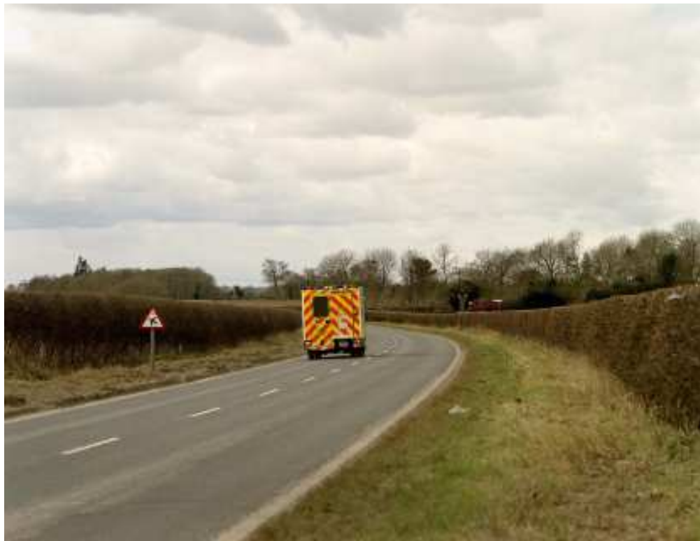
Figure 4 Scottow Road to the north of the airfield, built in the 1960s to link the villages of Buxton and Lamas to the B1150. This replaced an earlier route to the south which had been severed by the construction of the airfield. (c) English Heritage AA054358
