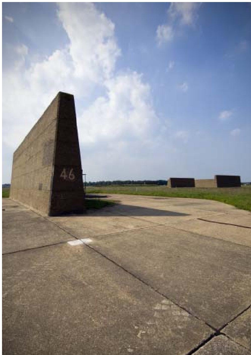
Figure 266 Late 1950s blast protection wal, eastern group wall 46. (c) English Heritage DP027174
