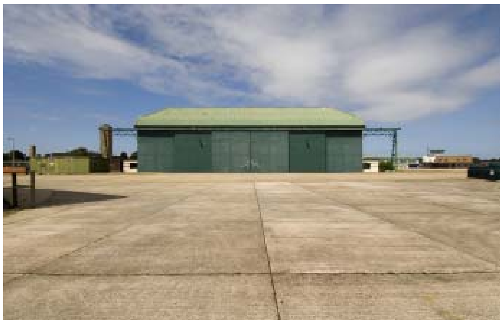
Figure 197 Hangar 3, south end. (c) English Heritage DP054394
