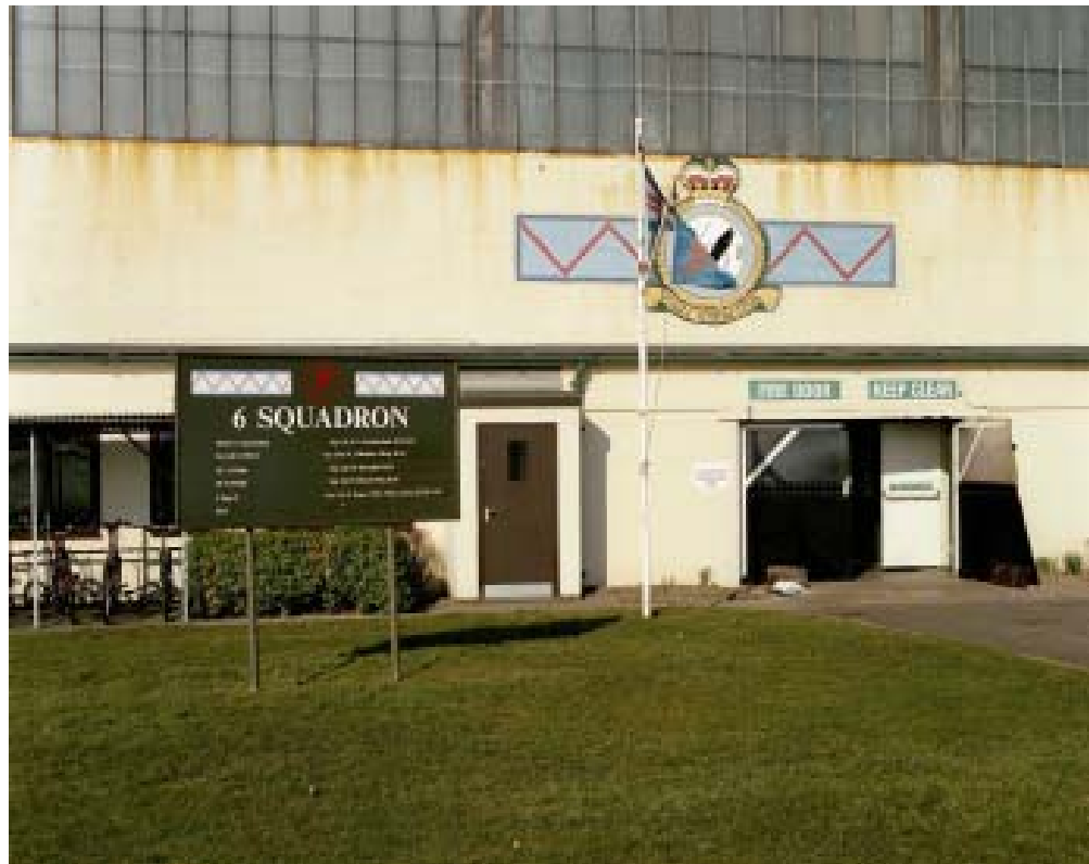
Figure 199 Hangar 3, 6 Squadron badge. (c) English Heritage AA054411
