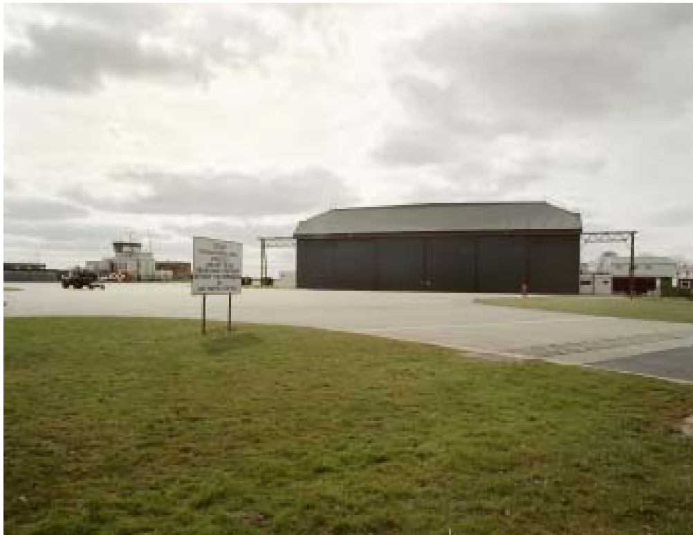
Figure 204 Hangar 2 north end (c) English Heritage AA054394
