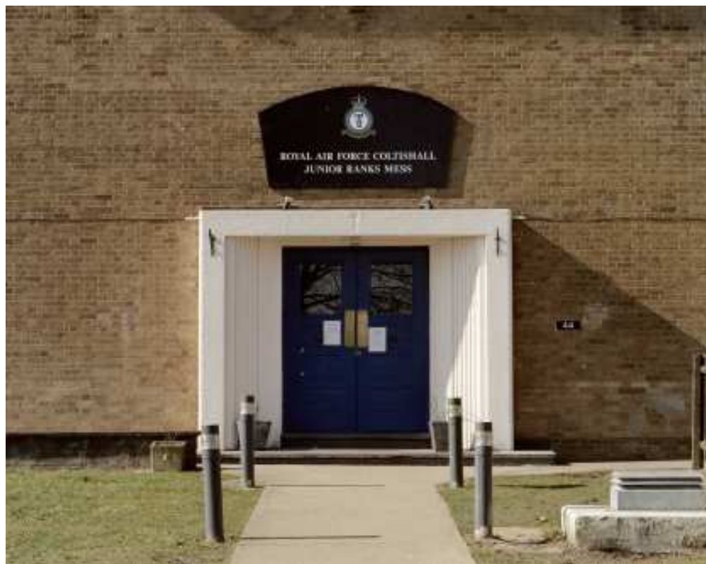
Figure 59 The airmens' institute, latterly Junior Ranks Mess, entrance. (c) English Heritage AA054450
