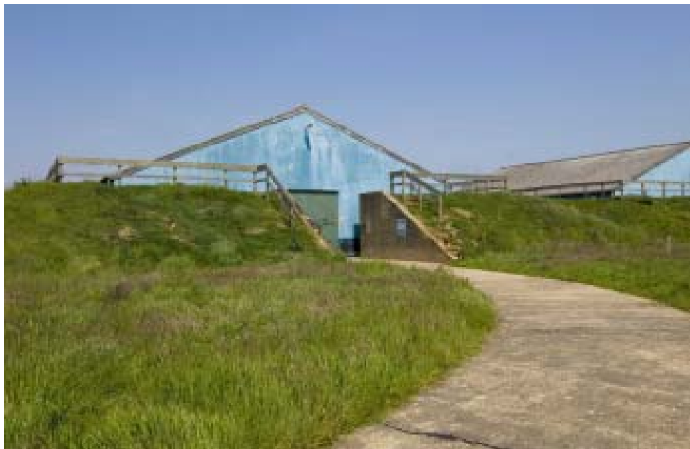
Figure 282 Missile and munitions storage area, 1950s missile storage building, from east. (c) English Heritage DP027178
