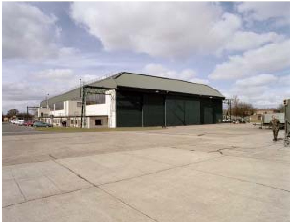
Figure 201 Hangar 4 from west. (c) English Heritage AA054390
