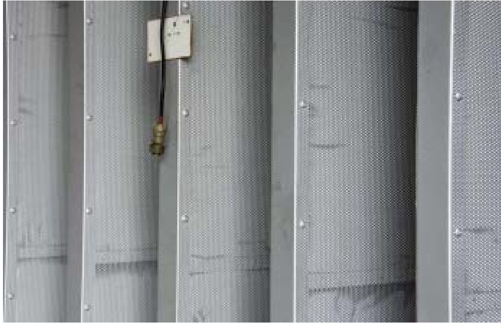
Figure 165 Uninstalled Engine Test Facility (UETF), detail of the air intake at the southwest end of the building. (c) English Heritage DP027324
