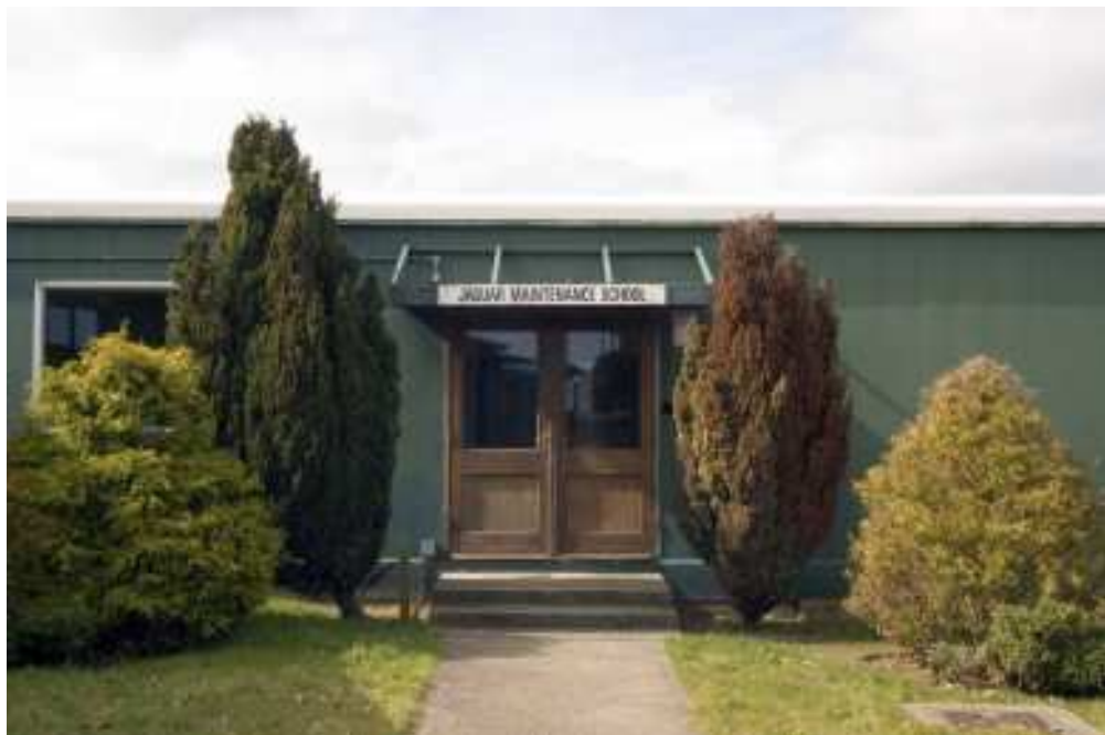
Figure 146 Building 280, Entrance to the Jaguar Maintenance School. (c) English Heritage DO029256
