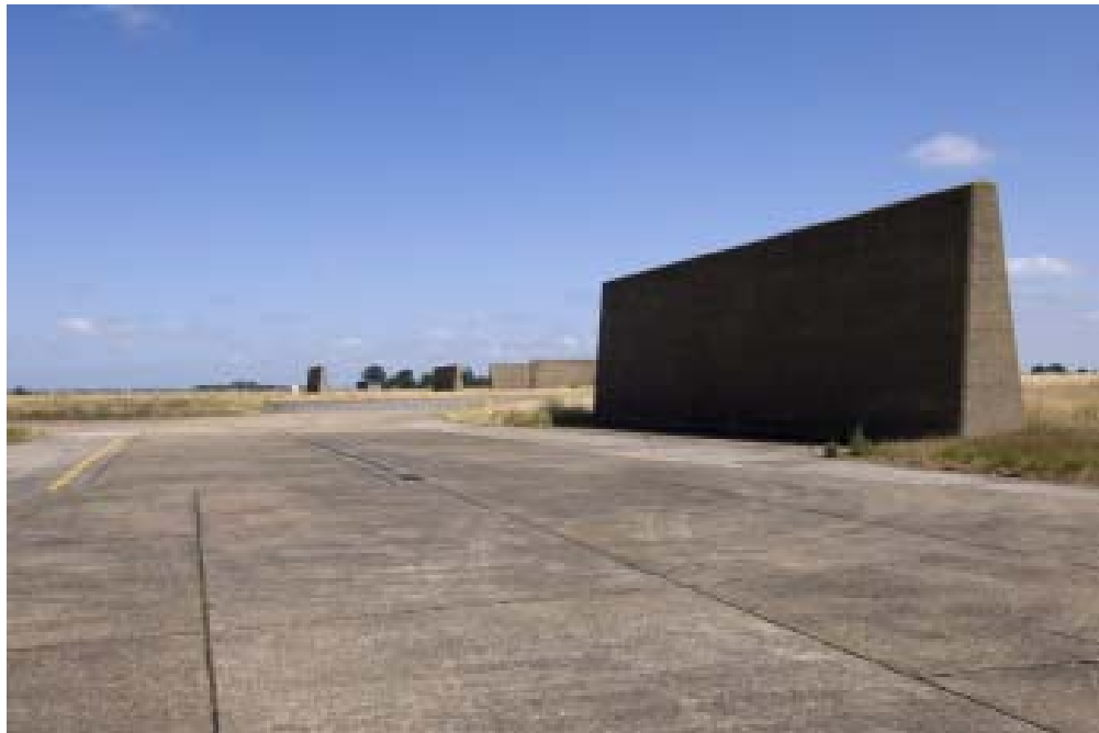
Figure 262 Late 1950s blast protection wall. (c) English Heritage DP027356
