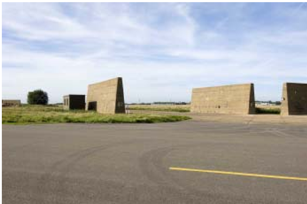
Figure 255 Late 1950s blast protection walls, eastern group walls 48 and 49 looking west. (c) English Heritage DP035649
