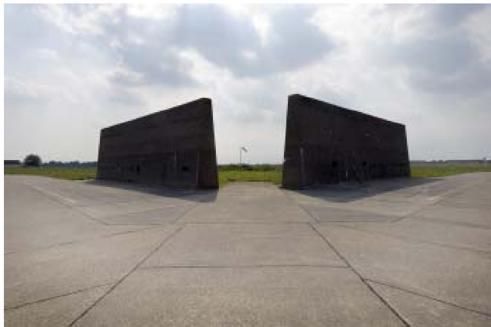
Figure 265 Late 1950s blast protection wall. (c) English Heritage DP027170
