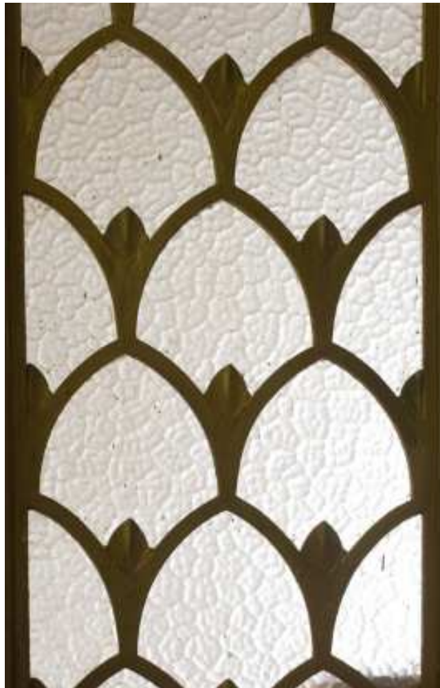
Figure 18 Station Headquarters, detail of window. (c) English Heritage DP027353
