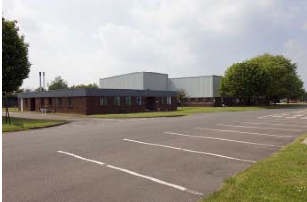
Figure 166 Building 349, Jaguar Flight Simulator operated by Thames Merlin Training Services, from south east. This building was specially constructed about 1975 to meet the training needs of the Jaguar pilots. (c) English Heritage DP027204
