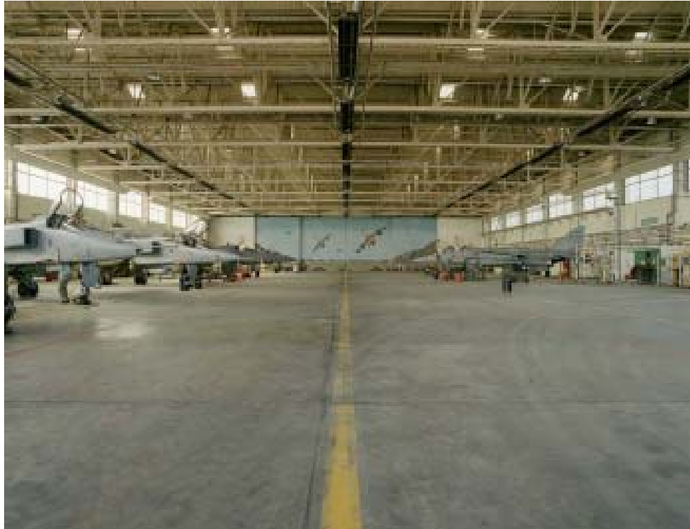
Figure 212 Hangar 1 interior looking towards the west doors. (c) English Heritage AA054404
