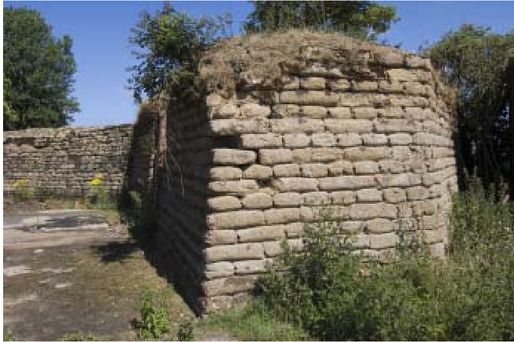
Figure 272 Second World War protected dispersal point to the south of Manor Farm, showing detail of cement sand bag construction technique (c) English Heritage DP027340
