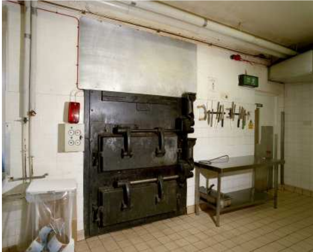
Figure 65 The Junior Ranks Mess, kitchen, west end, late 1930s Collins Cantilever Oven by Thomas Collins Co Ltd, Telephone Bristol 57061, it was originally coal fired oven. (c) English Heritage AA054452
