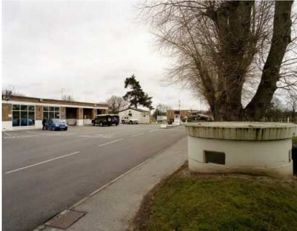
Figure 11 Main gate, showing the original guard room whose open veranda has been partly enclosed. To the right is a prefabricated Yarnold Shelter, these were constructed in the 1980s to guard against possible terrorist attack. (c) English Heritage AA054382
