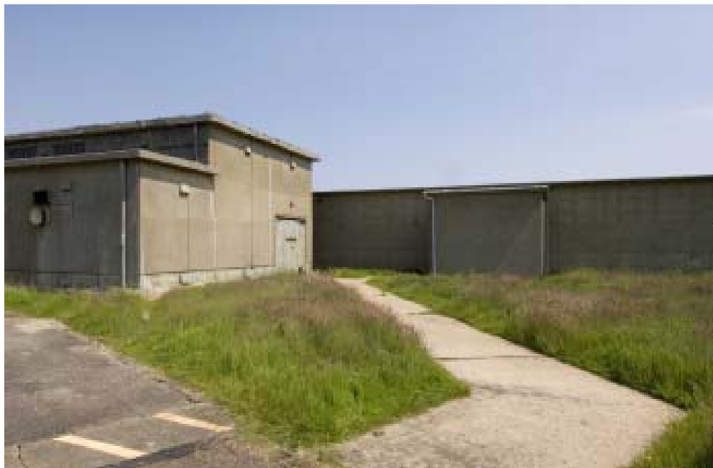
Figure 278 Missile and munitions storage area, 1950s missile inspection and preparation building, from south (c) English Heritage DP027185
