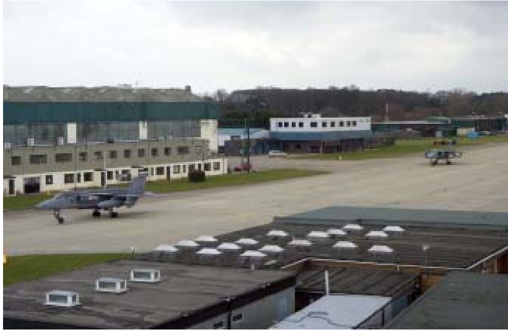
Figure 244 March 2006, view from Visual Control Room towards Hangar 1, Jaguar GR3A XX725, tailcode FE, on the taxiway in front of Hangar 1. (c) English Heritage DP029220
