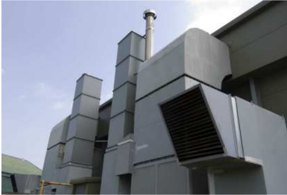
Figure 131 Jaguar Paint Facility, vents. (c) English Heritage DP027172
