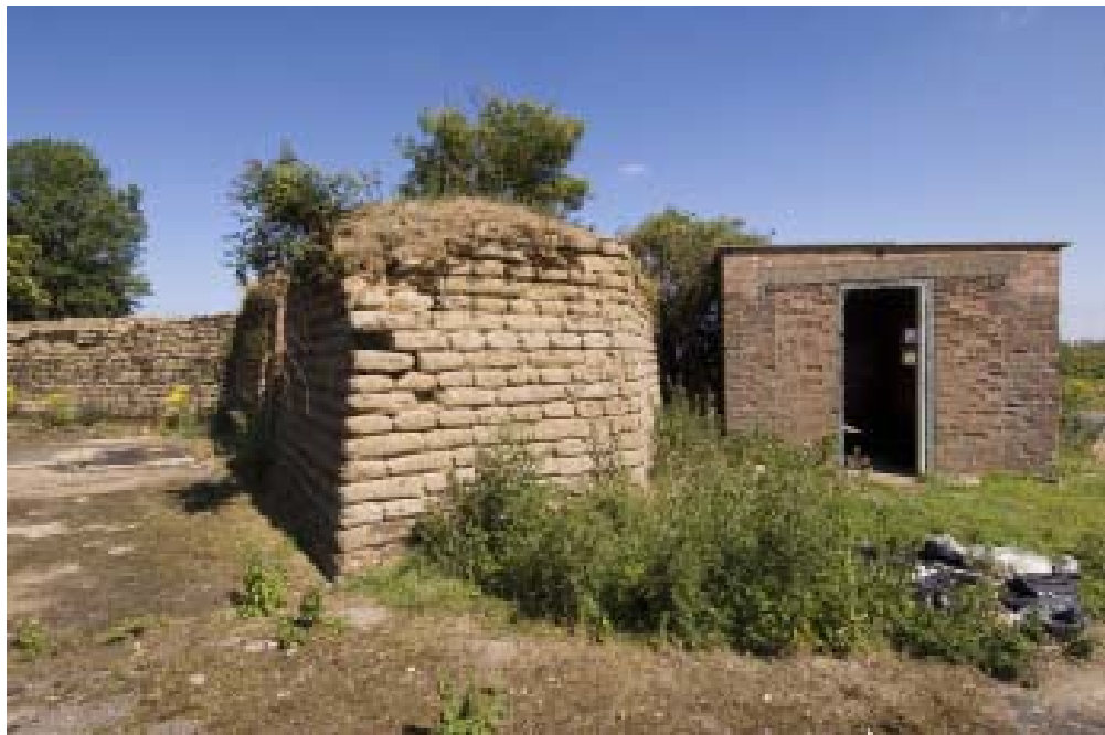
Figure 271 Second World War protected dispersal point to the south of Manor Farm, showing its cement sand bag walls and a small hut that perhaps originally housed an airfield tractor. The door opening has subsequently been reduced and a single door inserted. (c) English Heritage DP027341
