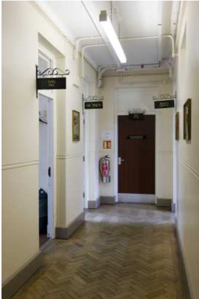
Figure 20 Station Headquarters, ground floor end of southwest corridor (c) English Heritage DP027348
