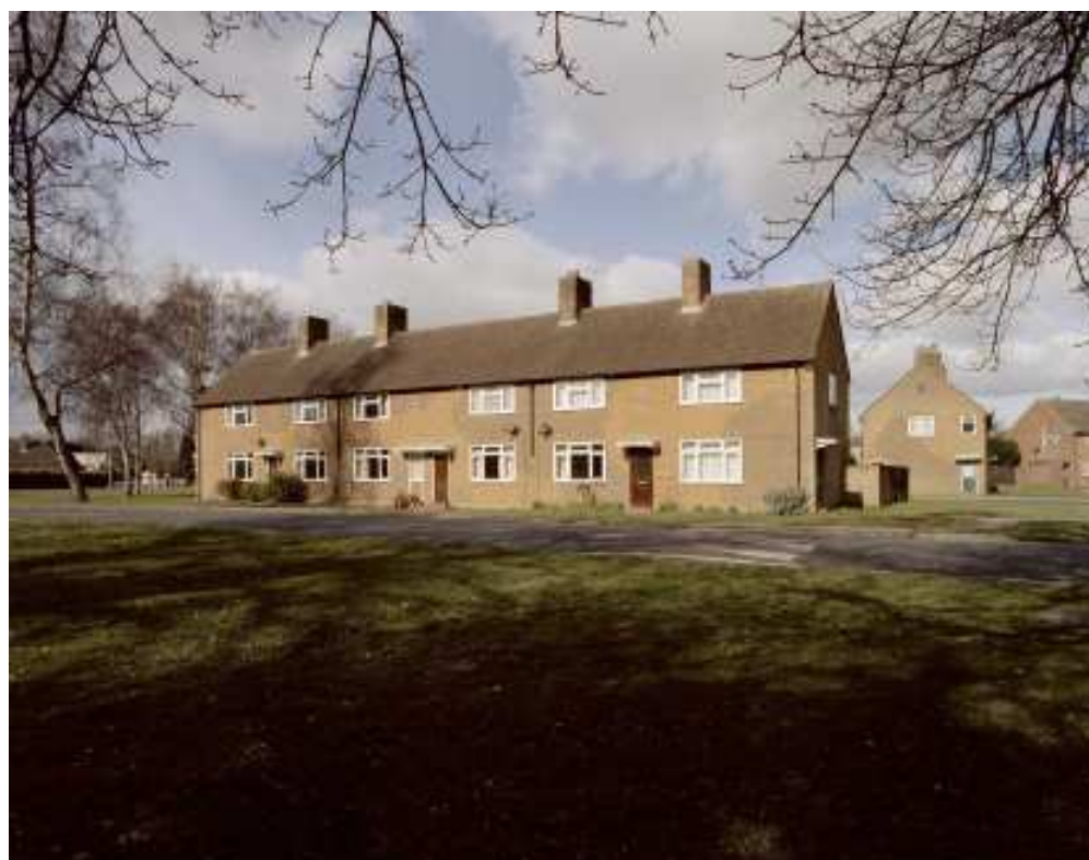
Figure 90 Cromes Place, 1930s Airmens' housing, south east corner of Ormesby Road. (c) English Heritage AA054362
