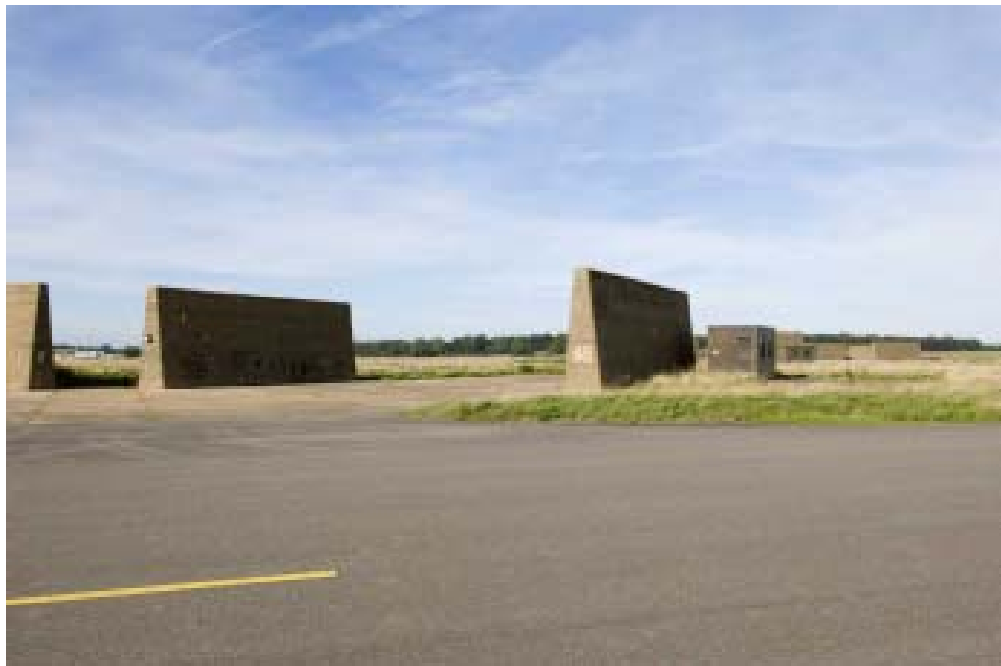
Figure 258 Late 1950s blast protection walls, eastern group wall 48 looking west (c) English Heritage DP035651
