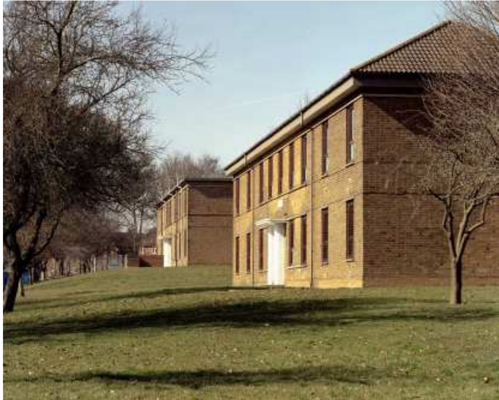
Figure 72 1930s barracks to the northeast of the parade ground, in the foreground Braham, Building 27B and to its rear 27A. These buildings originally had flat incendiary bomb proof roofs that have been replaced by later gable roofs. (c) English Heritage AA054446
