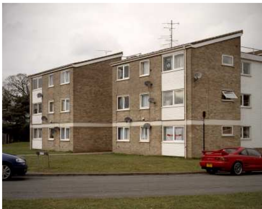
Figure 106 Post-war airmens' accommodation, 177-188 Ormesby Road. (c) English Heritage AA054368
