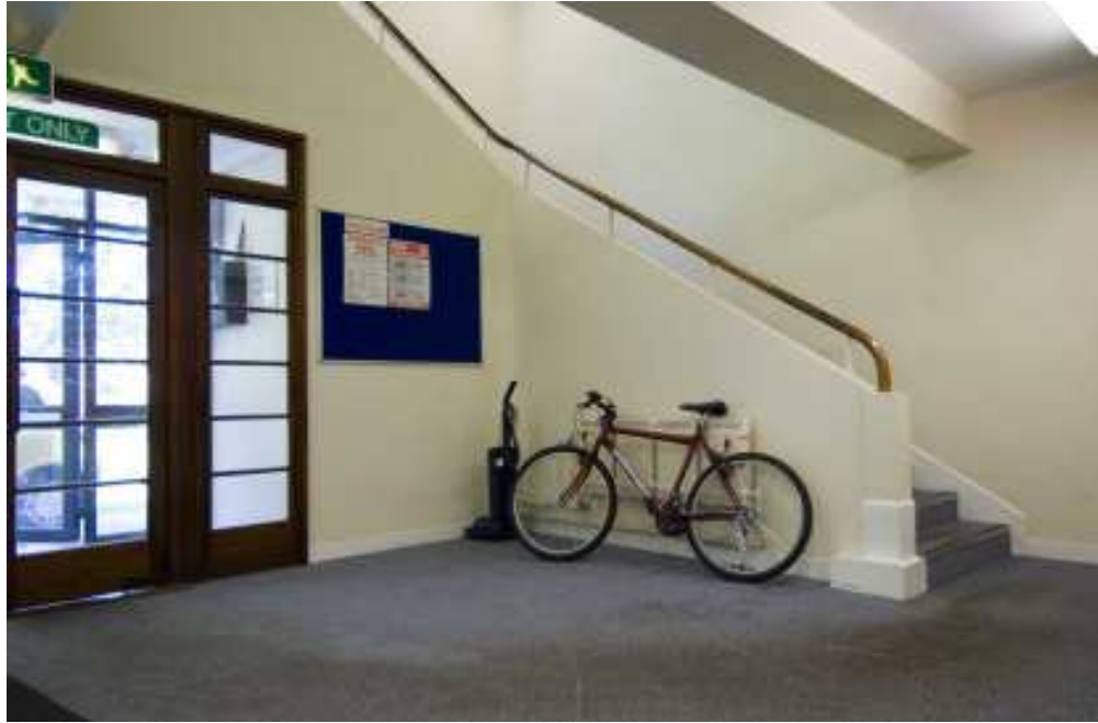
Figure 76 Hanbury block, main entrance. (c) English Heritage DP027330
