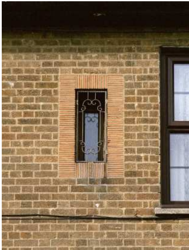
Figure 31 The officers' mess, architectural detail. (c) English Heritage AA054417
