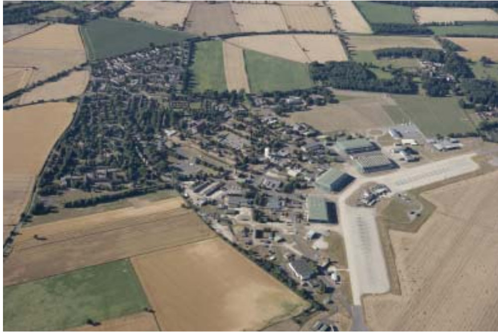
Figure 186 This view from the south shows the sweep of the hangars and to their right the 1950s aircraft servicing platforms. In the foreground is hangar 3 and above it hangars 2 and 1 with hangar 4 to the rear. In the original scheme it was intended to build another hangar to the right of hangar 3 but before completion it was destroyed German bombing. (c) English Heritage NMR 24369/017
