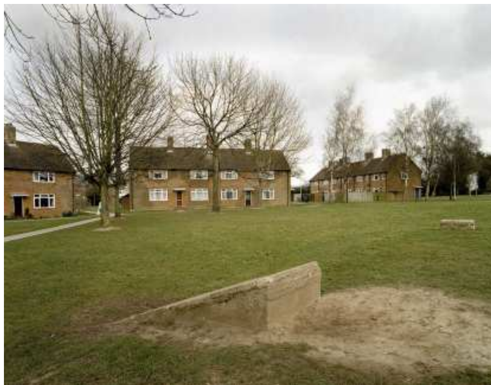
Figure 89 Cromes Place, 1930s Airmens' housing, in the foreground are the remains of a communal air raid shelter. (c) English Heritage AA054377
