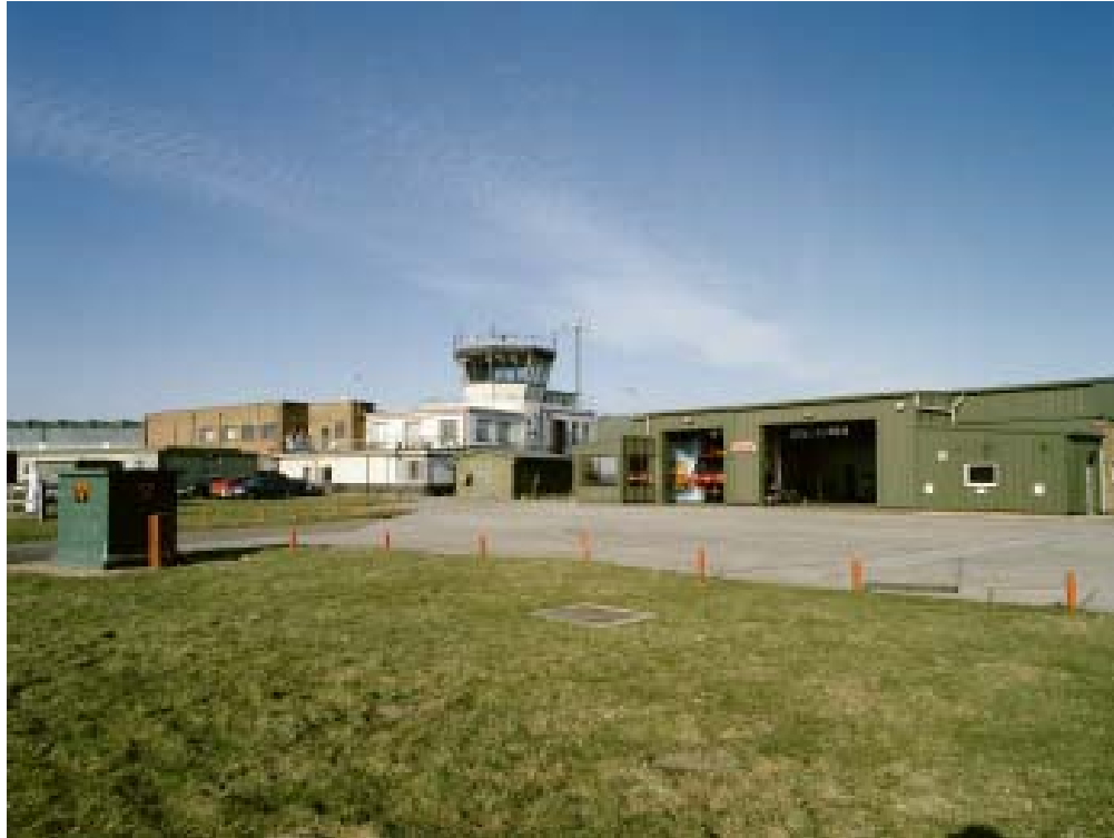
Figure 232 Watch Office and to its right the fire section (c) English Heritage AA054409
