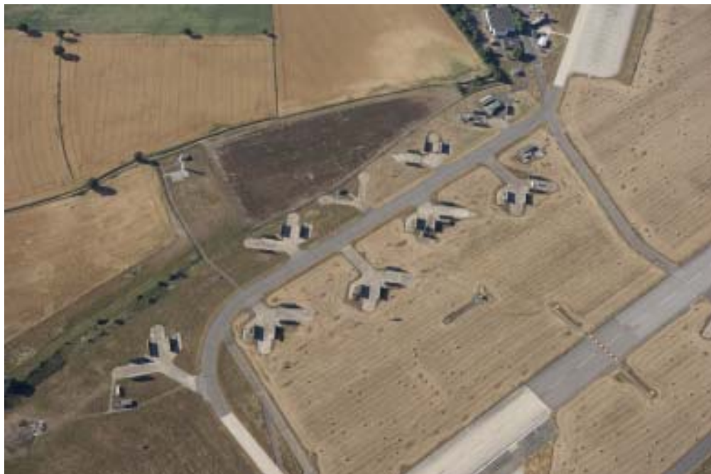
Figure 249 Group of 1950s blast protection wall in the south west corner of the airfield. The blast walls gave protection against low level attack for a squadron of aircraft. The black and yellow chequered line on the runway marks the position of the south west Rotary Hydraulic Arrestor Gear, between it and the blast walls are the remains of the Instrument Landing System. To the rear is the Watchman radar tower. (c) English Heritage NMR 24369/018
