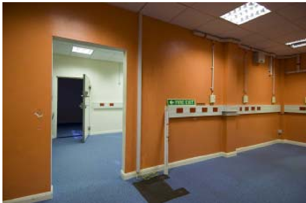
Figure 239 Watch Office, October 2006, stripped ground floor of the post-war extension that formerly housed communications and navigation equipment. (c) English Heritage DP035645
