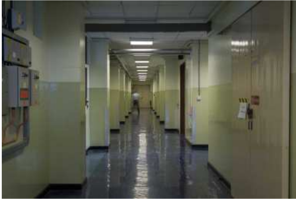
Figure 139 Building 295, Headquarters Electrical Engineering Squadron, internal corridor from south west (c) English Heritage DP029242.
