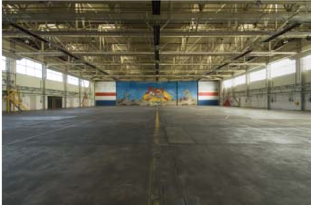
Figure 228 Hangar 1, October 2006, looking towards the east doors. (c) English Heritage DP035653
