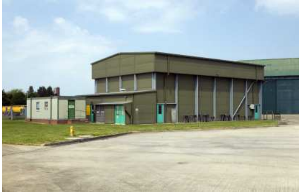
Figure 129 Building 378, Jaguar Paint Facility, this structure was purpose-built for spraying Jaguar aircraft . (c) English Heritage DP027167
