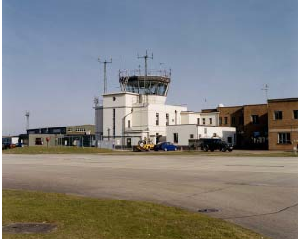
Figure 230 Watch Office, rear view from west showing the later 1950s extension to the right, with the meteorological briefing room on its upper floor. (c) English Heritage AA054461
