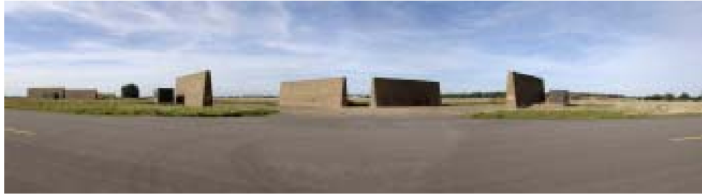
Figure 256 Late 1950s blast protection walls, eastern group 48 and 49 looking west. (c) English Heritage DP035672
