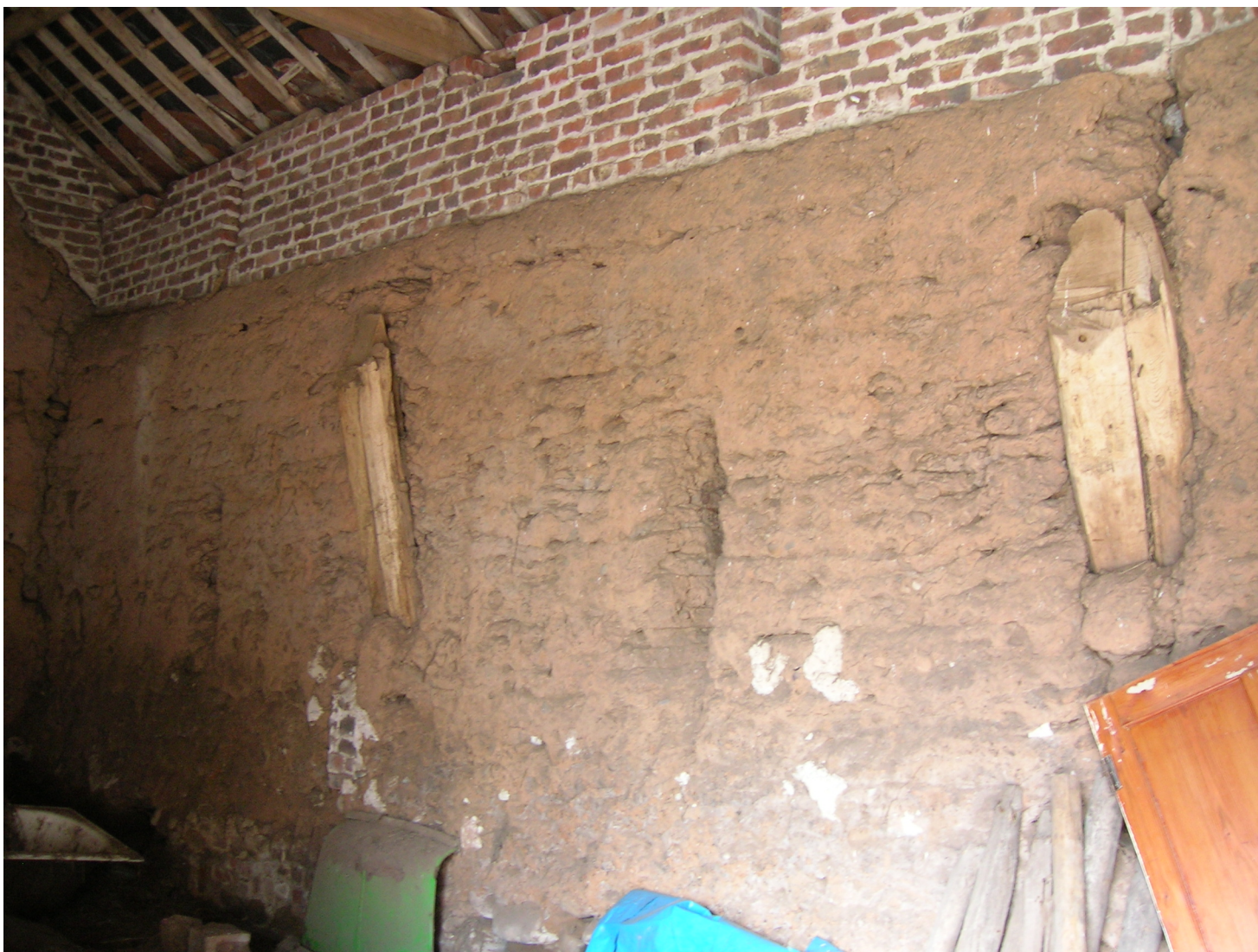
Figure 5: Truncated cruck blades F (left) and G, High Beeches and The Hollies, Thurstonfield, which were sampled for dendrochronology
