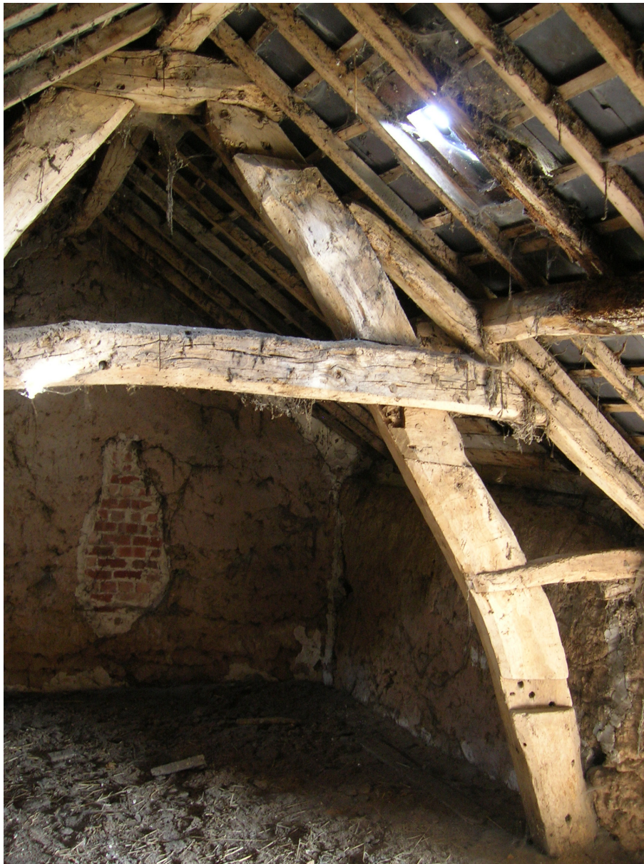
Figure 4: Cruck truss E-EI at High Beeches and The Hollies, Thurstonfield
