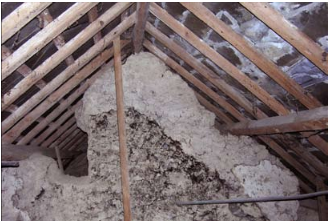
Fig. 15 The two-phase cob wall as viewed from the roof space above the hall, looking north. [DP047048]
