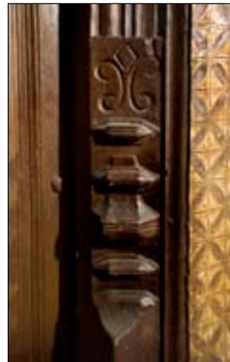
Fig. 31 Detail of stop, door in north wall of hall. [DP031557]
