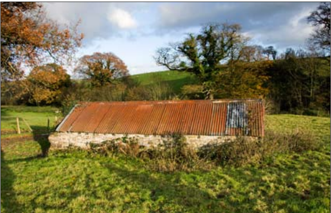
Fig. 74 The wheel house. [DP031649]
