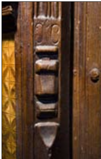
Fig. 30 Detail of stop, door in west wall of hall. [DP031549]
