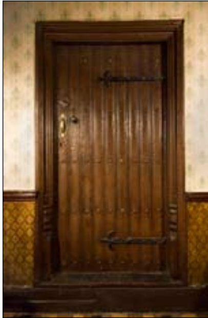
Fig. 28 The door in the west wall of the hall. [DP031548]
