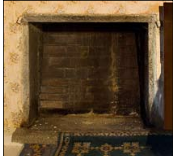
Fig. 17 Granite fireplace surround of the chamber above the old kitchen. [DP031622]
