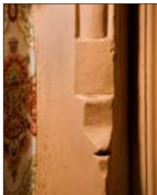
Fig. 26 Detail of stop, door of the chamber above the parlour. [DP031693]
