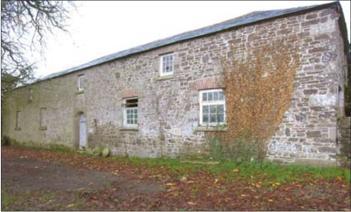
Fig. 69 The stable block, with the reset 'IBMB 1641' doorcase. [DP047065]
