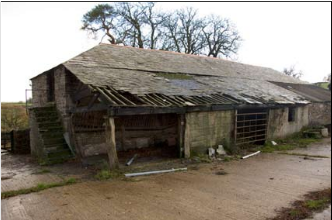
Fig. 70 The linhay portion of the stable block. [DP031665]
