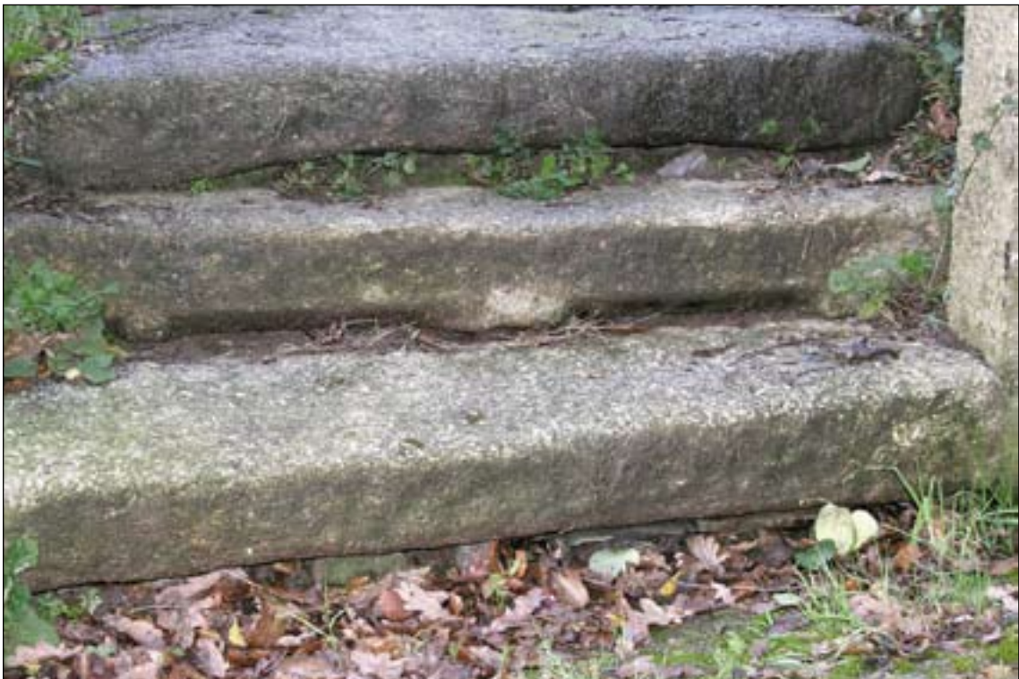
Fig. 18 Granite window lintels reused as steps west of the house, showing the nibs of some mullions. [DP047050]
