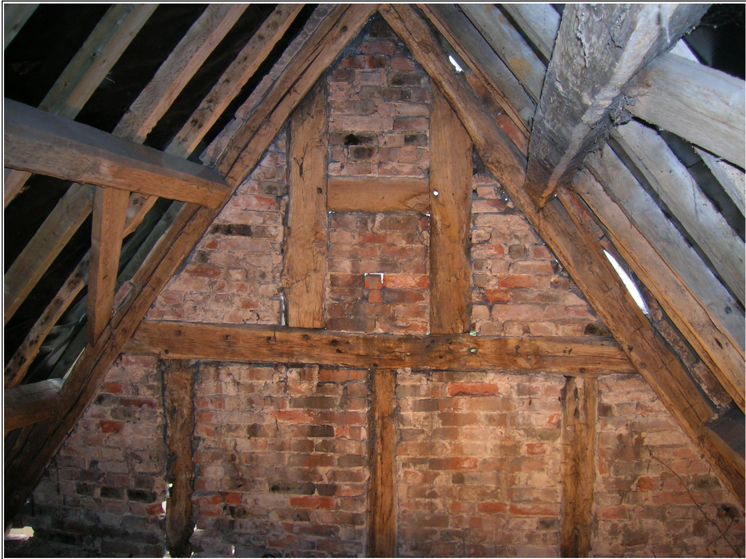
Figure 11: Timber-Framed Range, west gable
