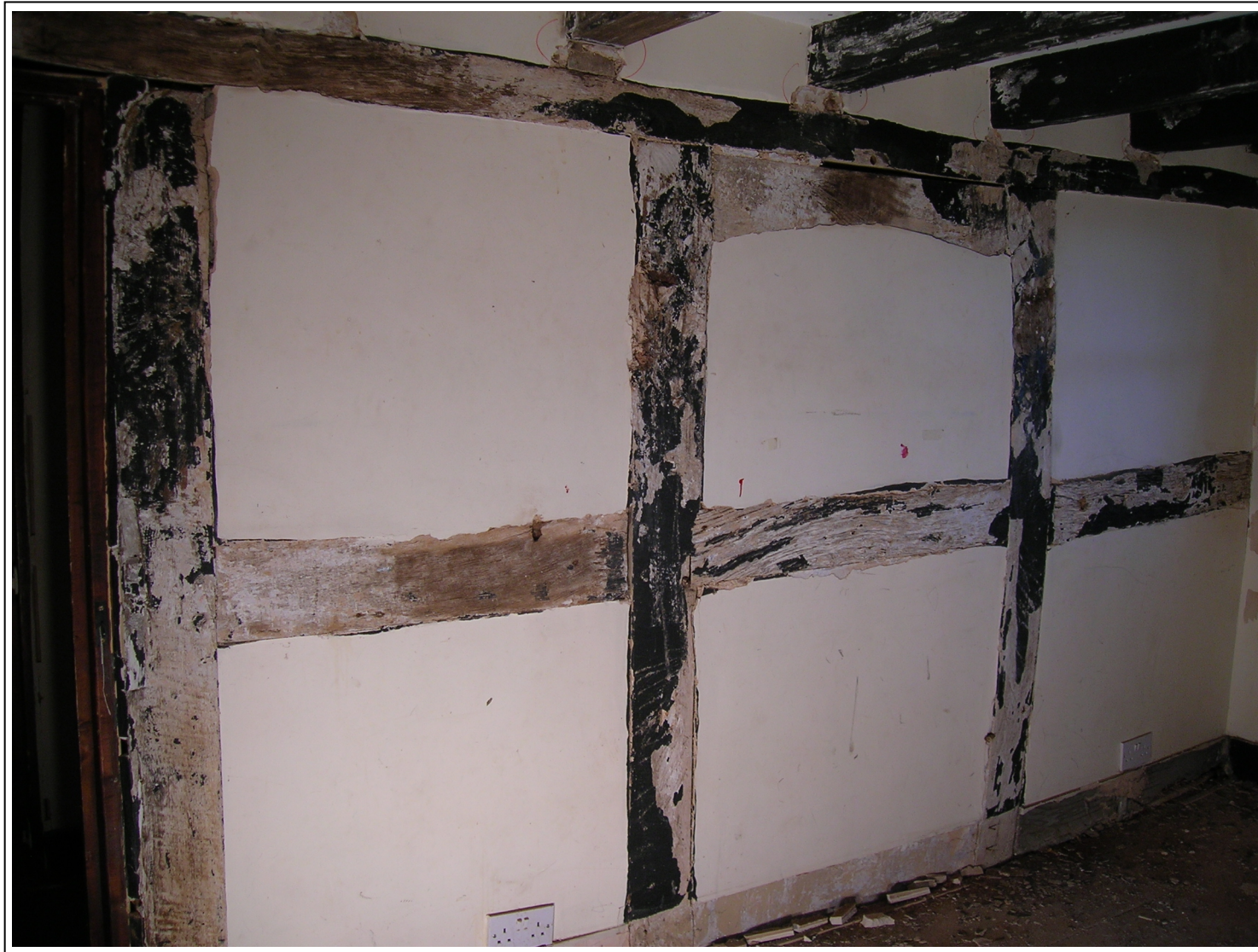
Figure 6: Stone Range, first-floor framing
