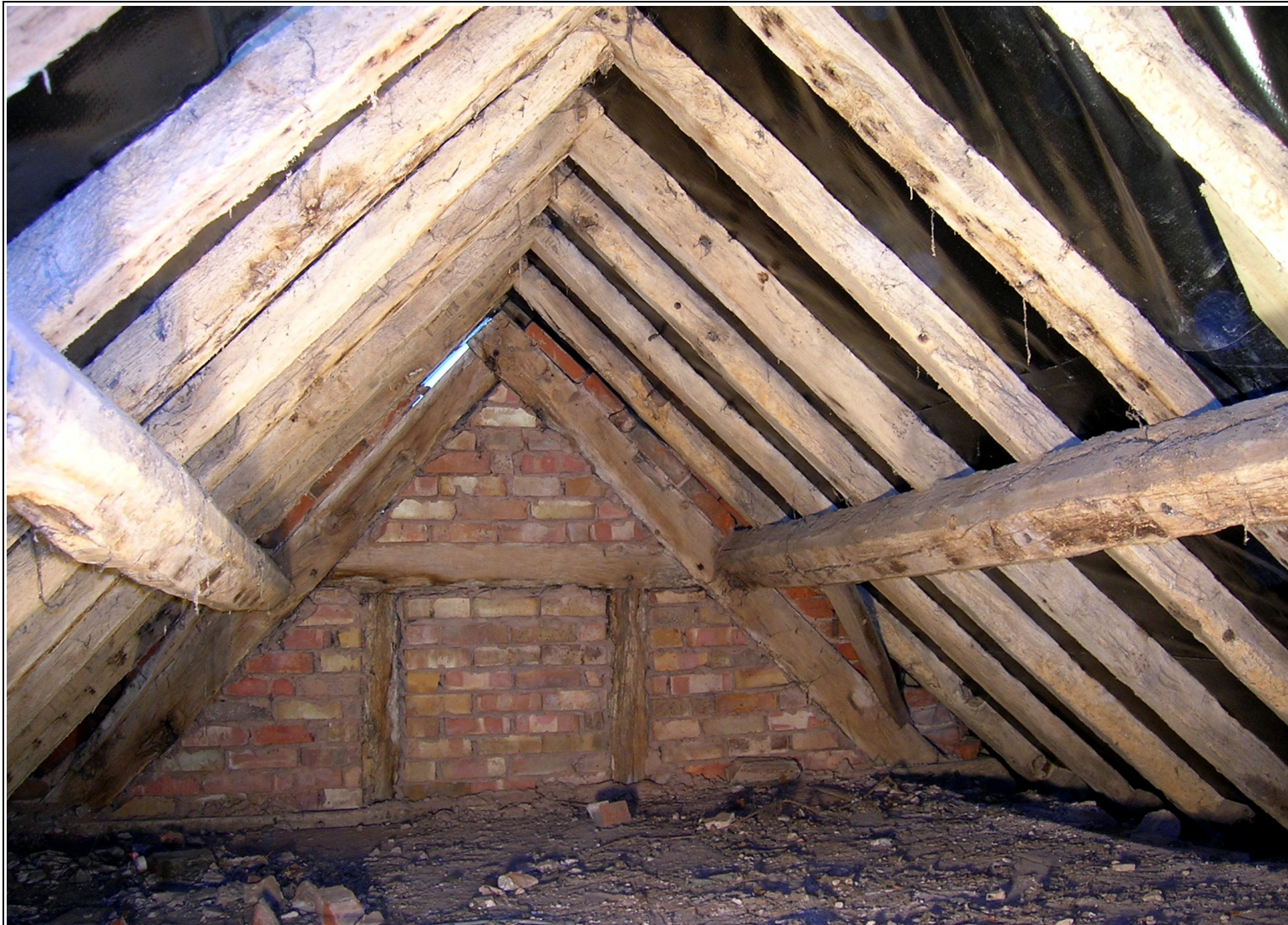
Figure 7: Stone Range, east roof, south gable truss
