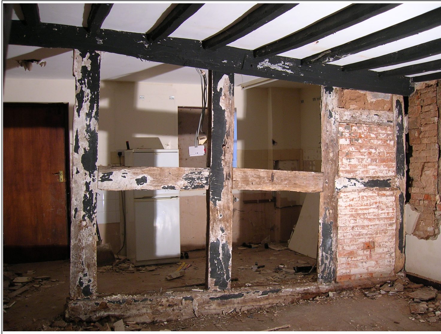
Figure 9: Timber-Framed Range, ground-floor framing
