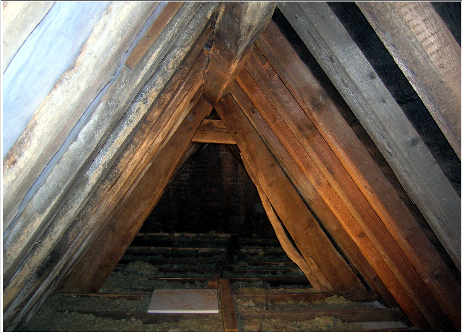
Figure 8: Stone Range, west roof (from the north)
