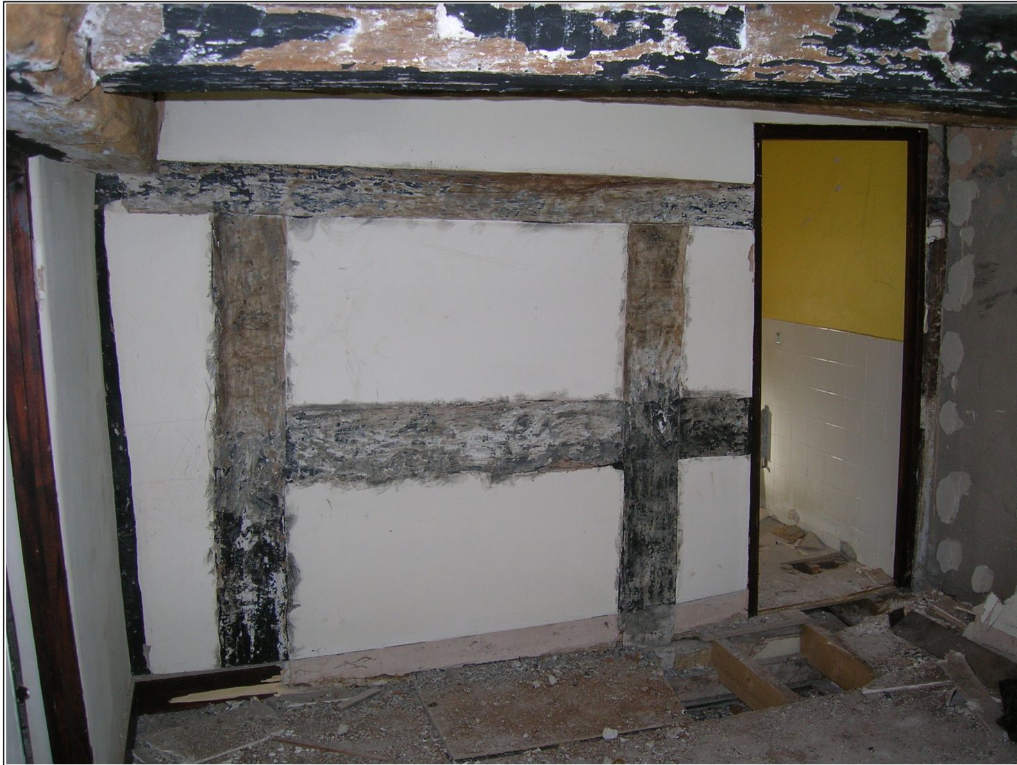
Figure 10: Timber-Framed Range, first-floor framing
