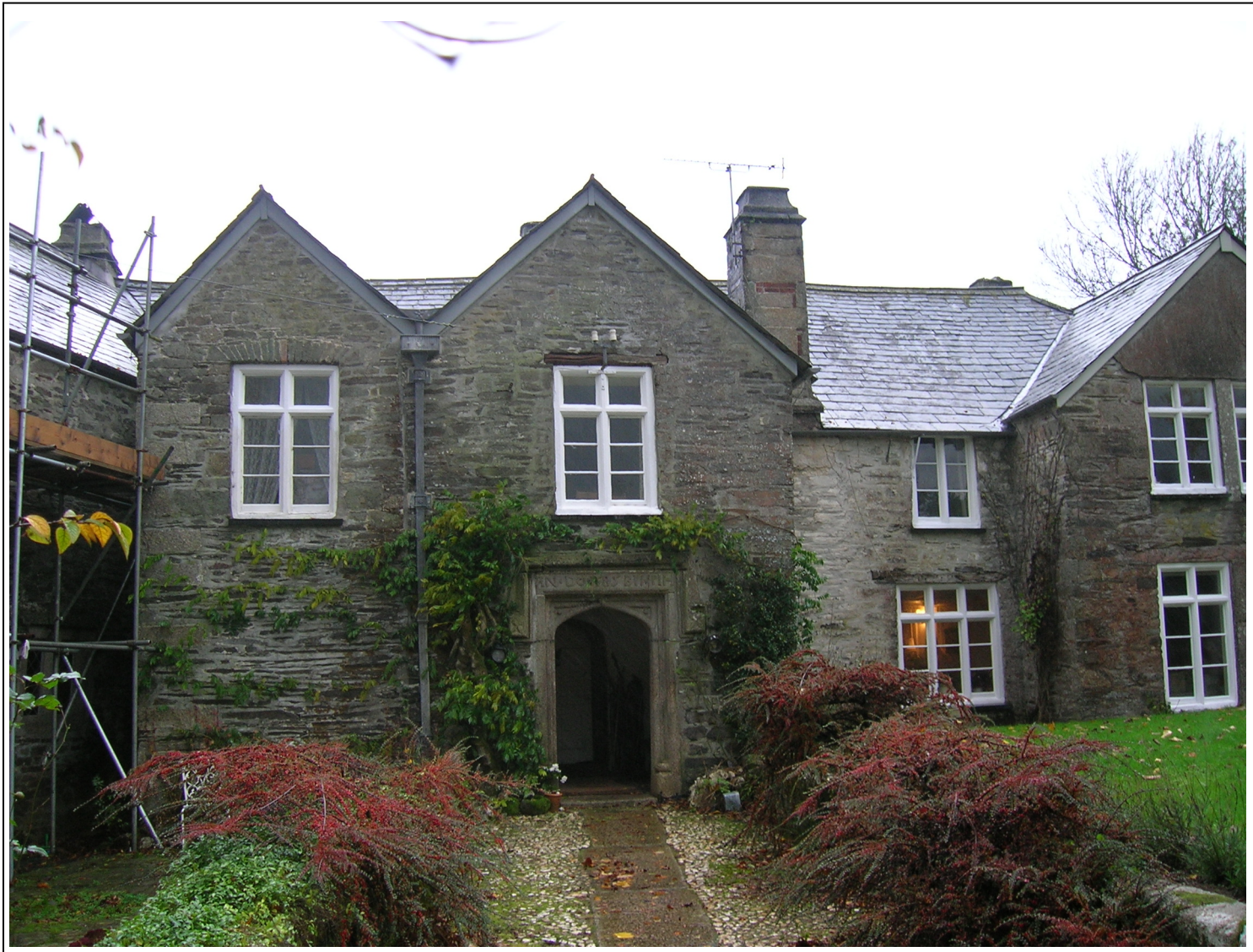
Figure 3: Hall range with porch addition
