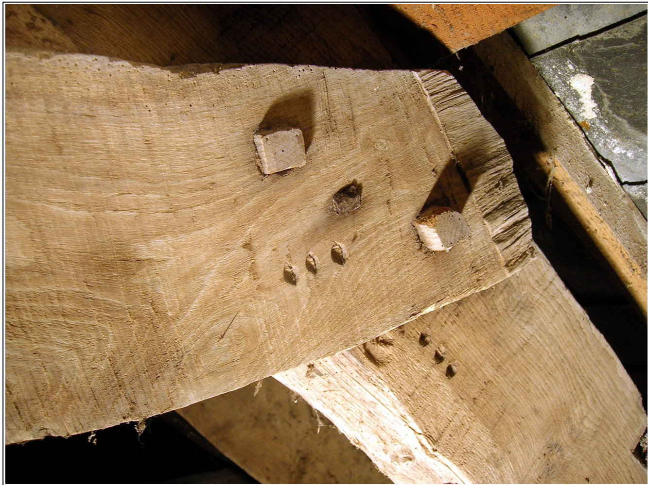
Figure 10: Trerithick House; West range, showing the 'dimple' carpenters mark (looking west)
