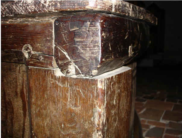
Figure 12: Detail of top left front joint of Cope Chest showing chamfer misaligning with corner post (D Miles)
