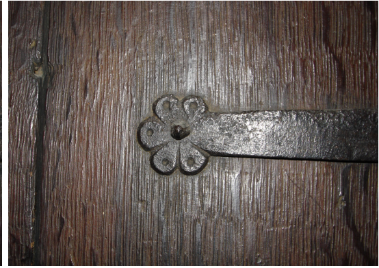
Figure 36: Termination of hinge to the Richard II Cupboard or Armoire, Muniment Room (D Miles)
