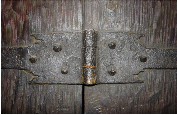
Figure 35: Knuckle of hinge to the Richard II Cupboard or Armoire, Muniment Room (D Miles)
