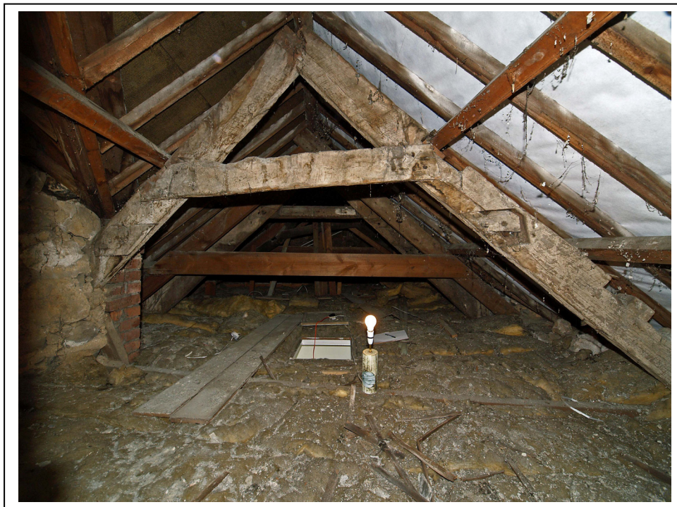
Figure 5a (top): Keigwin, roof over the rear range, showing smoke-blackened truss
