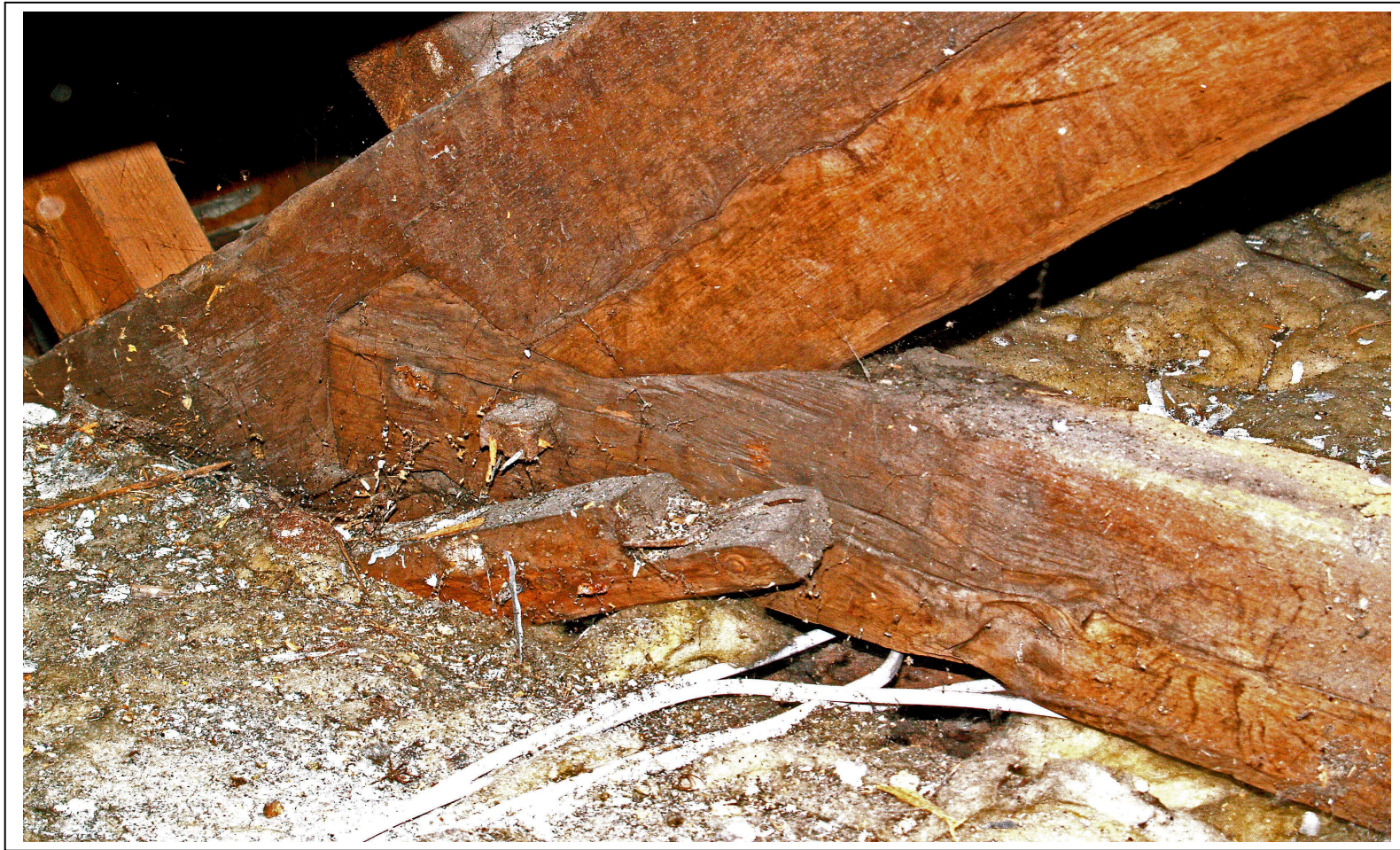
Figure 9: Little Keigwin (the upper chamber roof) showing the partially halved lap-dovetailed (or fishtail) collar joints (after Eric Berry and Nicholas Cahill)
