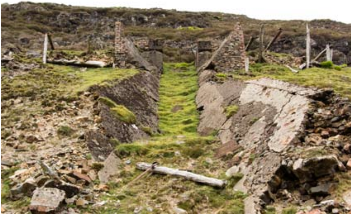
Figure 12. View from the south of the ore hopper and chute. © English Heritage 2007, NMR reference DP054892.
