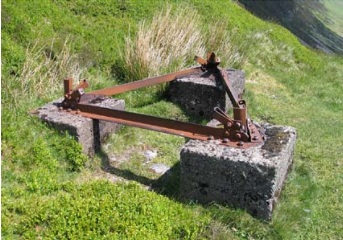
Figure 13. View of one of the aerial ropeway pylon bases. © English Heritage 2007.
