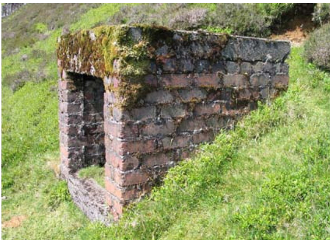
Figure 21. View from the east of the explosives store © English Heritage 2007
