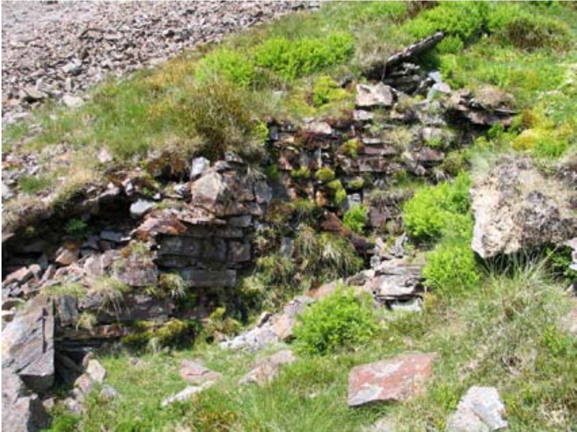
Figure 9. View from the south-east of the fragments of the possible early chute. © English Heritage 2007
