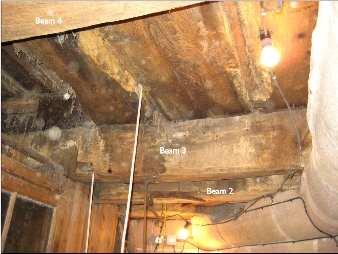
Figure 4: The underside of the belfry floor
