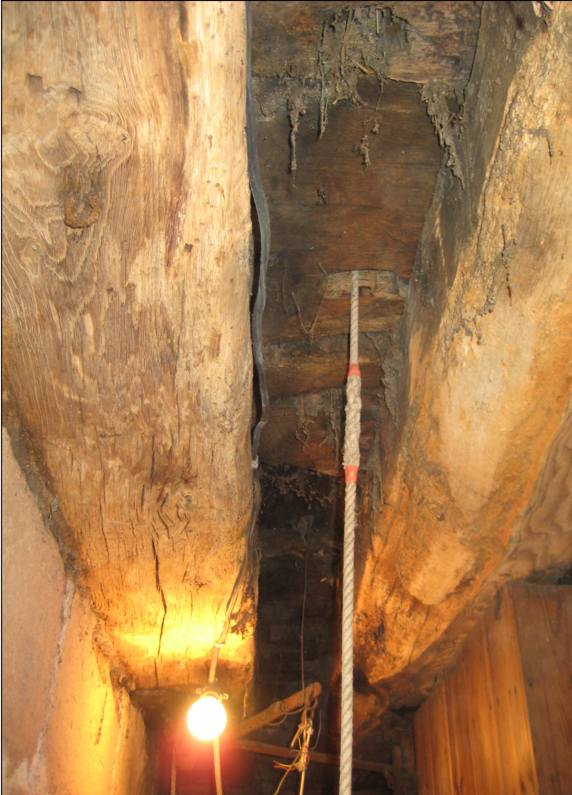
Figure 5: The underside of the belfry floor
