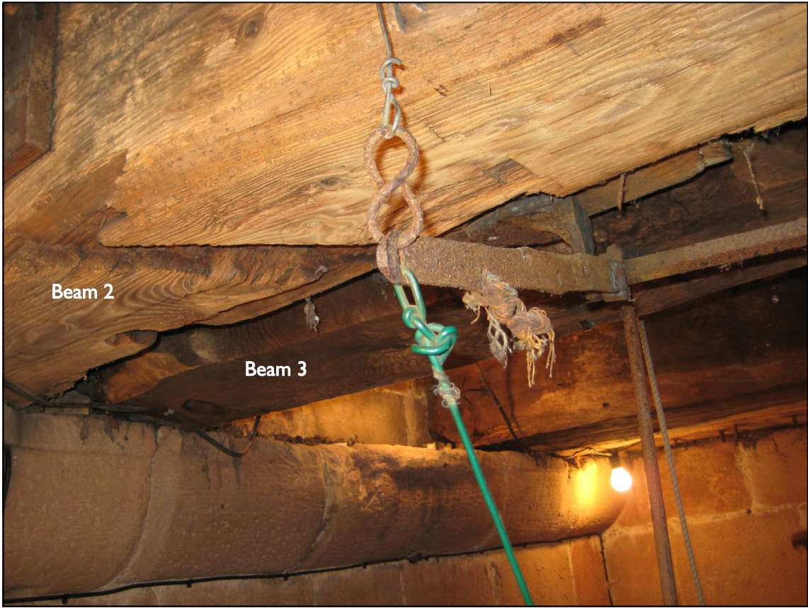
Figure 9: Beams 2 and 3 located immediately adjacent to each other
