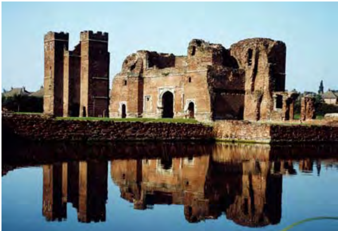
Figure 4: The unfinished remains of William, Lord Hastings' complete rebuild of the family seat at Kirby Muxloe.
