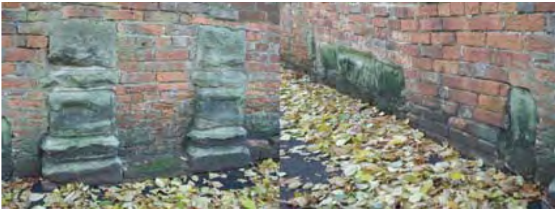
Figure 22: Masonry, probably reset, marking the possible position of gateways into the garden from Mount Walk.
