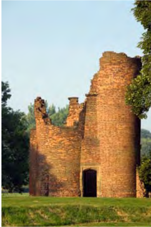
Figure 26: The western garden building.
