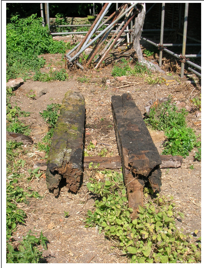
Figure 5: Photograph to show two of the removed bridging beams
