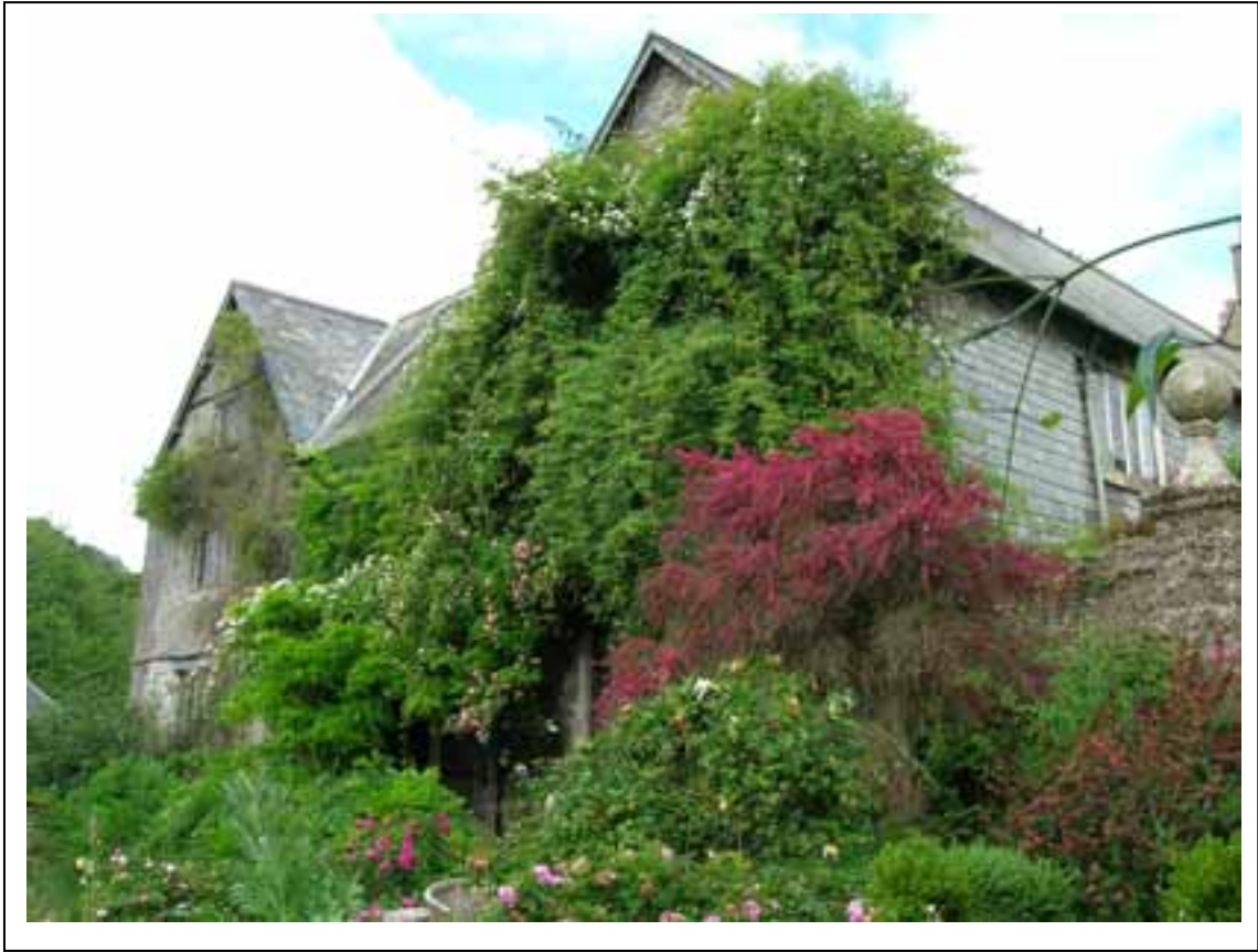
Figure 5: View of Pridhamsleigh Manor from the south west
