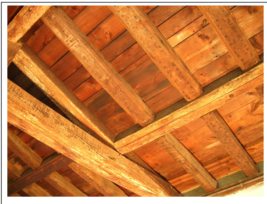
Figure 5a (top): View of the moulded tiebeam of truss 3, the moulded upper south common rafters in bay 3 and the plain common rafters.
