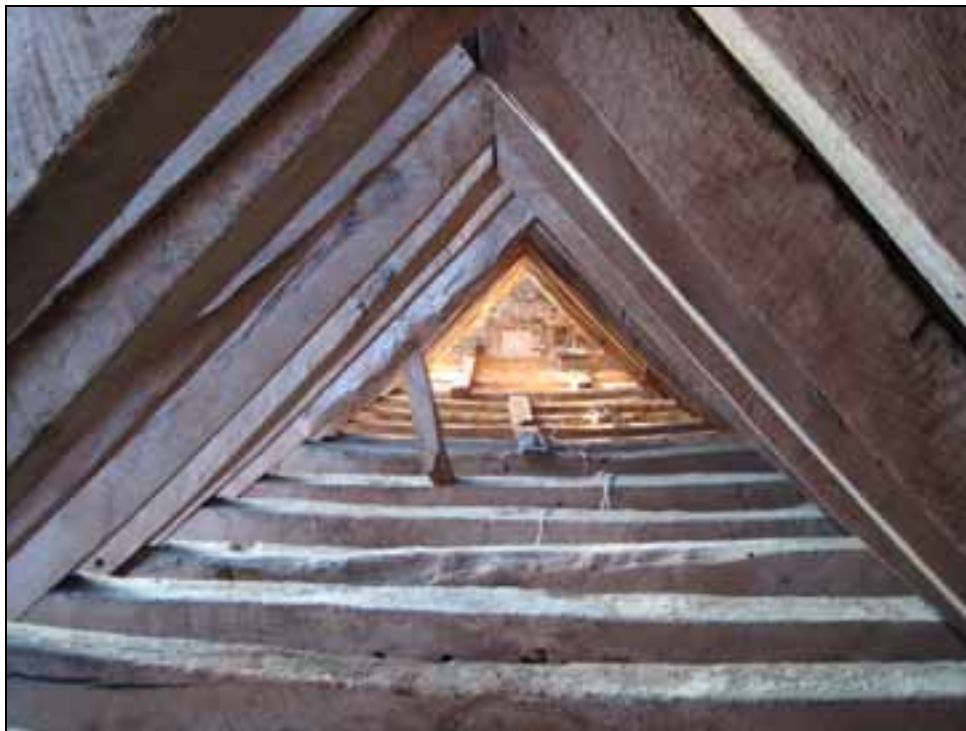
Figure 4: St Andrews Church, Nave roof, looking west
