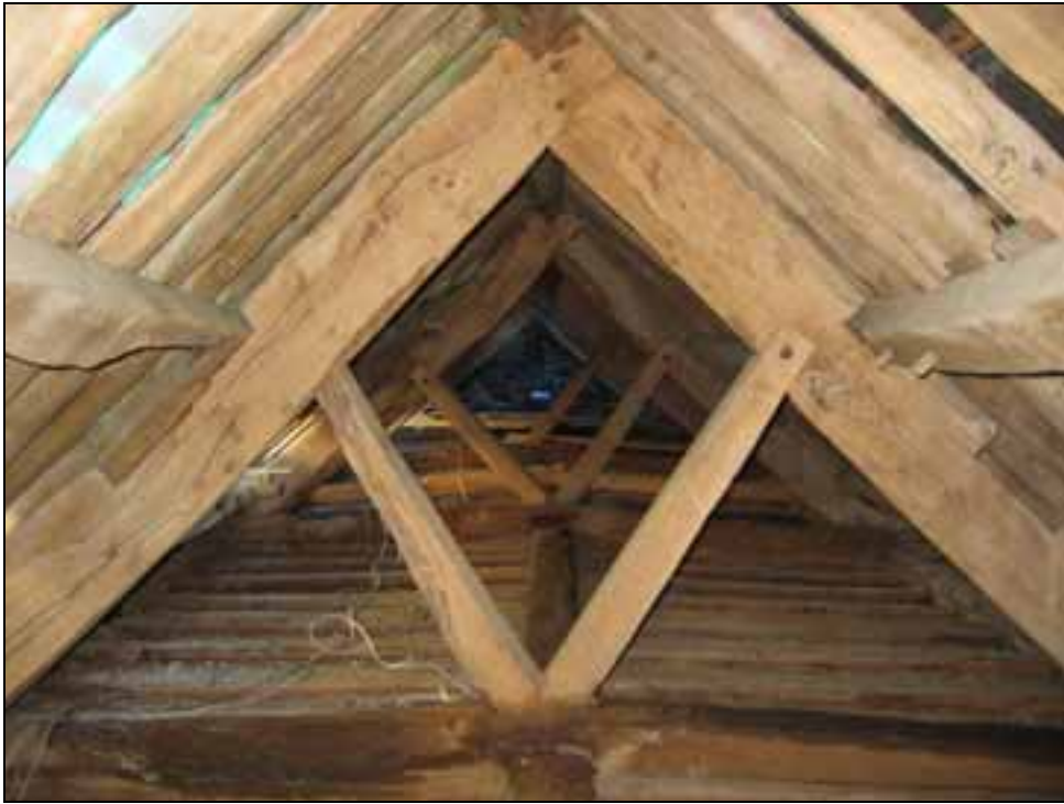
Figure 3: St Andrew's Church, South Aisle roof, Truss 6 in foreground
