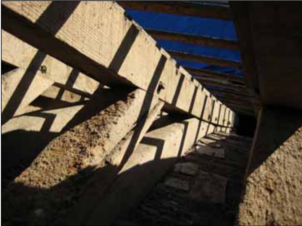
Figure 5: St Andrew's Church, Nave roof
